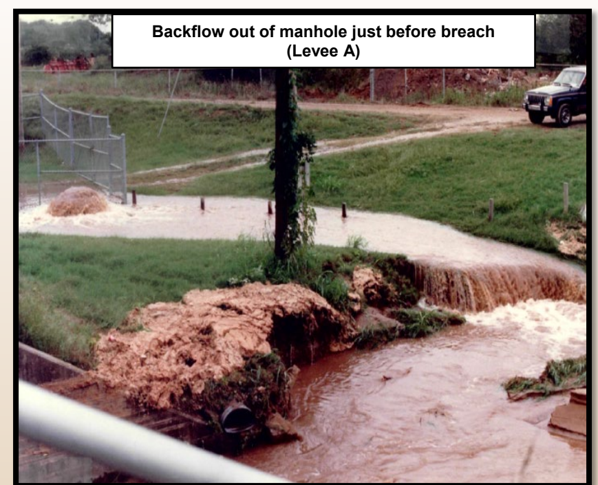
Partial Breach at Pump Station 1 (Levee A)
