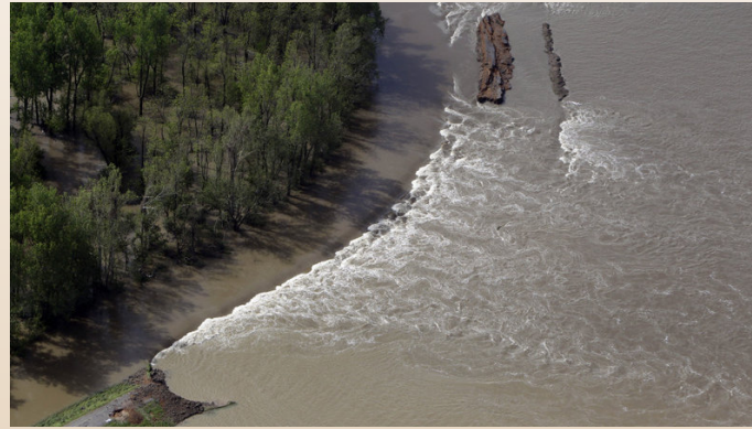
Floodway Operation Mississippi River May 2011
