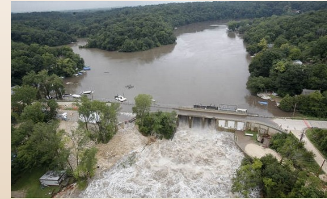
Dam Overtopping Iowa July 2010
