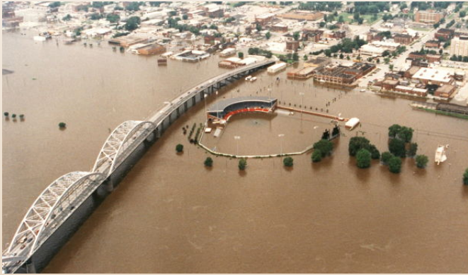
Levee Overtopping Mississippi River July 1993
