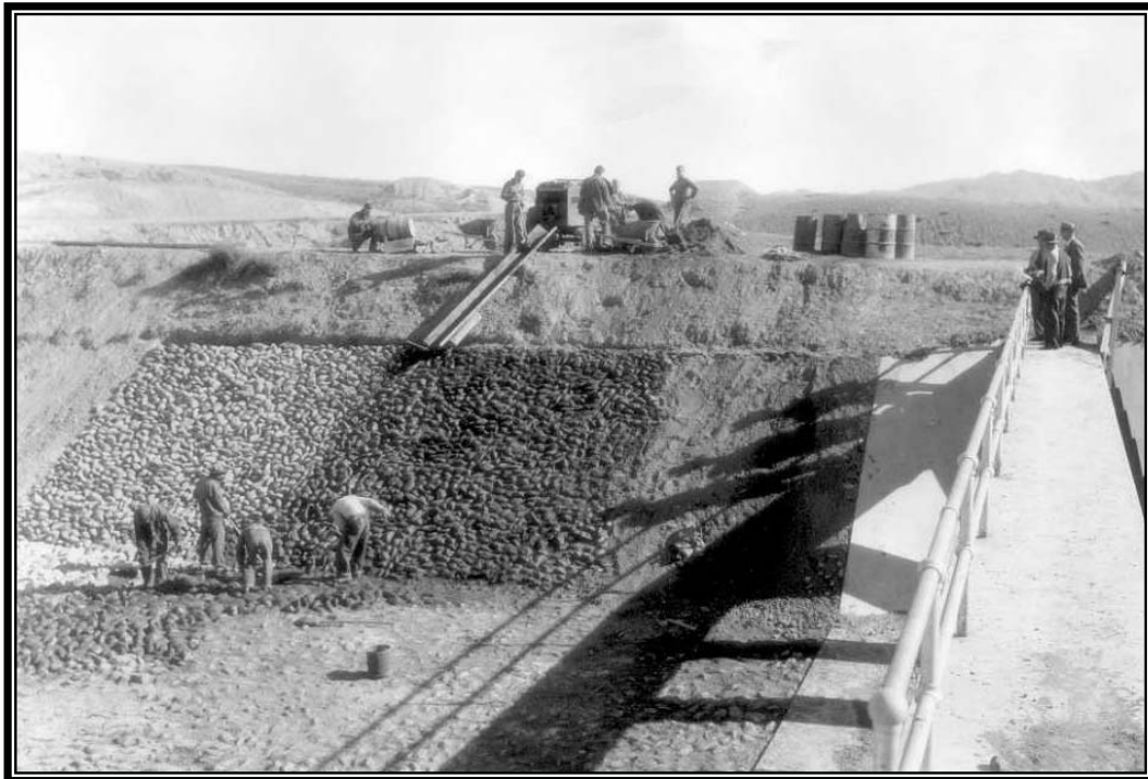
Camp BR-87: Shoshone Project, grouting and paving check in Heart Mountain Canal, October 9, 1941 (courtesy of Shoshone Irrigation District).
