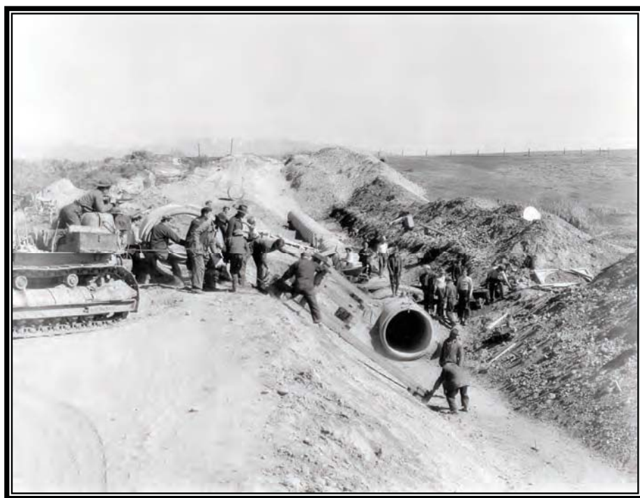
Camp BR-73: Boise Project, enrollees replacing old Ten Mile Flume with new concrete pipe siphon, March 13, 1941 (Box 2, Entry 31, RG 115, National Archives, Denver).
