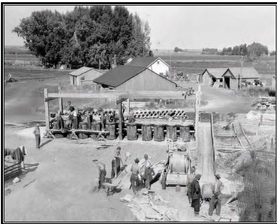
Camp BR-24; Boise Project, concrete pipe manufacturing plant built and operated by Camp BR-24, 1939 (Box 39, Entry 10, RG 115, National Archives, Denver).
