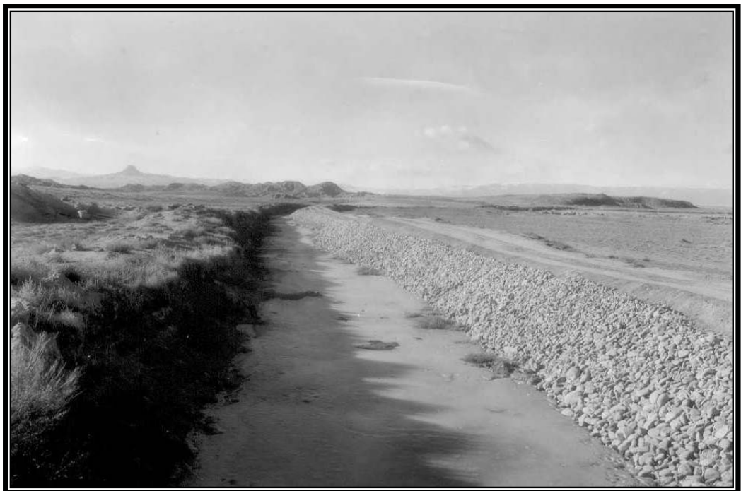
Camp BR-72: Shoshone Project, same section of Willwood Canal after being sloped and riprapped by CCC, January 14, 1939 (courtesy of Shoshone Irrigation District).
