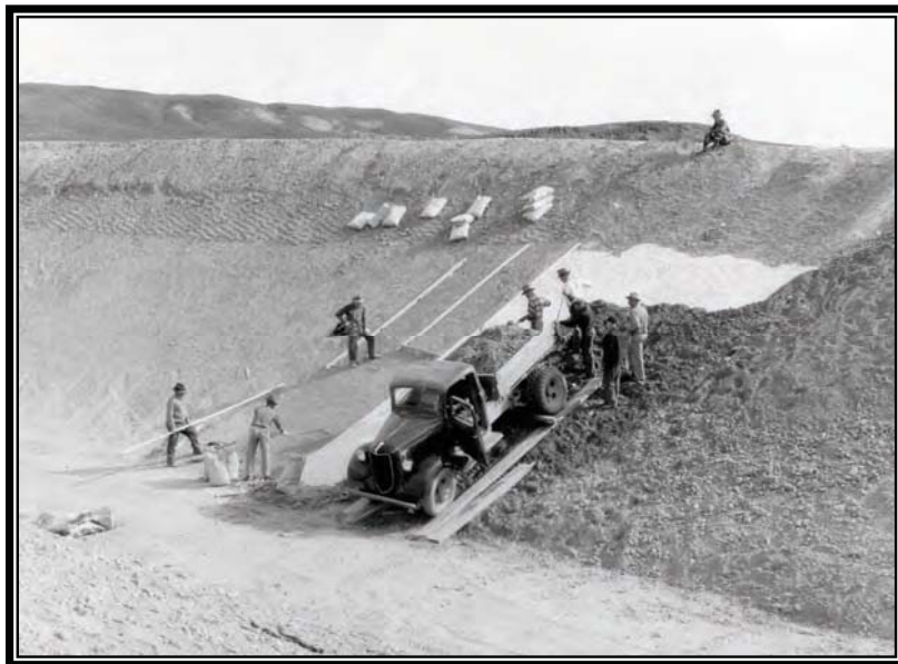
Camp BR-43: Owyhee Project, an 11-inch gravel blanket is placed on the layer of bentonite, March 18, 1941 (Box 1, Entry 31, RG 115, National Archives, Denver).
