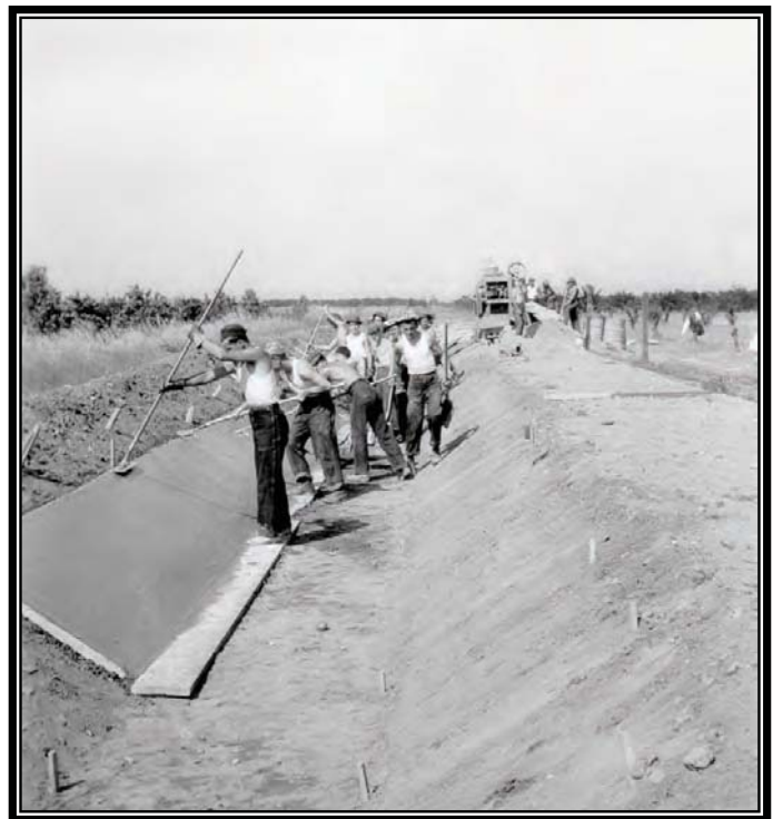
Camp BR-78: Orland Project, concrete lining operations on Lateral 50, date unknown (Box 2, Entry 31, RG 115, National Archives, Denver).
