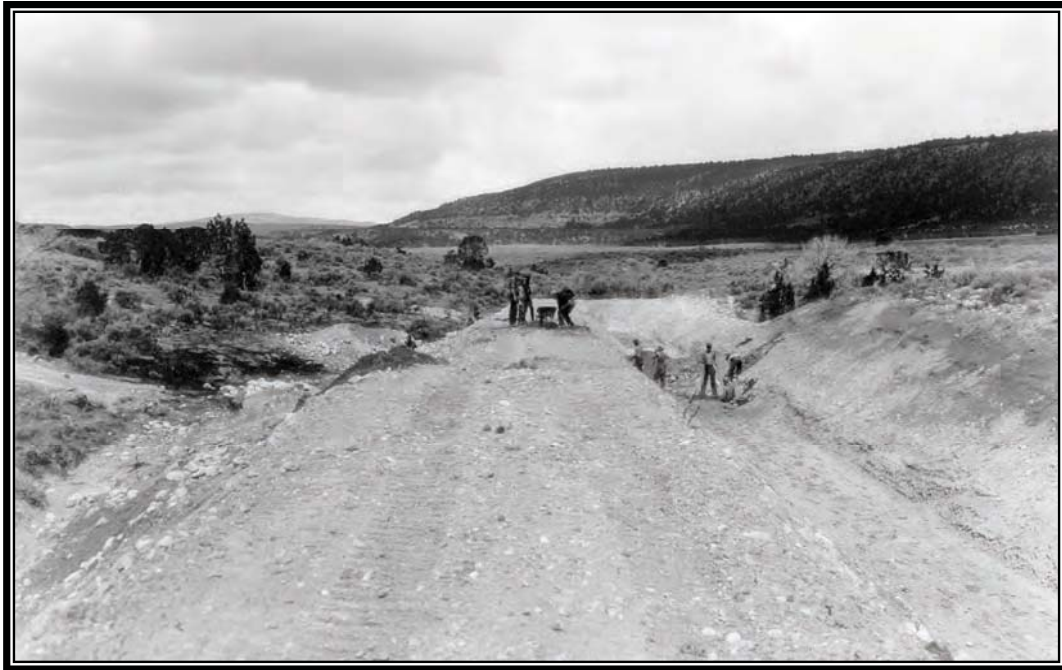
Camp BR-91: Provo River Project, enrollees excavating for diversion works of Cottonwood Wash, Yellowstone Feeder Canal, April 24, 1940 (Box 1, Entry 31, RG 115, National Archives, Denver).
