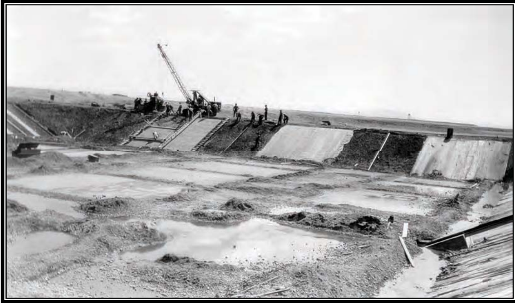
Camp BR-64: Provo River Project, concrete lining on equalizing reservoir No. 25 at the head of No. 25 Lateral System, South Ogden Distribution System on the Ogden River Project, June 26, 1941 (Box 1, Entry 31, RG 115, National Archives, Denver).
