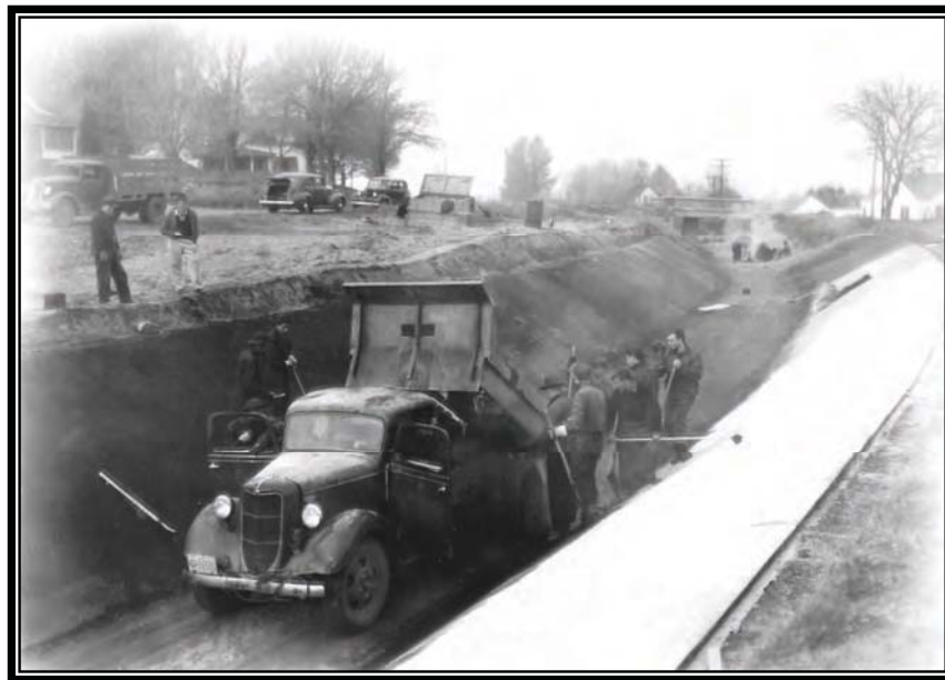
Camp BR-58: Yakima Project, asphaltic concrete lining experimental project, Snipes Mountain Canal, mile 6.21, showing placing of material, November 13, 1939 (Box 1, Entry 31, RG 115, National Archives, Denver).
