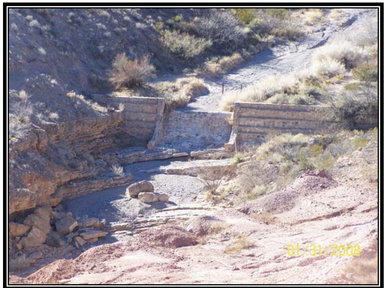
Camp BR-39: Rio Grande Project, view of CCC-constructed check dam in 2008 (courtesy of Dan Carter, Bureau of Land Management).
