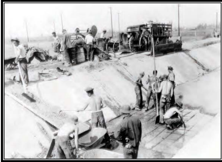
Camp BR-86: Yakima Project, Snipes Mountain Canal lining, placing concrete at about station 165+00, looking northwest from East Canal bank, March 22, 1940 (Box 21, 8NS-115-95-112, RG115, National Archives, Denver).
