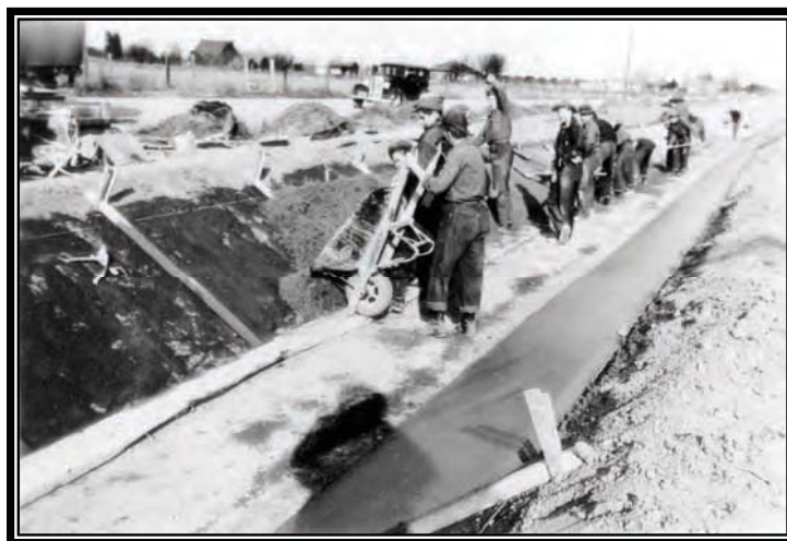
Camp BR-78: Orland Project, concrete lining operations on Lateral 232, date unknown (Box 2, Entry 31, RG 115, National Archives, Denver).
