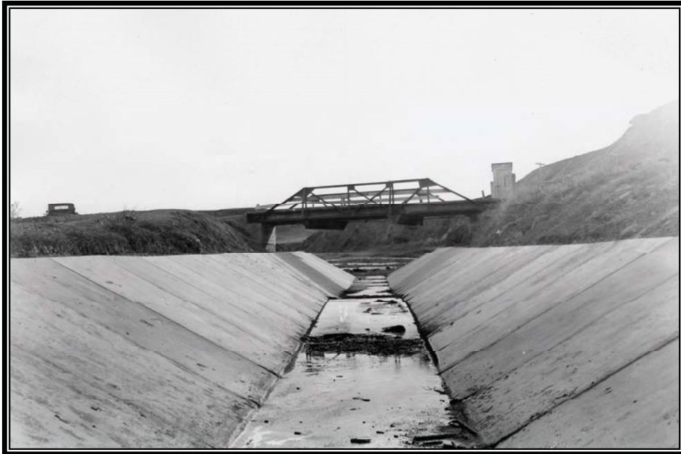
Camp BR-69: Milk River Project, concrete lining at Rocky Point looking downstream, December 6, 1939 (Box 1, Entry 31, RG 115, National Archives, Denver).
