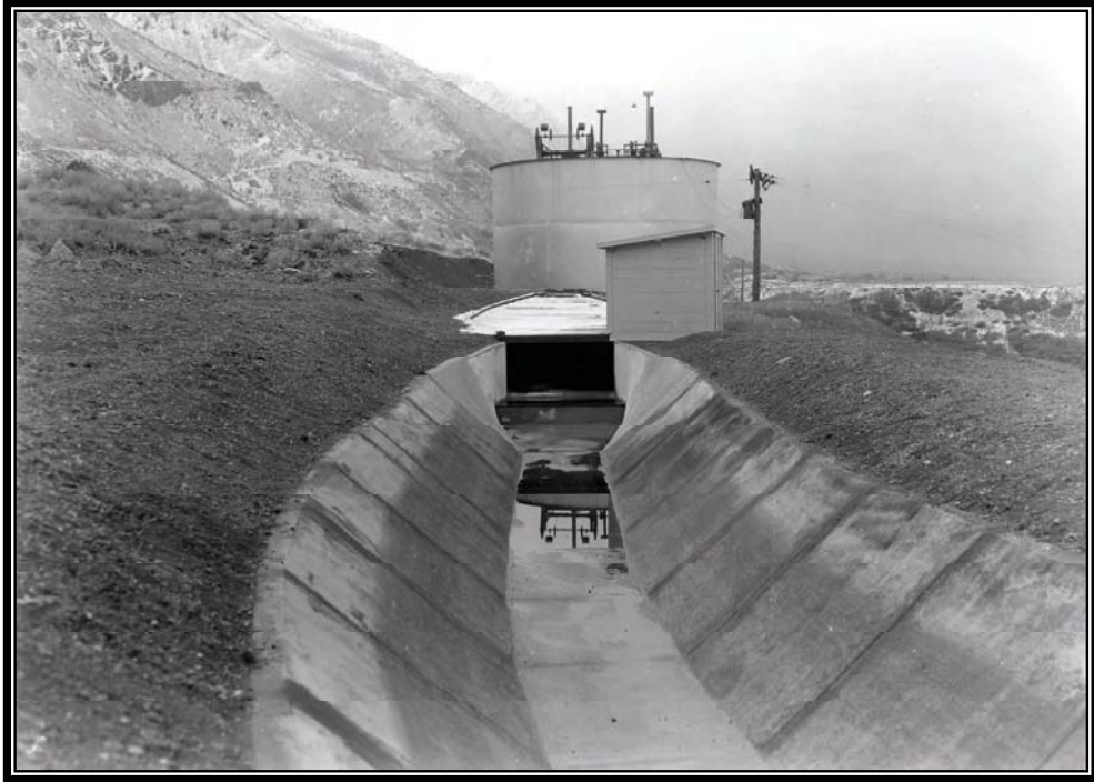
Camp BR-64: Provo River Project, upstream view of completed Venturi flume at station 0+30, Ogden-Brigham Canal, January 4, 1940 (Box 1, Entry 31, RG 115, National Archives, Denver).
