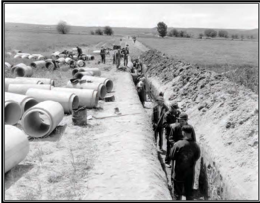
Camp BR-42: Owyhee Project, crew laying pipe siphon in Mitchell Butte Division, May 15, 1940 (Box 1, Entry 31, RG 115, National Archives, Denver).
