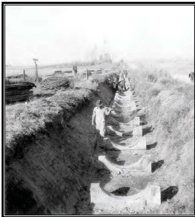
Camp BR-86: Yakima Project, replacement of 46-inch wood stave discharge pipe - Outlook Irrigation District. Shaping trench preparatory to laying new pipe, showing original pedestals on which new line will be erected, November 1939 (Box 2, Entry 31, RG 115, File 1, Photo No. 5).
