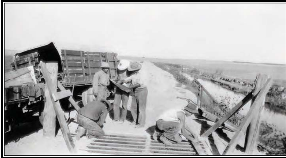
Camp BR-83: North Platte Project, cattle guard nearing completion, September 4, 1939 (Box 2, Entry 31, RG 115, National Archives, Denver).
