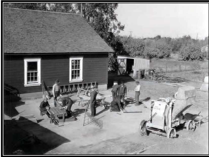
Camp BR-78: Orland Project, enrollees constructing concrete form work, date unknown (Box 2, Entry 31, RG 115, National Archives, Denver).
