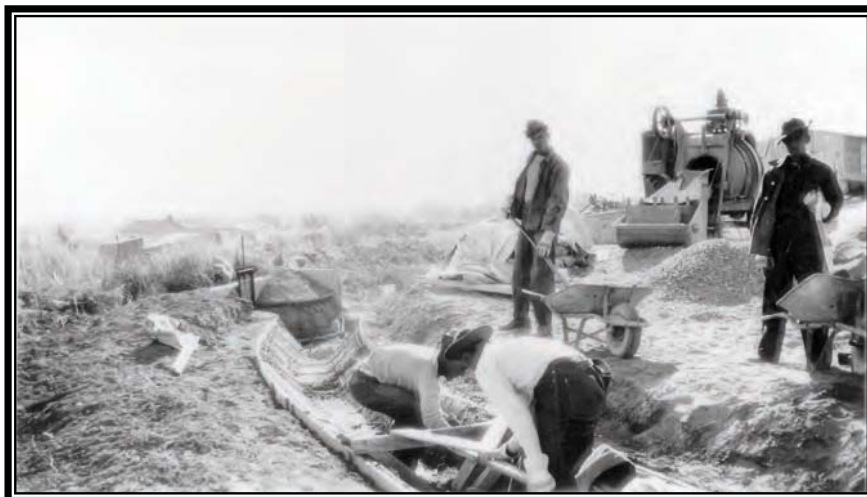
Camp BR-83: North Platte Project, concrete lining: backfilling and placing forms on section of Gantz Lateral, off Springer Main Lateral, September 24, 1940 (Box 2, Entry 31, RG 115, National Archives, Denver).
