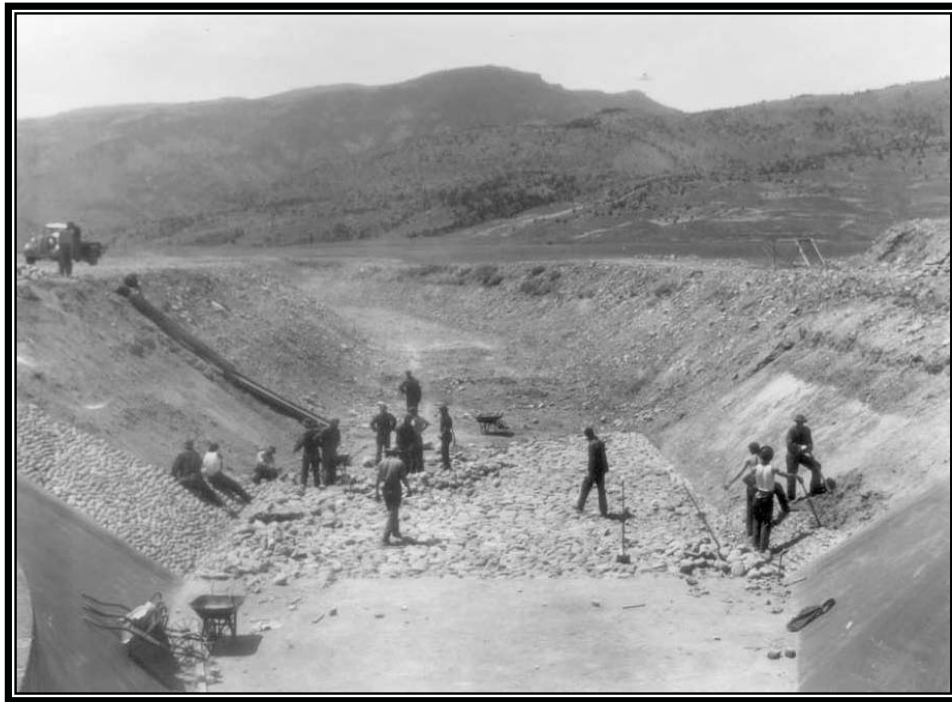
Camp BR-87: Shoshone Project, dry rock paving, Trail Creek, June 5, 1939 (courtesy of Shoshone Irrigation District).
