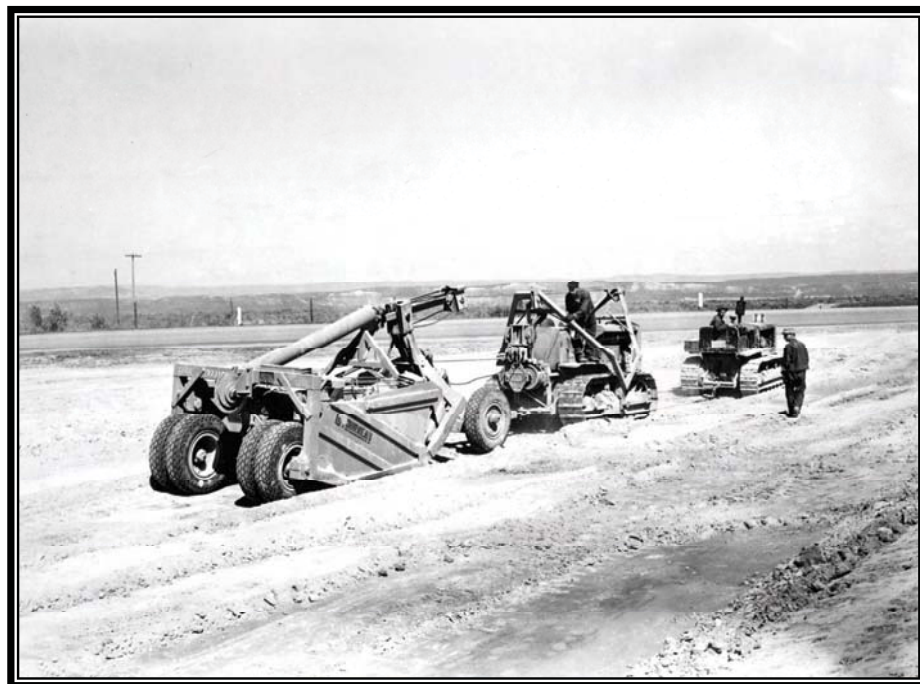
Camp BR-42: Owyhee Project, equipment operated by CCC to obtain material for lateral fill (Box 128, Accession No. 8NN-115-90-011, National Archives, Denver).
