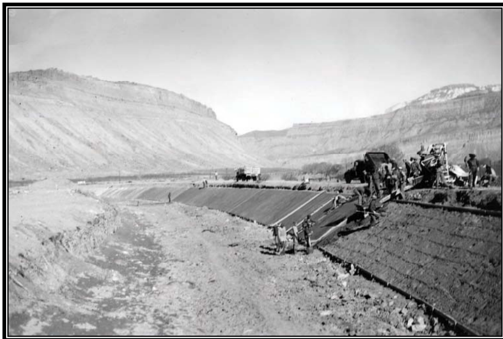
Camp BR-59: Grand Valley Project, placing of concrete lining by CCC on Main Canal, Palisade Division, 1939 (Box 320, Accession No. 8NN-115-90-011, RG 115, National Archives, Denver).
