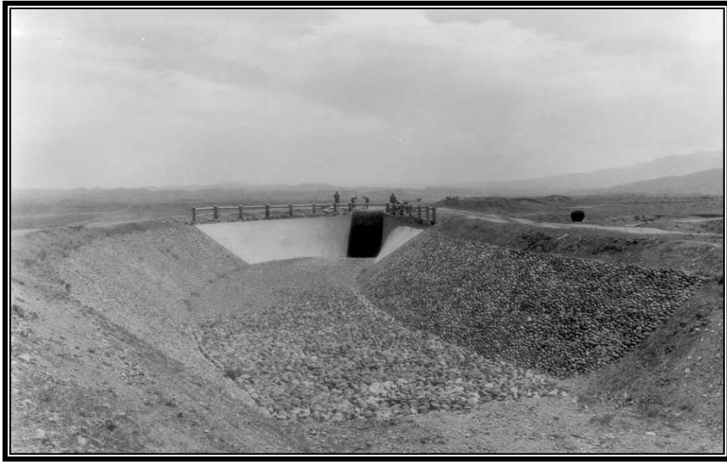
Camp BR-87: Shoshone Project, Heart Mountain Division, completed dry rock paving in the Heart Mountain Canal at the outlet of the North Cottonwood Creek Siphon. Also shows log guardrail constructed by CCC enrollees, June 18, 1940 (Box 2, Entry 31, RG 115, National Archives, Denver).
