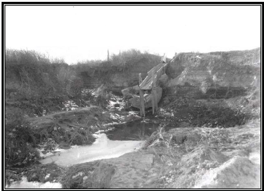
Camp BR-30: Lower Yellowstone Project, drop at end of Main Canal in need of replacement, May 21, 1936 (Box 75, Entry 21, RG 115, National Archives, Denver).
