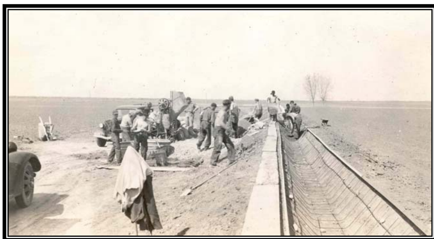
Camp BR-53: North Platte Project, Matheny Lateral, steel in place, ready for concrete, 1937 (Box 122, Entry 22, RG 115, National Archives, Denver).
