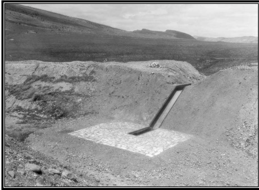
Camp BR-87: Shoshone Project, a completed drainage inlet on Heart Mountain Canal, June 5, 1939 (courtesy of Shoshone Irrigation District).
