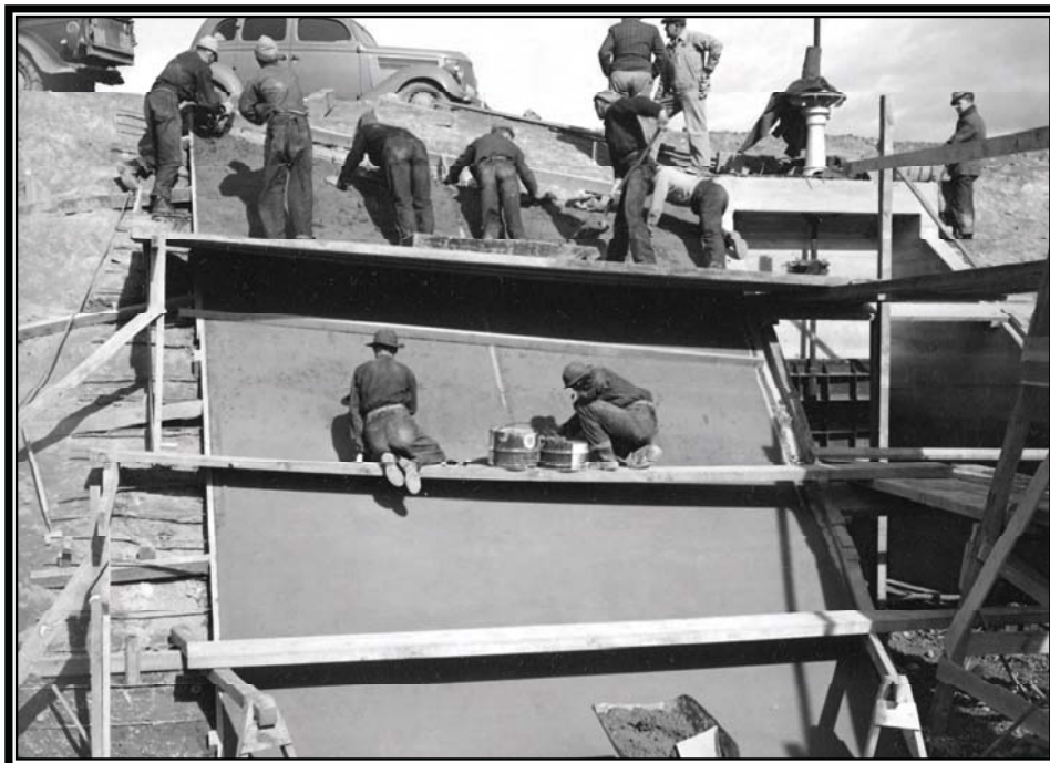
Camp BR-42: Owyhee Project, placing and finishing concrete on new Kingman Check, 1940 (Box 128, Accession No. 8NN-115-90-011, RG 115, National Archives, Denver).
