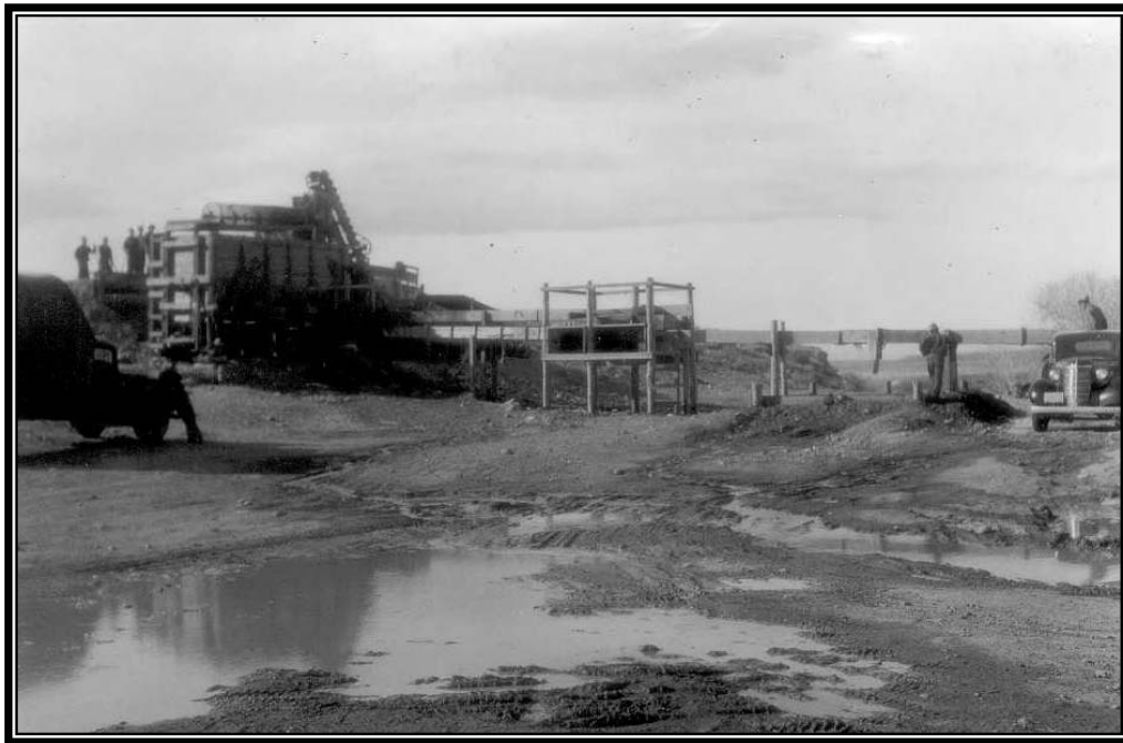
Camp BR-72: Shoshone Project, CCC crushing plant and sand washer, date unknown (courtesy of Shoshone Irrigation District).
