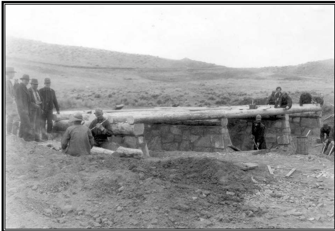
Camp BR-87: Shoshone Project, Heart Mountain Division, log and masonry bridge over Dry Creek, on the operating road for the Heart Mountain Canal, December 13, 1939 (Box 2, Entry 31, RG 115, National Archives, Denver).
