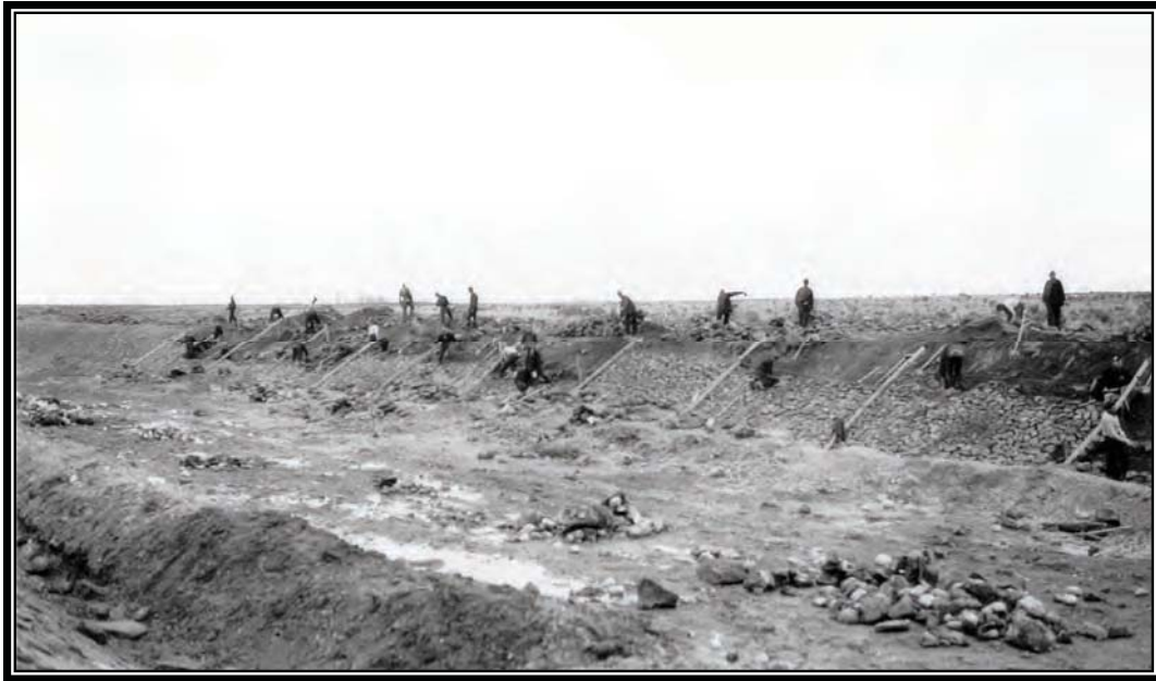
Camp BR-27: Minidoka Project: Subforeman Christian's crew on South Side Main Canal riprap work, February 6, 1941 (Box 1, Entry 31, RG 115, National Archives, Denver).
