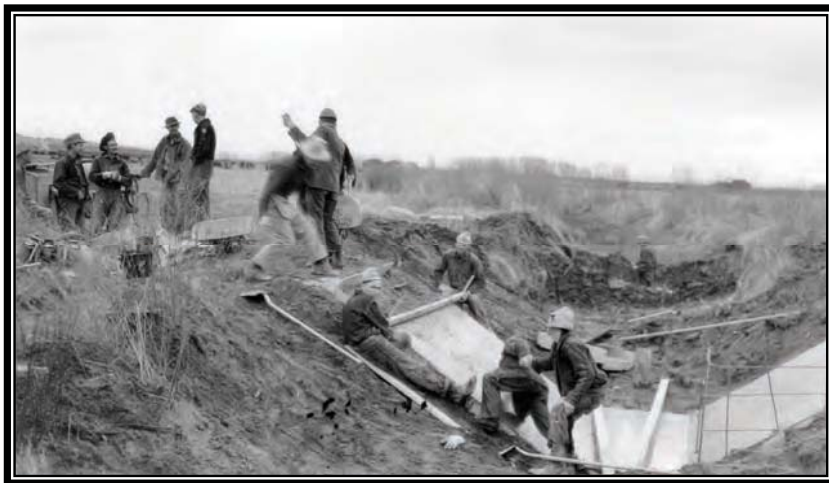
Camp BR-41: Klamath Project, placing of concrete water control structure on G-3 Lateral, January 31, 1941 (Box 1, Entry 31, RG 115, National Archives, Denver).
