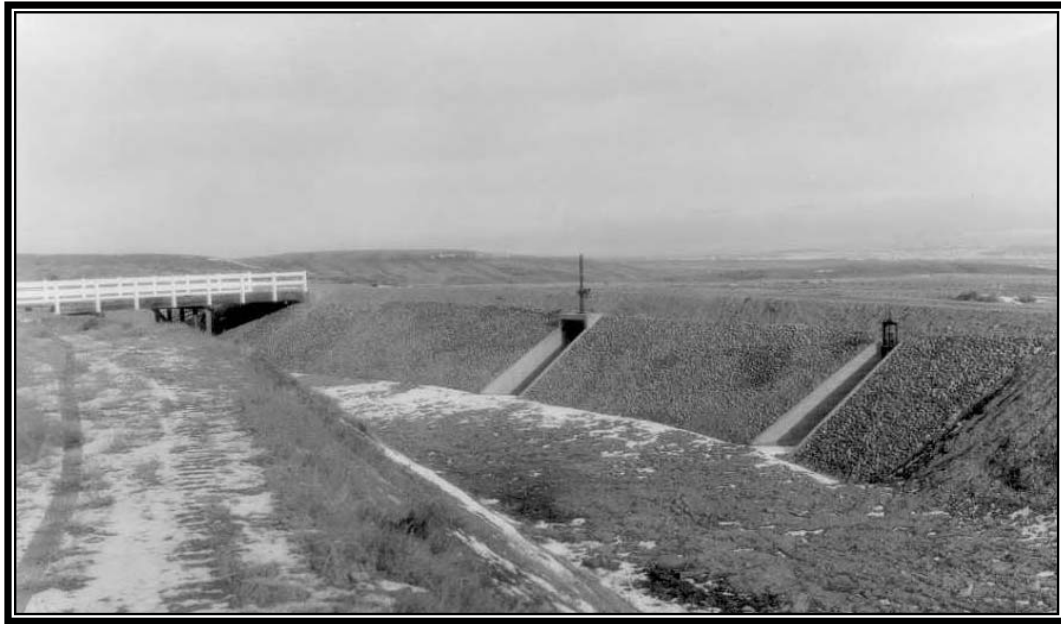
Camp BR-87: Shoshone Project, dry rock paving at Lateral 67, Heart Mountain Canal, showing type of work done on curves in this canal by enrollees, December 2, 1940 (Box 2, Entry 31, RG 115, National Archives, Denver).
