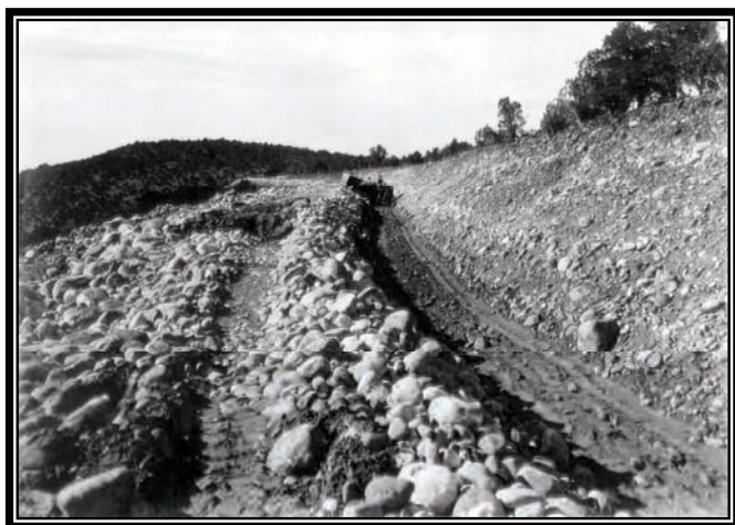
Camp BR-91: Provo River Project, upstream view from station 877+00, Yellowstone Feeder Canal, showing the extremely rocky material encountered for the last 3,000 feet, April 24, 1940 (Box 1, Entry 31, RG 115, National Archives, Denver).
