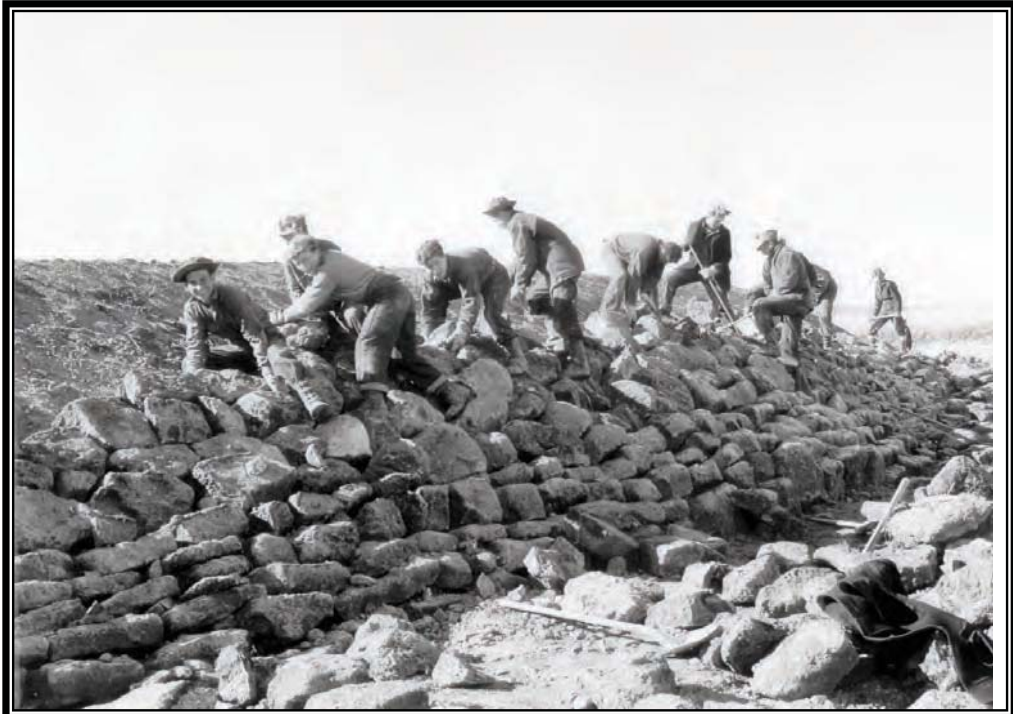
Camp BR-73: Boise Project, enrollees riprapping slopes of Mora Canal, February 21, 1940 (Box 2, Entry 31, RG 115, National Archives, Denver).
