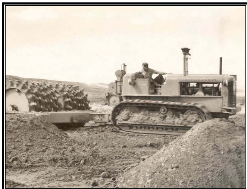
Camp BR-101 or BR-102: Eden Project, enrollee operating a tractor with a sheep's foot roller, coffer dam of Big Sandy Dam, 1941 (Box 156, Entry 10, RG 115, National Archives, Denver).
