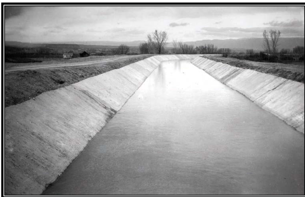
Camp BR-59: Grand Valley Project, section of Main Canal, Palisade Division, showing concrete lining, 1939 (Box 320, Accession No. 8NN-115-90-011, RG 115, National Archives, Denver).
