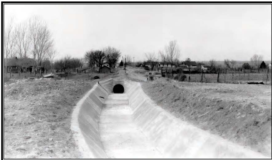
Camp BR-58: Yakima Project, 42-inch monolithic reinforced concrete siphon for replacement of Prosser Flume, transition and lining at outlet end, March 6, 1941 (Box 1, Entry 31, RG 115, National Archives, Denver).
