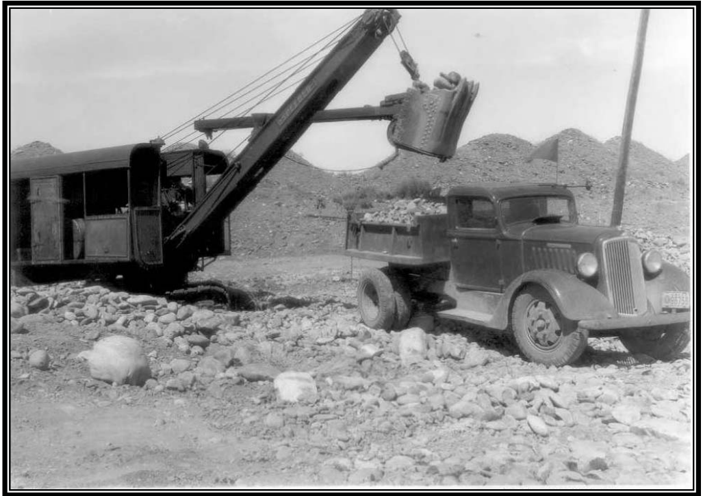
Camp BR-72: Shoshone Project, speeder shovel loading CCC trucks, April 22, 1938 (courtesy of Shoshone Irrigation District).
