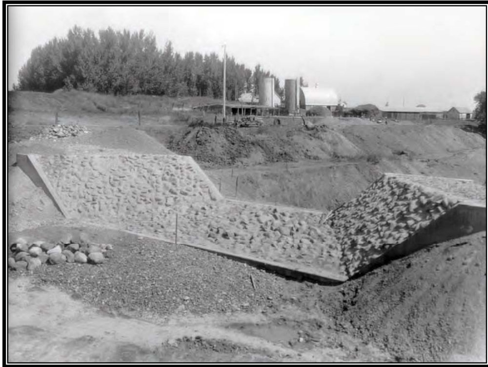
Camp BR-30: Lower Yellowstone Project, a completed drop structure, location and date unknown (Box 1, Entry 31, RG 115, National Archives, Denver).
