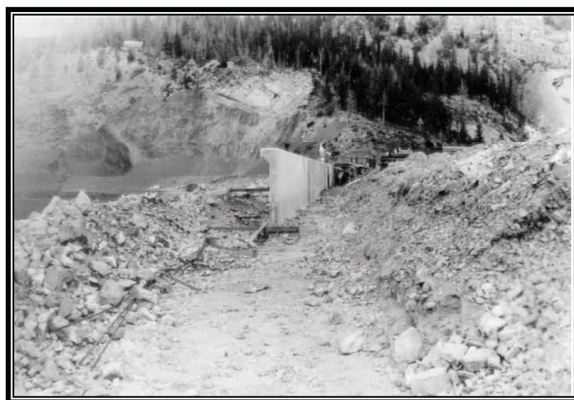
Camp BR-91: Provo River Project, parapet wall at Moon Lake Dam under construction by CCC forces, July 17, 1940 (Box 1, Entry 31, RG 115, National Archives, Denver).
