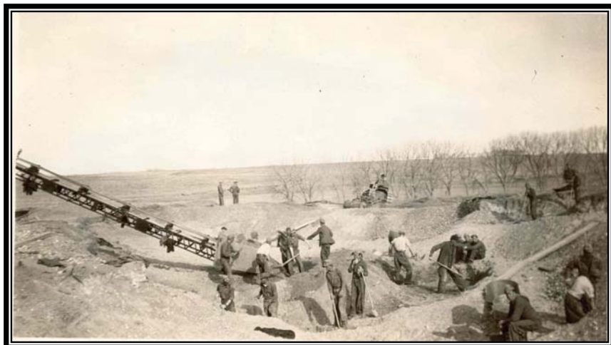
Camp BR-53: North Platte Project, gravel screening plant in operation, May 1936 (Box 122, Entry 22, RG 115, National Archives, Denver).
