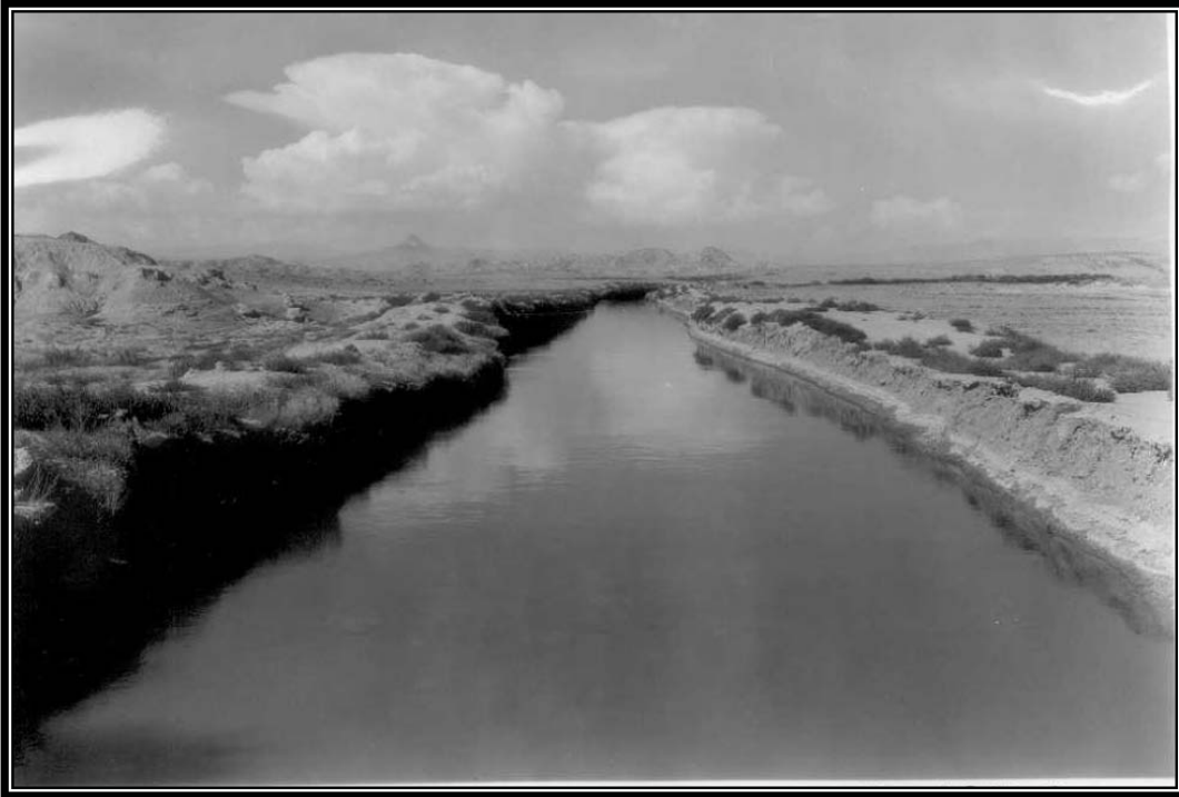
Camp BR-72: Shoshone Project, Willwood Canal showing condition of eroded banks, September 23, 1938 (courtesy of Shoshone Irrigation District).
