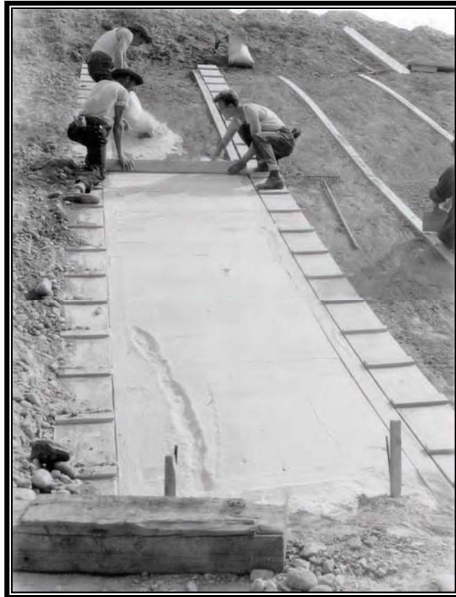
Camp BR-43: Owyhee Project, CCC enrollees working with project forces place a 1-inch layer of bentonite on compacted North Canal immediately above Snively Siphon, March 18, 1941 (Box 1, Entry 31, RG 115, National Archives, Denver).
