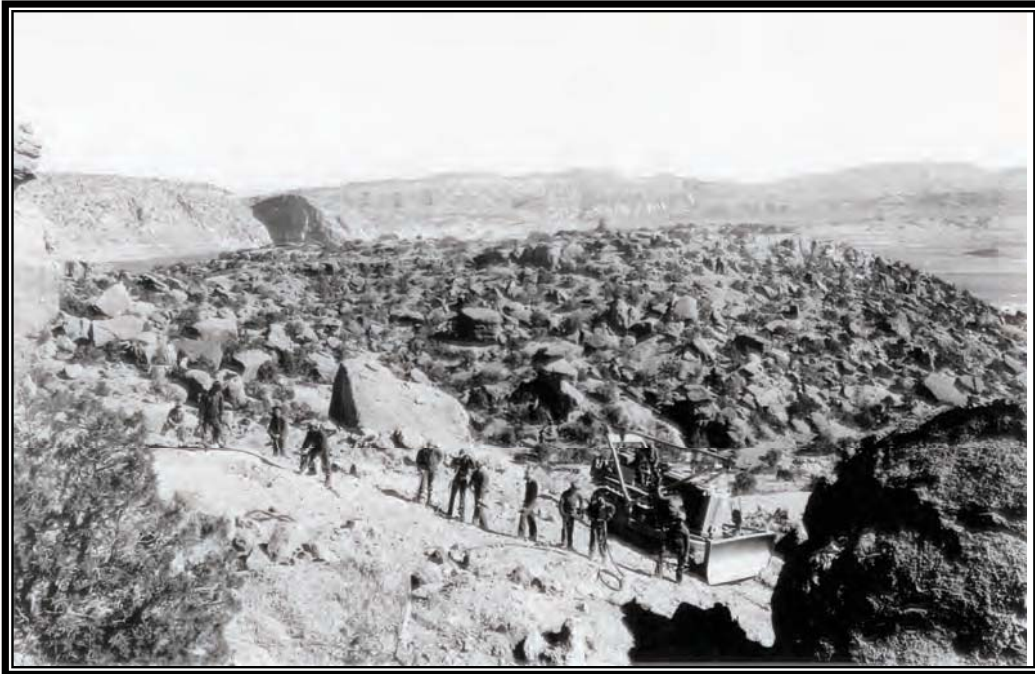
Camp BR-79: Kendrick Project, enrollees drilling for blasting at station 78, February 28, 1940 (Box 2, Entry 31, RG 115, National Archives, Denver).
