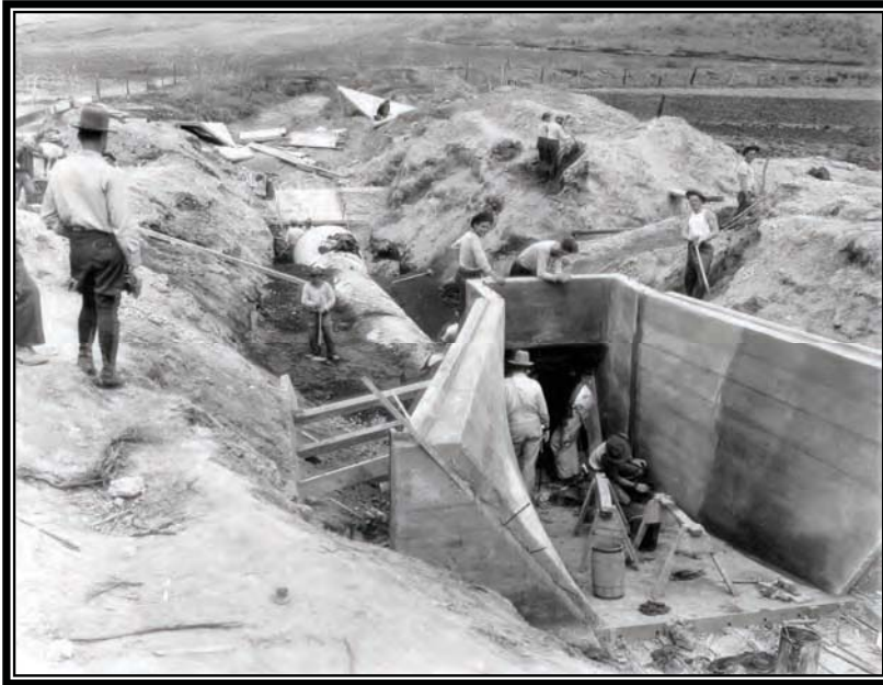
Camp BR-43: Owhyee Project, view of siphon under construction by CCC on Ontario-Nyassa Irrigation District Canal, March 31, 1941 (Box 1, Entry 31, RG 115, National Archives, Denver).
