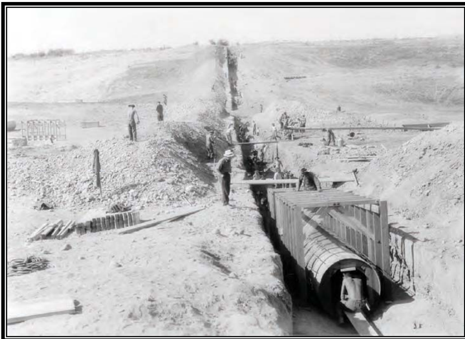
Camp BR-66: Yakima Project, construction of 48-inch monolithic reinforced concrete siphon at station 1216+12 on Lateral "G", looking upstream, enrollees placing forms and steel, September 6, 1940 (Box 1, Entry 31, RG 115, National Archives, Denver).
