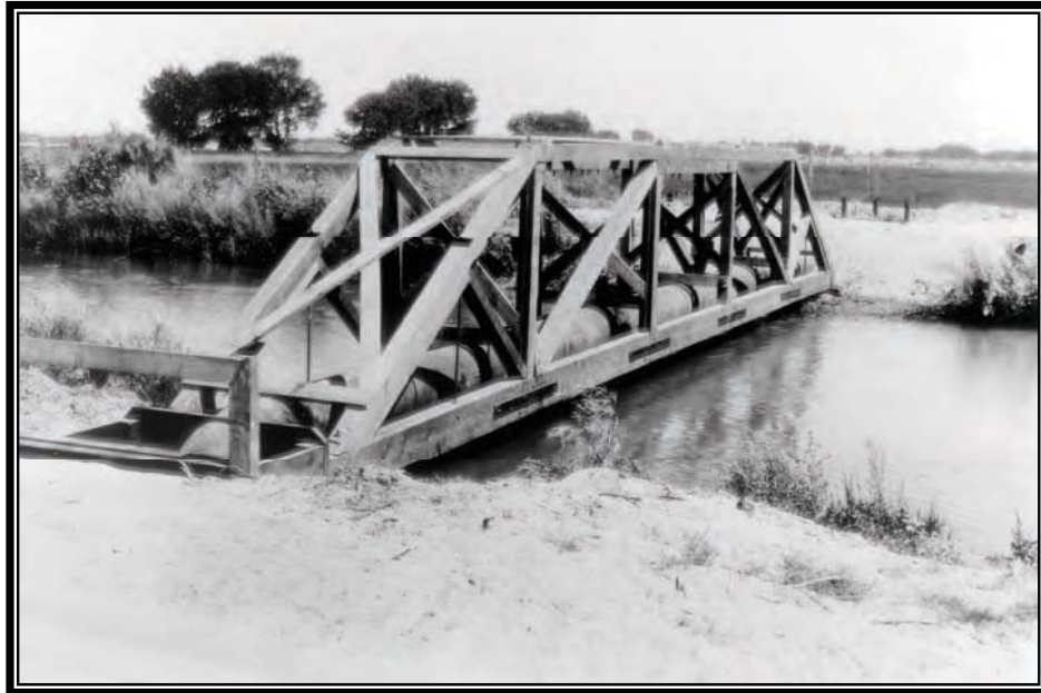
Camp BR-34: Newlands Project, view of lateral carried across a main canal in pipe supported by truss, July 8, 1935 (Box 10, Accession No. 8NS-115-95-112, RG 115, National Archives, Denver).
