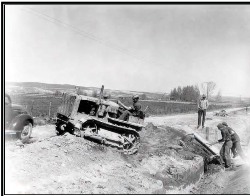
Camp BR-42: Owyhee Project, enrollees building laterals with tractor and fresno scraper, April 14, 1941 (Box 1, Entry 31, RG 115, National Archives, Denver).
