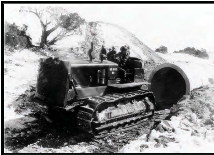
Camp BR-79: Kendrick Project, skidding 60-inch precast concrete pipe into place, Alcova Reservoir scenic drive, February 1939 (Box 36, Entry 22, RG 115, National Archives, Denver).
