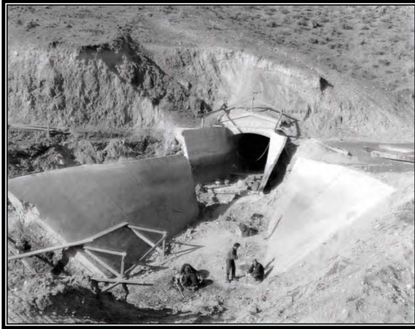
Camp BR-42: Owyhee Project, view of inlet transition, Owyhee River Siphon, showing damage caused by mudslide, January 16, 1940 (Box 1, Entry 31, RG 115, National Archives, Denver).
