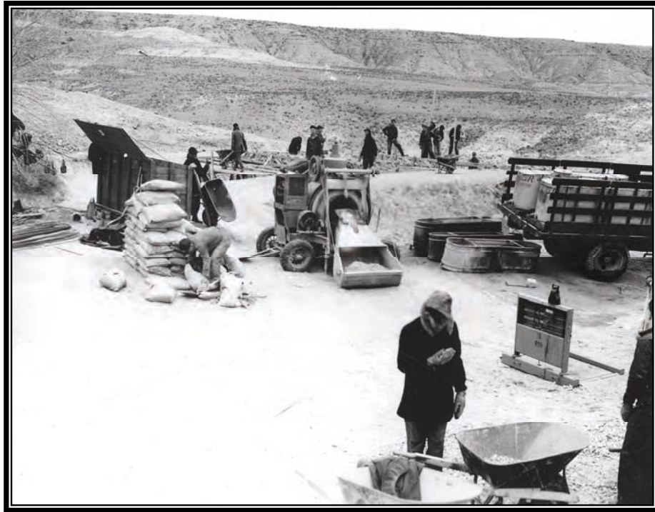
Camp BR-61: North Platte Project, crew setting up to pour intake at Siphon No. 5, January 15, 1941 (Box 1, Entry 31, RG 115, National Archives, Denver).
