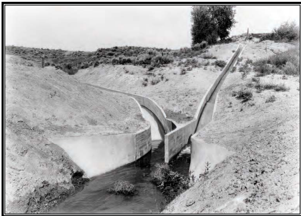
Camp BR-7: Shoshone Project, completed concrete chute on lateral 114, Frannie Division; left chute is for flood water, June 19, 1940 (Box 1, Entry 31, RG 115, National Archives, Denver).
