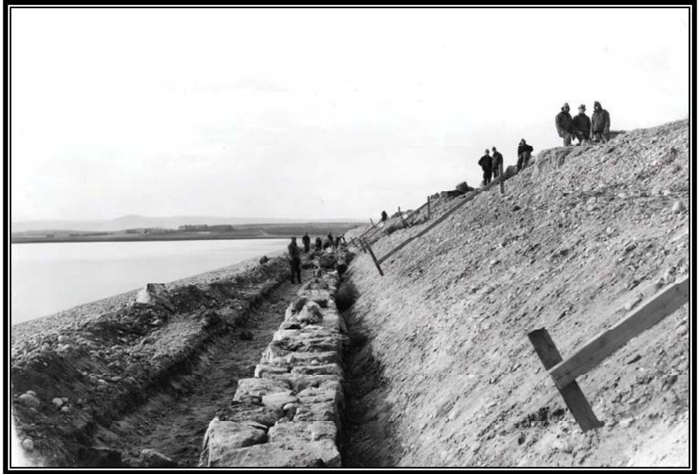
Camp BR-24: Boise Project, enrollees constructing toe wall and preparing to place rocks on slope of Lower Deer Flat Embankment, December 17, 1935 (Box 38, Entry 10, RG 115, National Archives, Denver).
