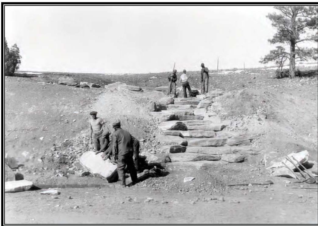
Camps BR-9 and BR-10: North Platte Project, constructing stairway to trail leading to foot of spillway, March 5, 1935 (Box 181, Entry 7, RG 115, National Archives, Denver).
