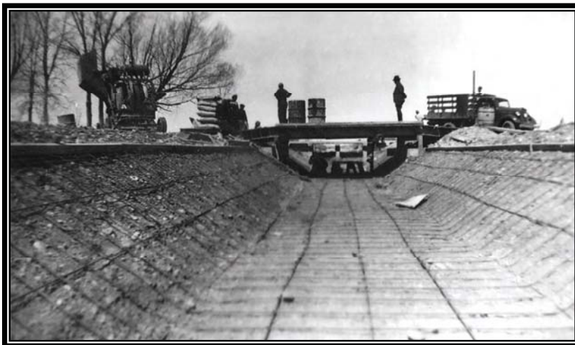
Camp BR-57: Huntley Project, view of Highline Canal concrete lining project after sloping and placing of steel, April 12, 1938 (Box 101, Entry 22, RG 115, National Archives, Denver).
