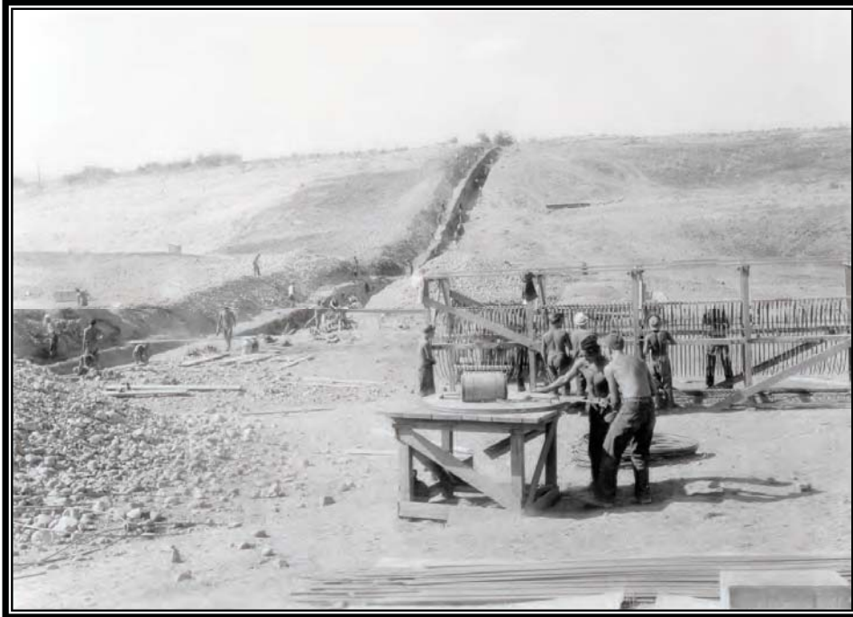
Camp BR-66: Yakima Project, construction of 48-inch monolithic reinforced concrete siphon at station 1216+12 on Lateral "G", looking upstream, showing enrollees bending hoops for siphon barrel reinforcement in foreground, September 6, 1940 (Box 1, Entry 31, RG 115, National Archives, Denver).
