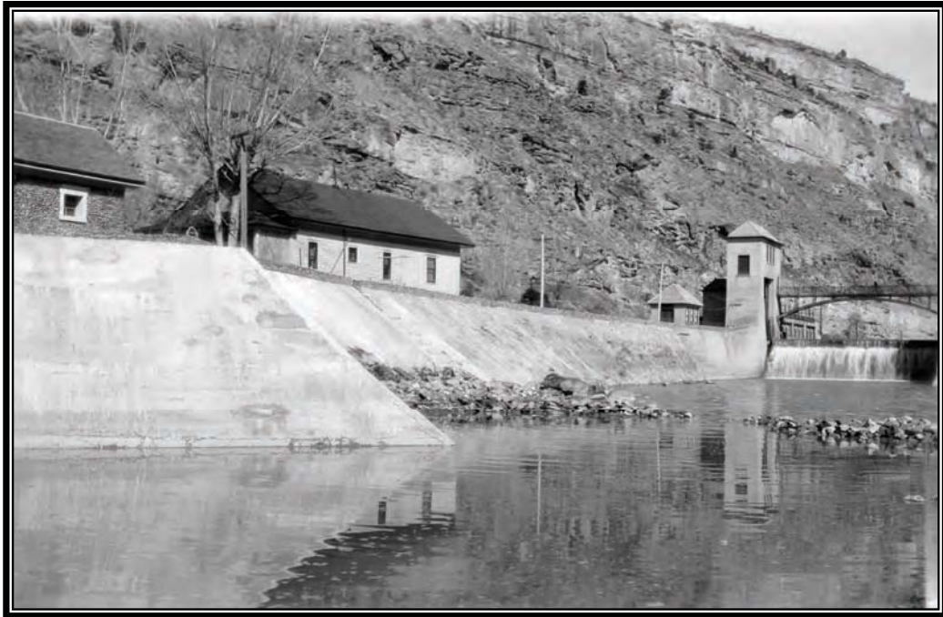
Camp BR-59: Grand Valley Project, finished jetty At Grand Valley Diversion Dam following removal of forms, July 1939 (Box 1, Entry 31, RG 115, National Archives, Denver).
