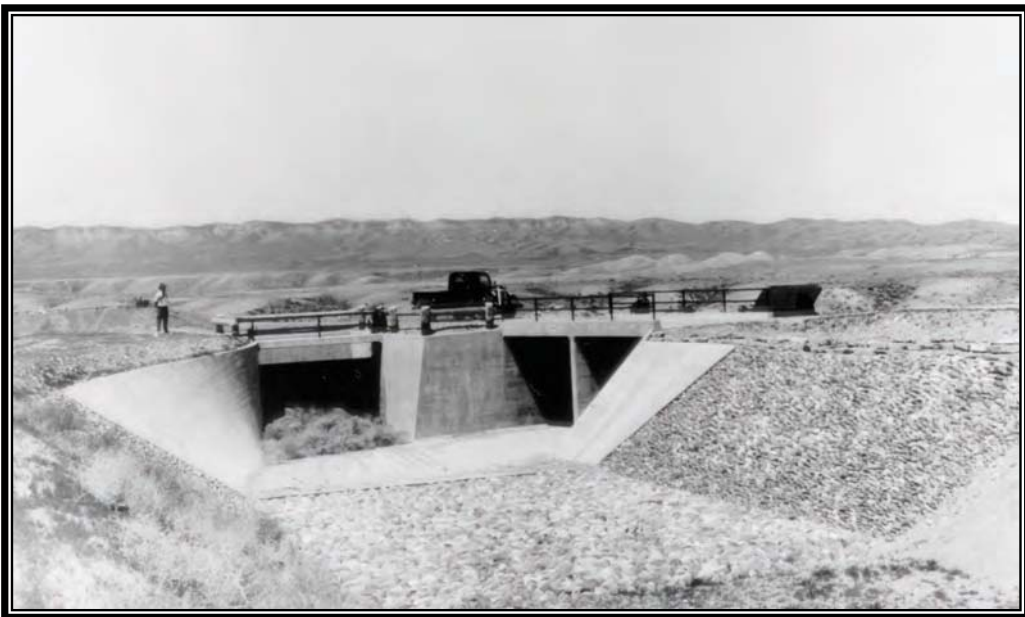
Camp BR-87: Shoshone Project, Heart Mountain Division, completed dry rock paving and log guardrail at the inlet of the North Cottonwood Siphon - Heart Mountain Canal, June 18, 1940 (Box 2, Entry 31, RG 115, National Archives, Denver).
