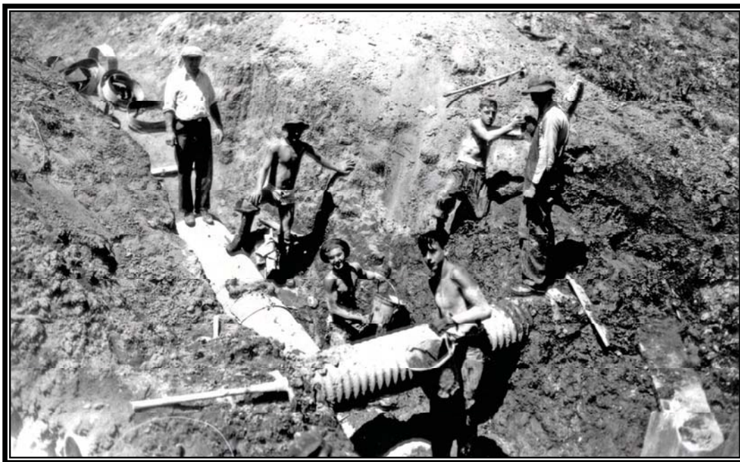
Camp BR-45: Vale Project, construction of concrete pipe inflow at Lateral 385, Willow Creek Unit, May 1937 (Reclamation History Program photo database).
