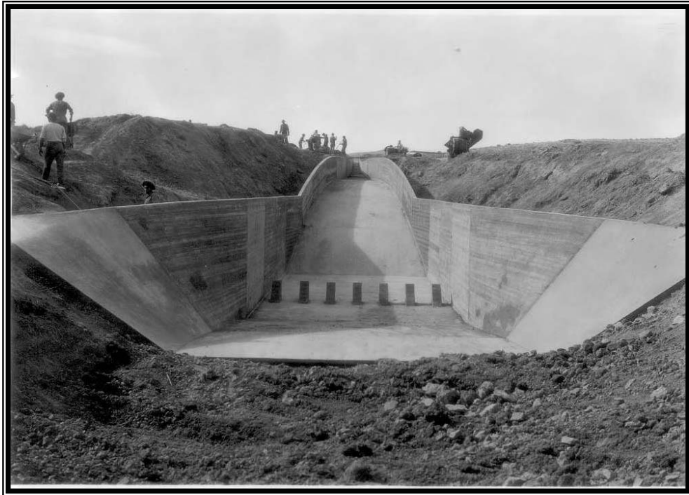
Camp BR-72: Shoshone Project, looking upstream into completed Willwood Canal Chute, date unknown (courtesy of Shoshone Irrigation District).
