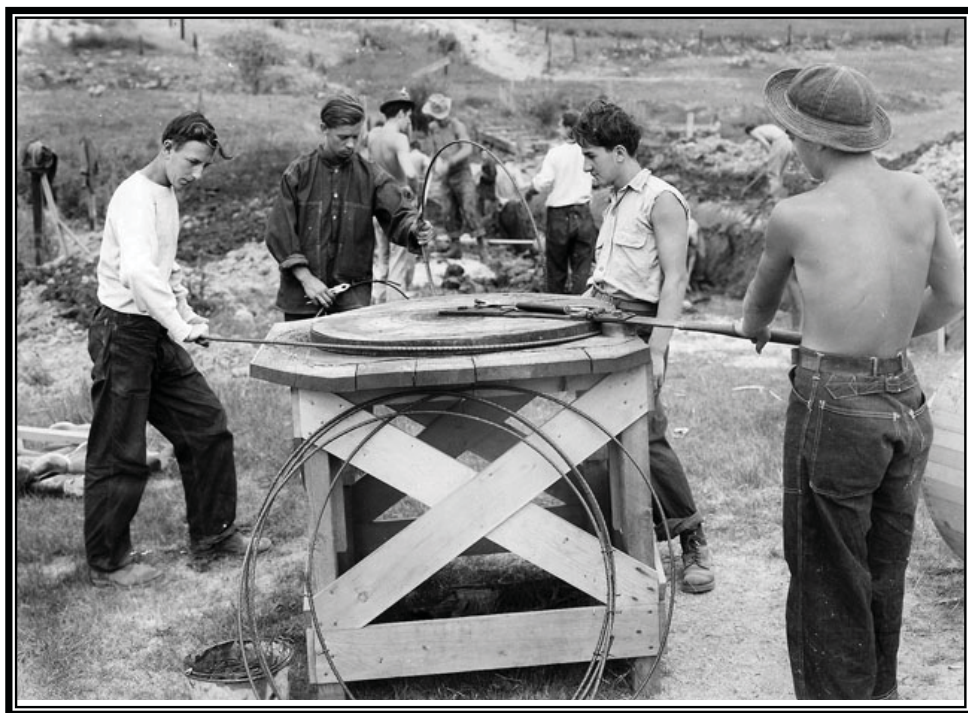
Camp BR-58: Yakima Project, bending reinforcement steel for a 30-inch monolithic siphon at Mathieson Lateral 2.68, Grandview Orchards Tract (Reclamation Columbia-Cascades Area Office, Washington).
