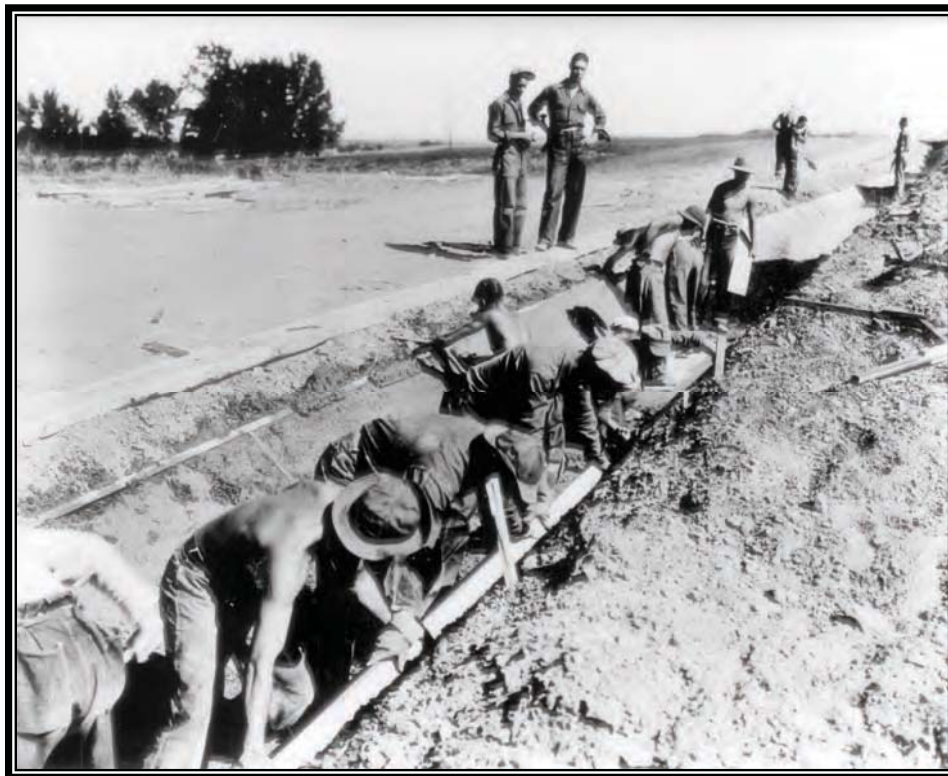
Camp BR-53: North Platte Project, CCC enrollees finishing concrete lining of Seger Lateral, August 22, 1936 (Box 11, Accession No. 8NS-115-95-112, RG 115, National Archives, Denver).
