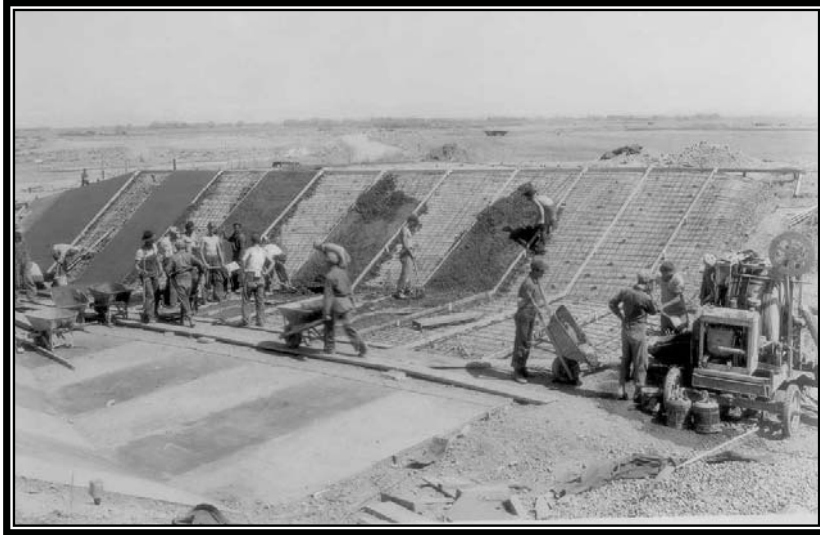
Camp BR-72: Shoshone Project, enrollees mixing, placing, and finishing concrete in the upper transition of Alkali Creek Chute, April 23, 1940 (Box 2, Entry 31, RG 115, National Archives, Denver).
