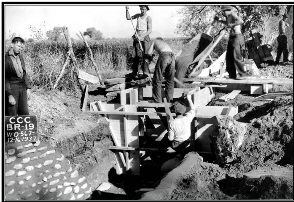
Camp BR-19: Salt River Project, replacing old wooden turnout with concrete one, December 16, 1937 (Box 143, Entry 22, RG 115, National Archives, Denver).
