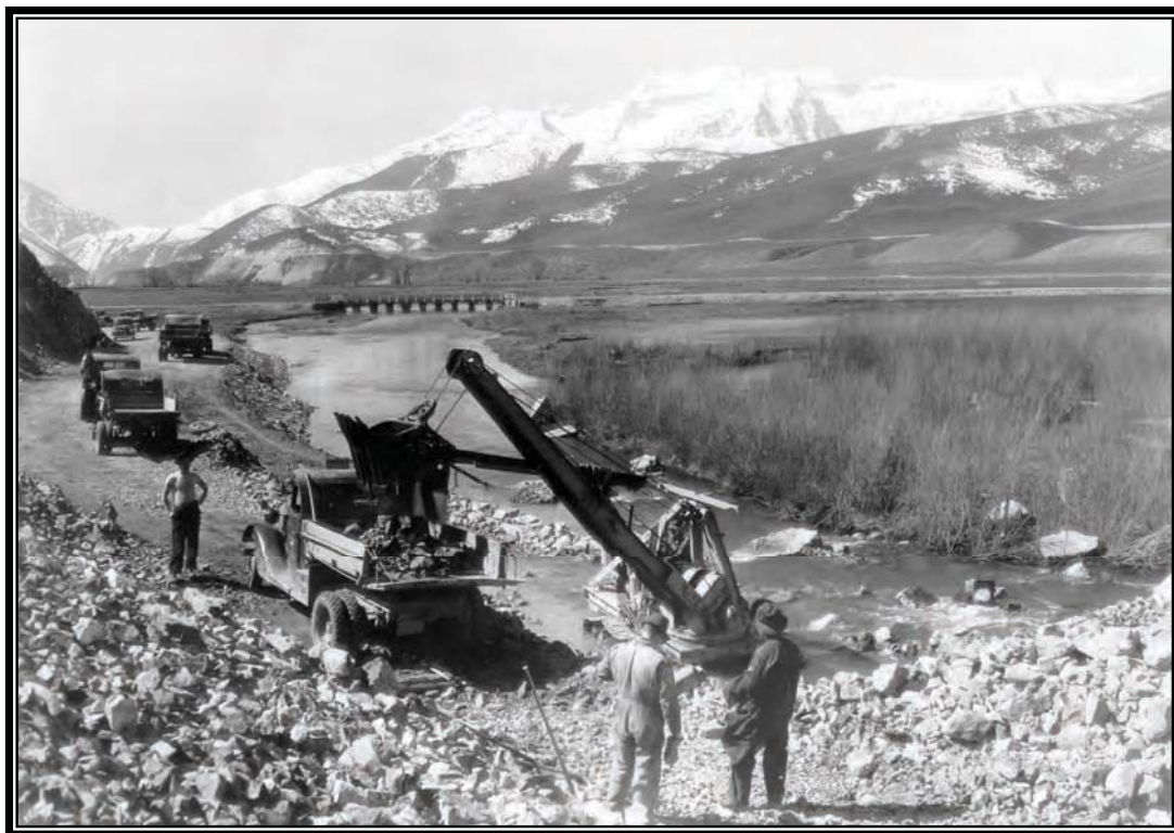
Camp BR-64: Provo River Project, loading rock from waste pile into CCC dump trucks for riprap on Charleston-Midway Highway fill through Deer Creek Reservoir, March 26, 1941 (Box 1, Entry 31, RG 115, National Archives, Denver).
