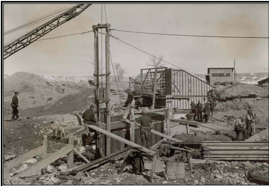
Camp BR-11: Moon Lake Project, driving laminated timber piling for cutoff wall along axis at Duchesne Feeder Canal diversion structure, March 2, 1939 (Accession No. 8NN-115-90-011, RG 115, National Archives, Denver).
