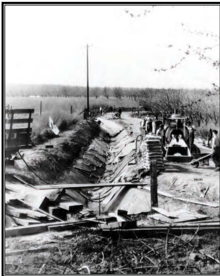
Camp BR-86: Yakima Project, concrete lining at Main Lateral, Granger Irrigation District, March 26, 1941 (Box 2, Entry 31, RG 115, National Archives, Denver).
