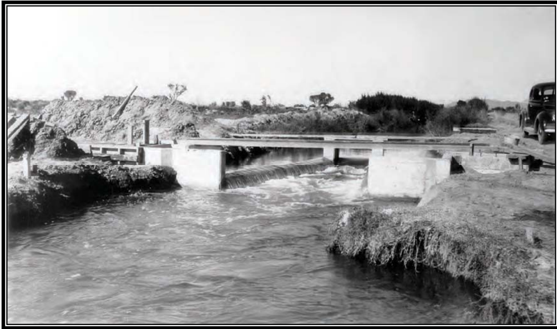
Camp BR-74: Yuma Project, check in Central Canal and Turnout to Cavanah Lateral, December 12, 1939 (Box 2, Entry 31, RG 115, National Archives, Denver).
