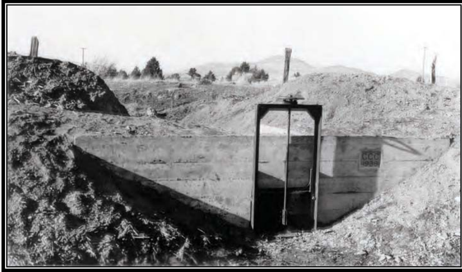
Camp BR-41: Klamath Project, finished concrete turnout on F-1 Canal at station 95-00, December 21, 1939 (Box 1, Entry 31, RG 115, National Archives, Denver).
