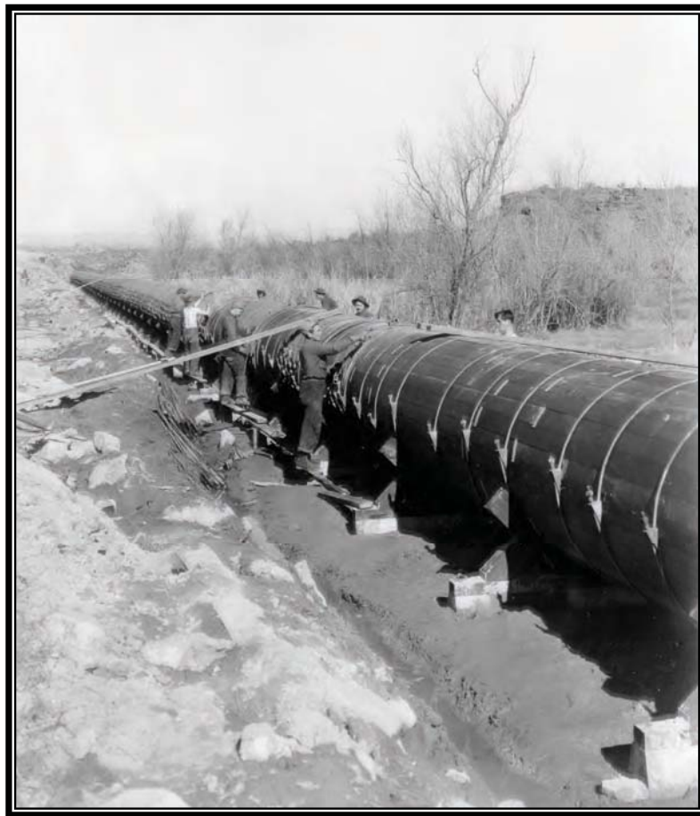
Camp BR-58: Yakima Project, Mabton Siphon replacement, placing bands on new 56-inch creosoted wood stave pipe. View looking upstream, March 6, 1941 (Box 1, Entry 31, RG 115, National Archives, Denver).
