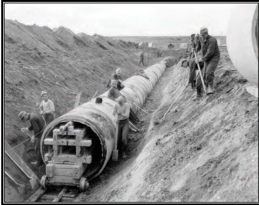
Camp BR-42: Owyhee Project, enrollees placing concrete pipe and tamping backfill, Ontario Nyassa Pumping Plant discharge pipe, February 8, 1940 (Box 1, Entry 31, RG 115, National Archives, Denver).
