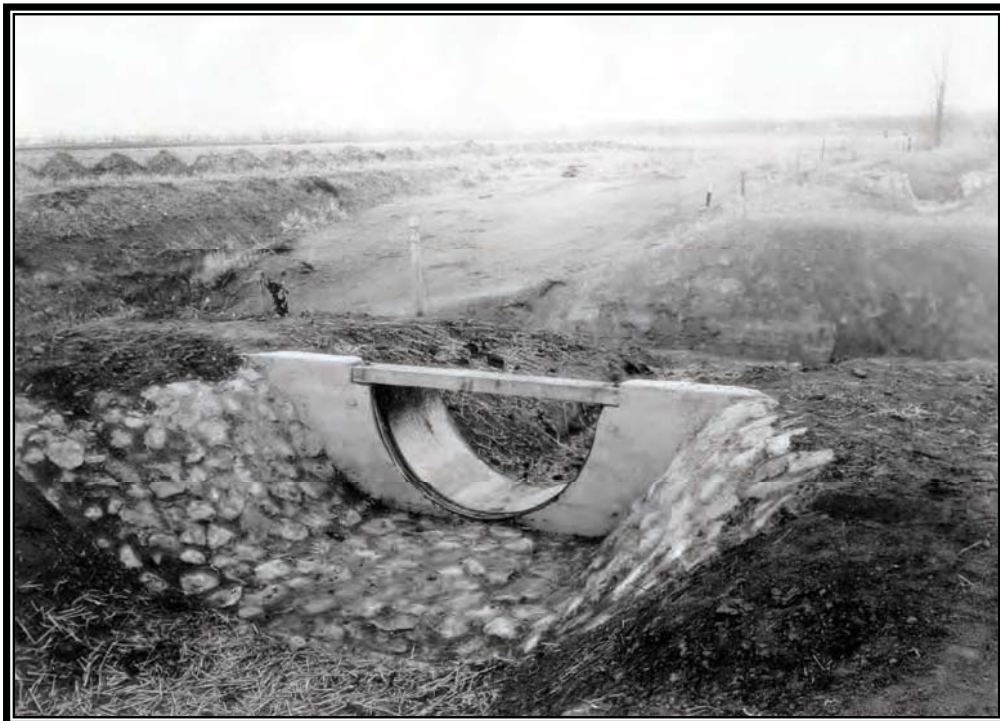
Camp BR-69: Milk River Project, flume on Dodson North Lateral 104 after construction of headwalls, December 14, 1939 (Box 1, Entry 31, RG 115, National Archives, Denver).
