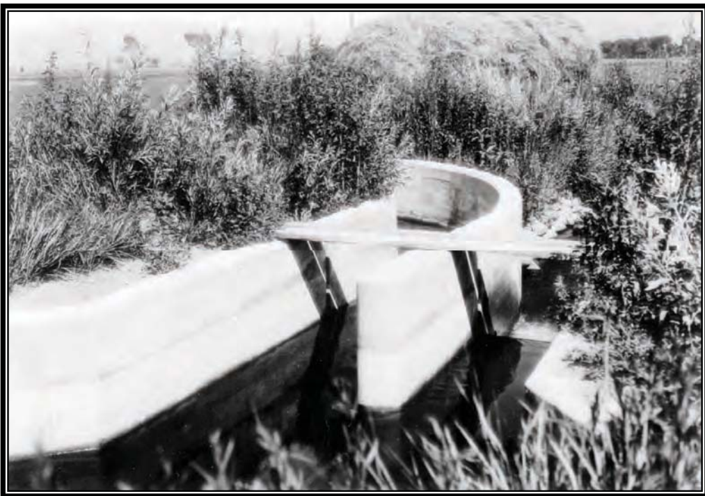
Camp BR-37: Truckee River Project, view showing typical concrete canal division box built by enrollees, July 13, 1936 (Box 19, Accession No. 8NS-115-95-112, RG 115, National Archives, Denver).
