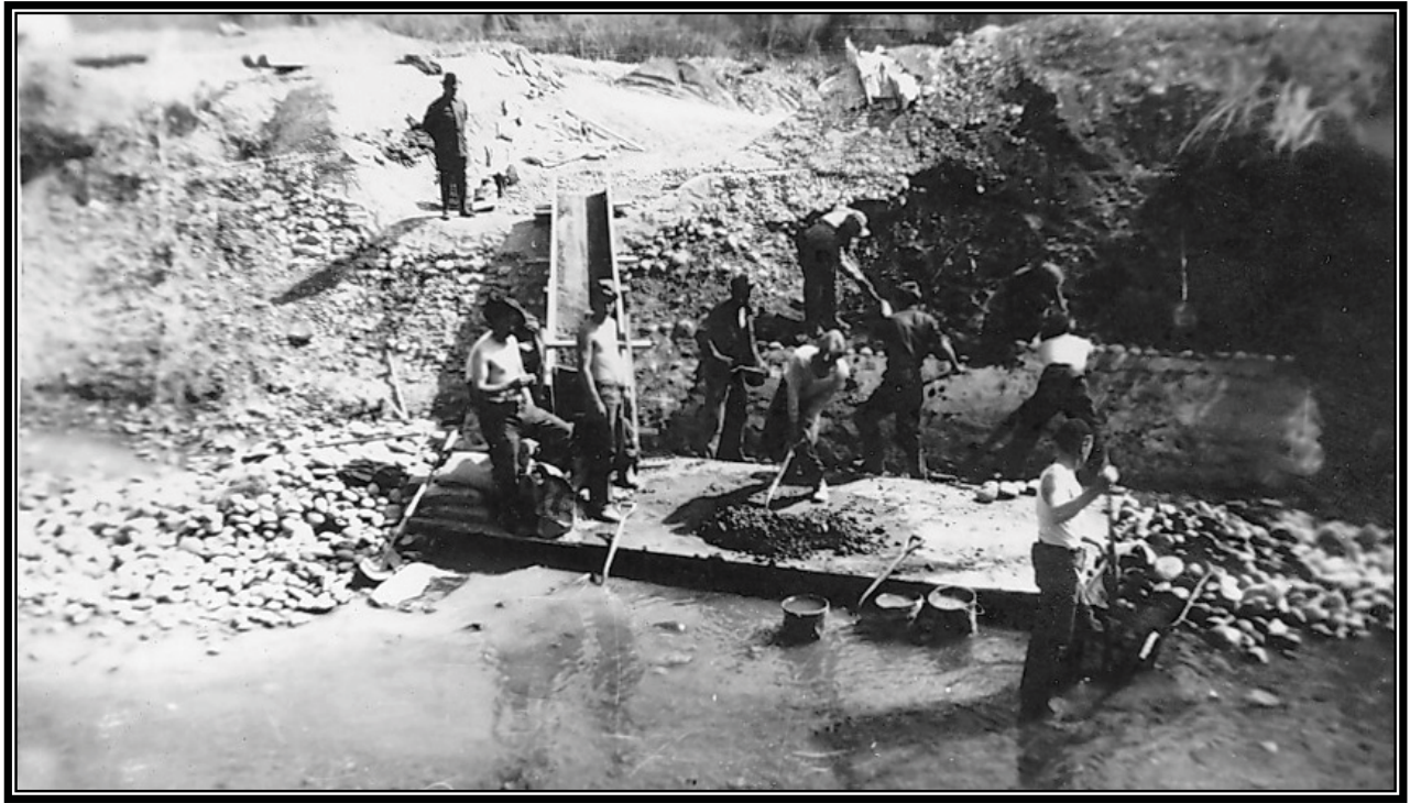
Camp BR-57: Huntley Project, preparing and placing grouting on Main Canal, April 12, 1938 (Box 101, Entry 22, RG 115, National Archives, Denver).
