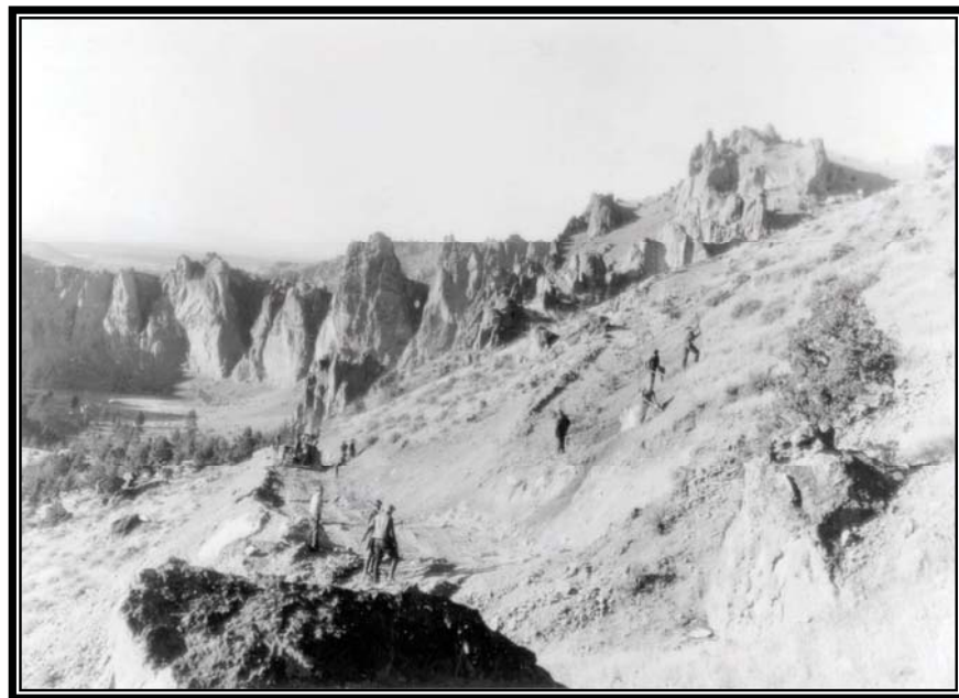
Camp BR-88, BR-89, and BR-90: Deschutes Project, enrollees excavating construction road near Tunnel No. 1 "Smith Rock" Section, North Unit Main Canal, February 7, 1941 (Box 2, Entry 31, RG 115, National Archives, Denver).
