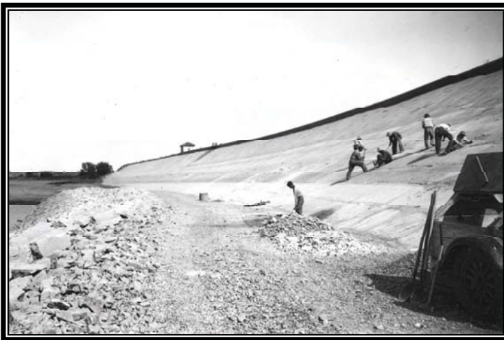
Figure 2.5 Repairing Belle Fourche Dam, Camp Fruitdale (BR-2), Belle Fourche Project, South Dakota, 1940.
