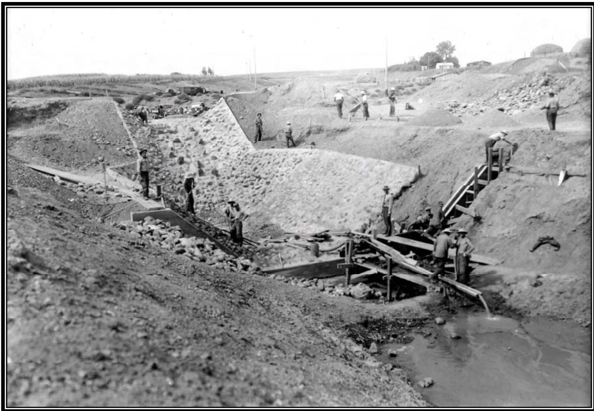
Camp BR-30: Lower Yellowstone Project, enrollees building drop structure, location and date unknown (Box 1, Entry 31, RG 115, National Archives, Denver).
