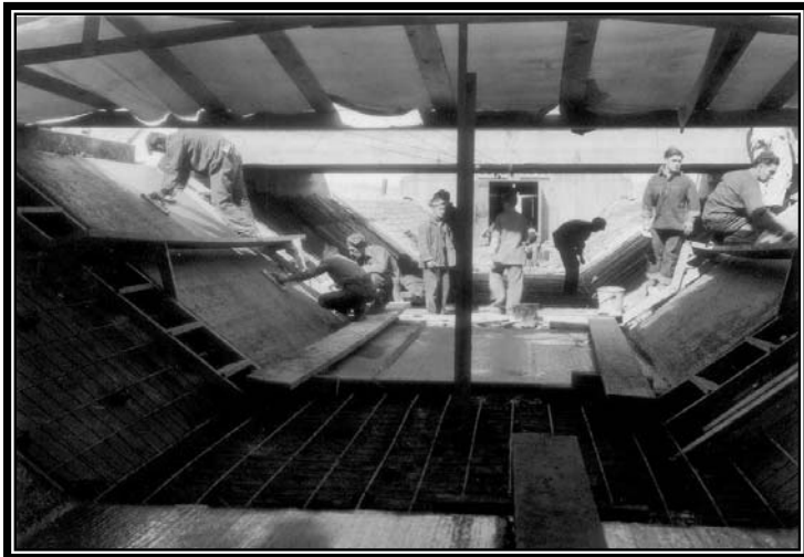
Camp BR-72: Shoshone Project, enrollees finishing concrete in Alkali Creek Chute, 1940 (courtesy of Shoshone Irrigation District).
