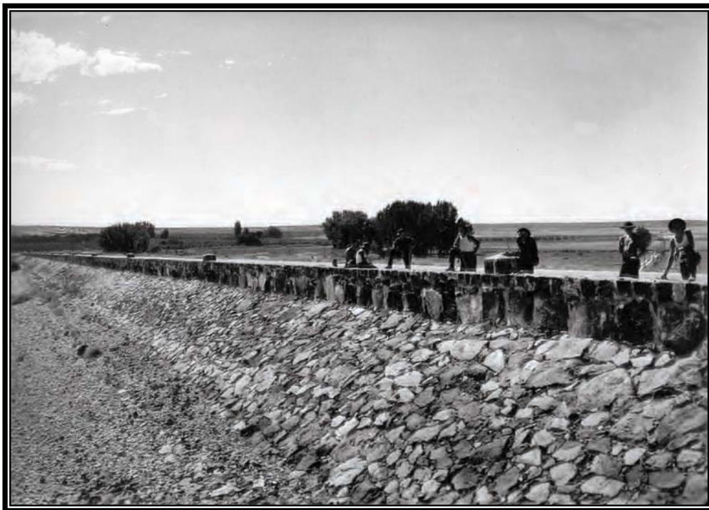
Camp BR-24: Boise Project, rock paving and parapet on Lower Deer Flat Embankment placed by CCC enrollees, 1937 (Box 39, Entry 10, RG 115, National Archives, Denver).
