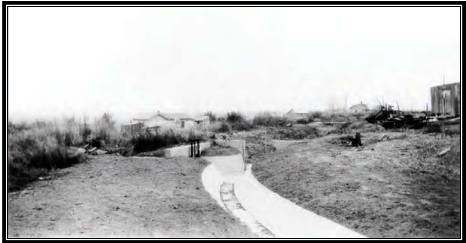
Camp BR-83: North Platte Project, concrete lining: completed section of Gantz Lateral, off Springer Main Lateral, November 4, 1940 (Box 2, Entry 31, RG 115, National Archives, Denver).
