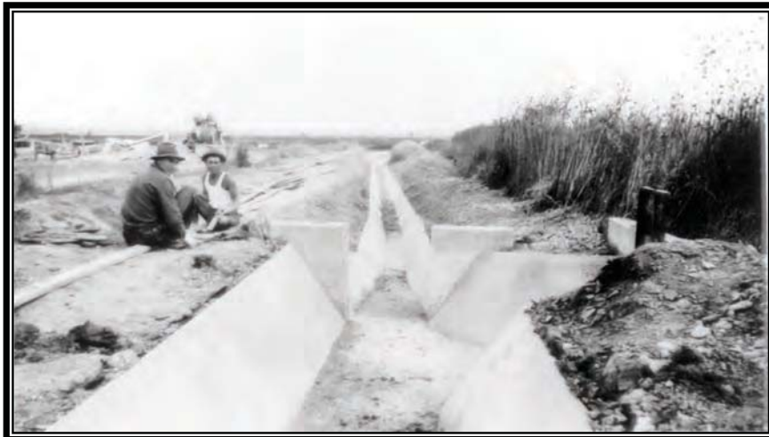
Camp BR-83: North Platte Project, cattle guard nearing completion, September 4, 1939 (Box 2, Entry 31, RG 115, National Archives, Denver).
