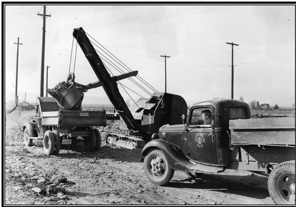
Camp BR-58: Yakima Project, strengthening of Main Canal banks, loading dump trucks with power shovels, February 16, 1939 (Reclamation Columbia-Cascades Area Office, Washington).
