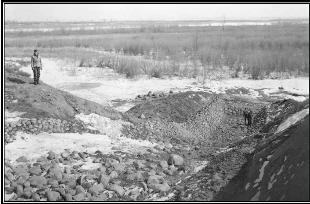
Camp BR-97: Buford-Trenton Project, CCC drainage crossing and drop, 1942 (Box 75, Entry 10, RG 115, National Archives, Denver).
