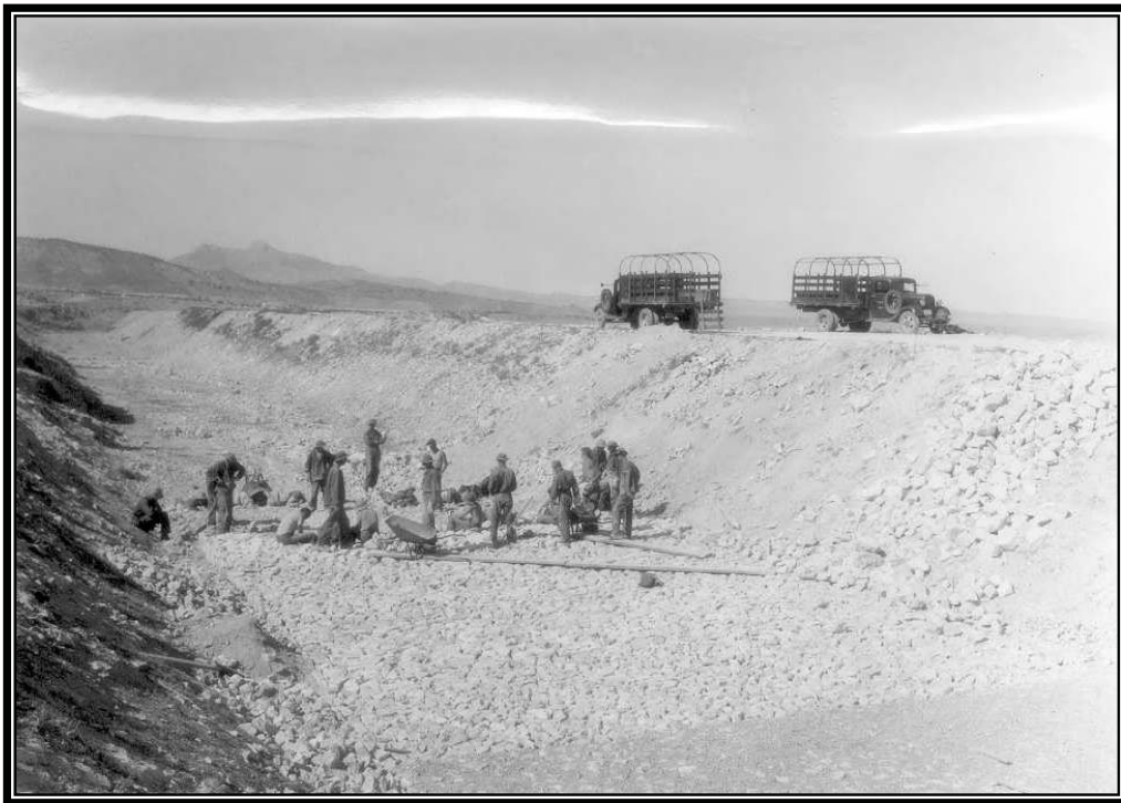
Camp BR-72: Shoshone Project, enrollees placing dry rock paving, date unknown (courtesy of Shoshone Irrigation District).
