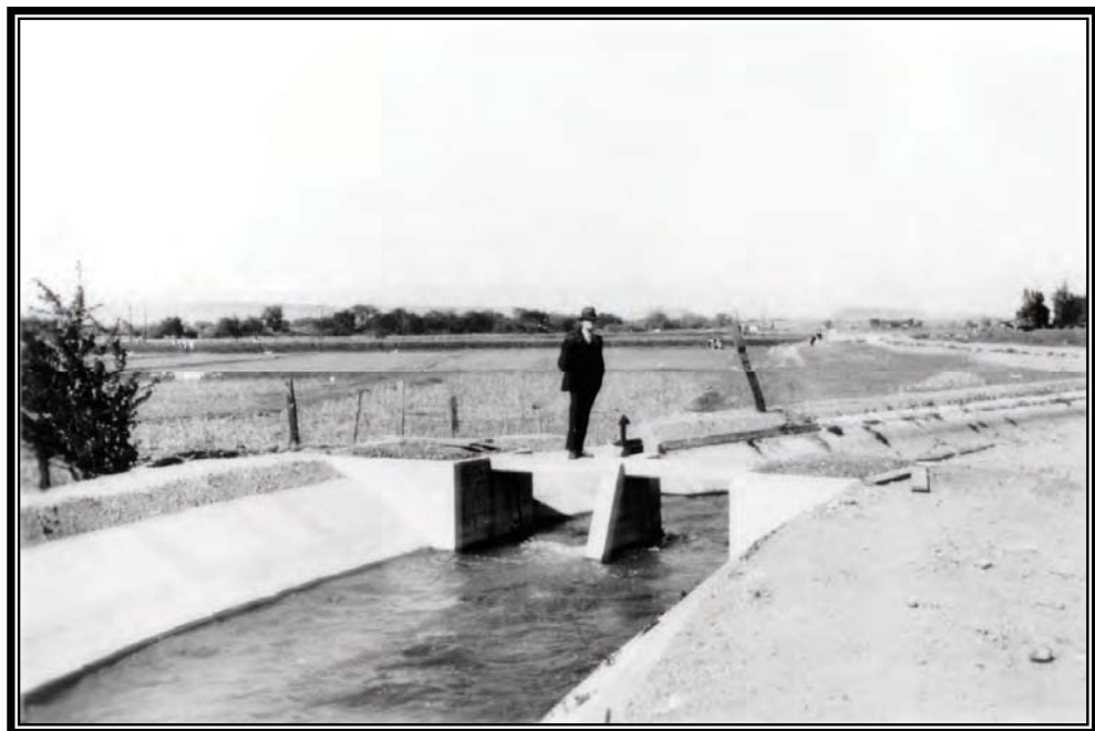
Camp BR-78: Orland Project, completed check and section of completed canal on Lateral 100, date unknown (Box 2, Entry 31, RG 115, National Archives, Denver).
