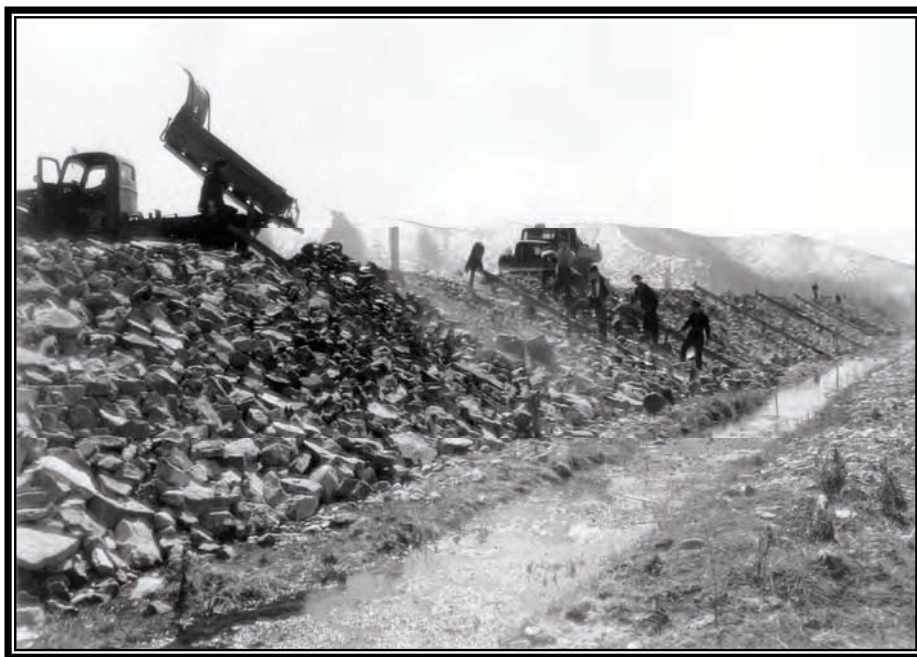
Camp BR-64: Provo River Project, CCC forces placing riprap on Charleston-Midway Highway fill through upper end of Deer Creek Reservoir, March 26, 1941 (Box 1, Entry 31, RG 115, National Archives, Denver).
