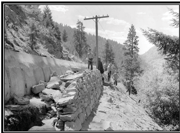
Camp BR-66: Yakima Project, building rock riprap retaining wall for foot trail widening and improvement along Tieton Main Canal, September 7, 1939 (Reclamation Columbia-Cascades Area Office, Washington).
