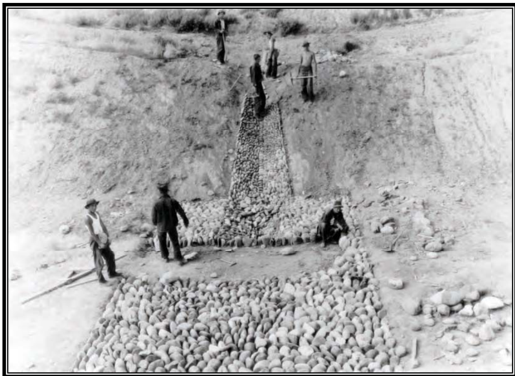
Camp BR-87: Shoshone Project, enrollees constructing a drain inlet into Heart Mountain Canal. The portion of the structure on the slope will be cement grouted, September 11, 1940 (Box 2, Entry 31, RG 115, National Archives, Denver).
