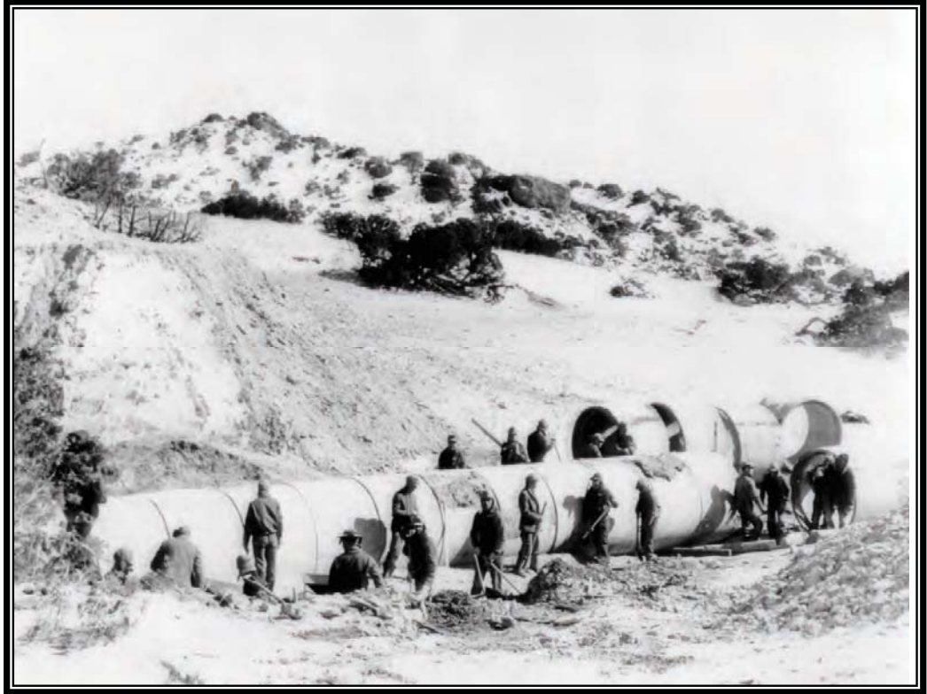
Camp BR-79: Kendrick Project, placing 60-inch precast concrete pipe, February 1939 (Box 36, Entry 22, RG 115, National Archives, Denver).
