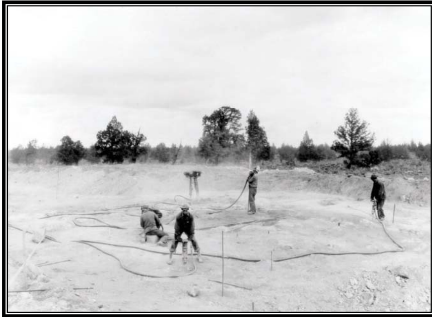
Camp BR-88, BR-89, and BR-90: Deschutes Project, enrollee drilling crew working on North Unit Main Canal, station 1001, March 27, 1940 (Box 2, Entry 31, RG 115, National Archives, Denver).
