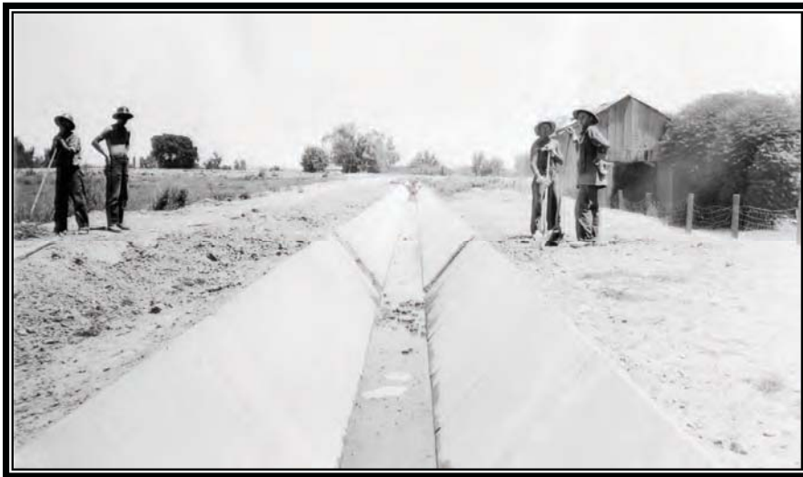
Camp BR-13: Yuma Project, concrete precast slabs placed in Woods Lateral, September 20, 1939 (Box 1, Entry 31, RG 115, National Archives, Denver).
