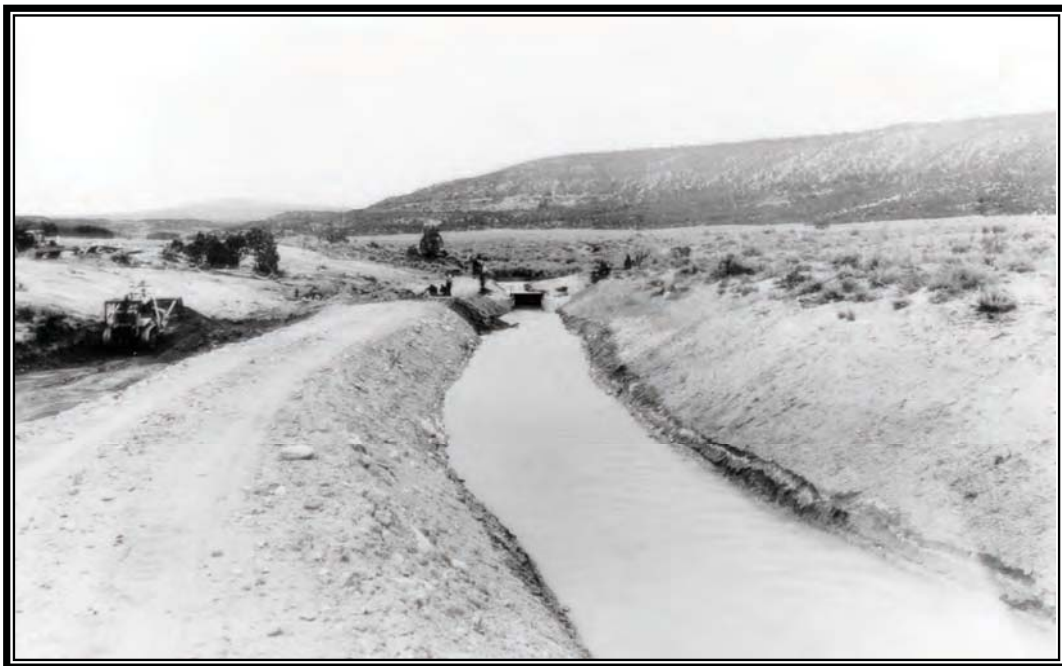
Camp BR-91: Provo River Project, Section of Yellowstone Feeder Canal with diversion works at station 599 in background, cleanup work in progress on diversion works, July 17, 1940 (Box 1, Entry 31, RG 115, National Archives, Denver).
