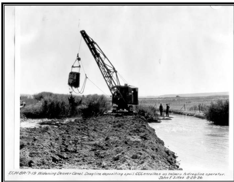
Camp BR-7: Shoshone Project, enrollees working with dragline to widen Deaver Canal; note former width of canal, August 28, 1936 (courtesy of Shoshone Irrigation District).
