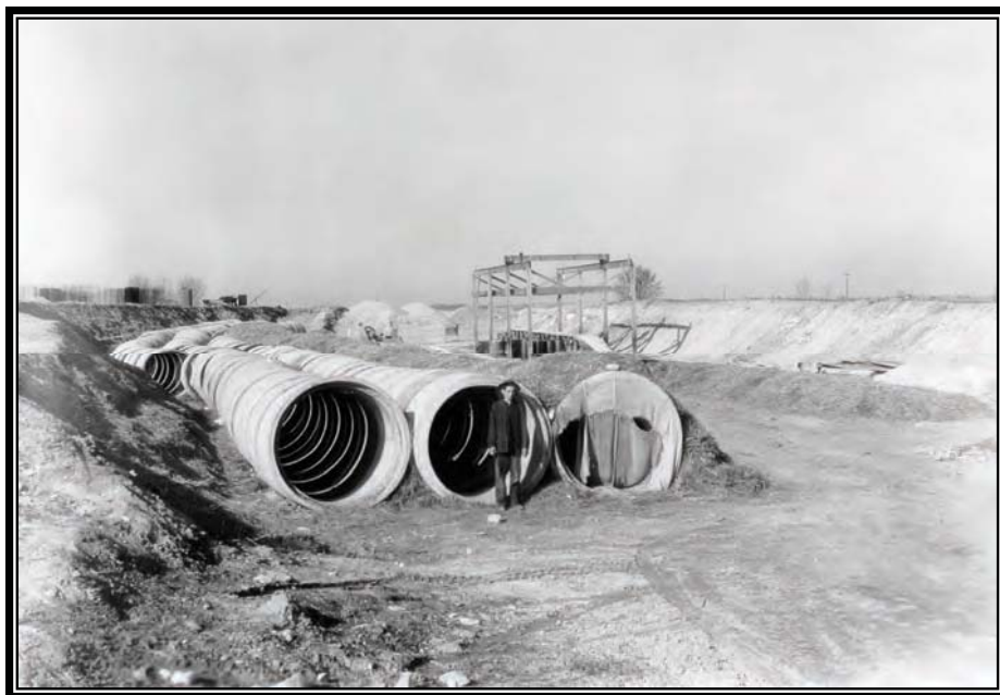
Camp BR-73: Boise Project, plant for manufacturing concrete pipe operated by CCC, March 13, 1941 (Box 2, Entry 31, RG 115, National Archives, Denver).
