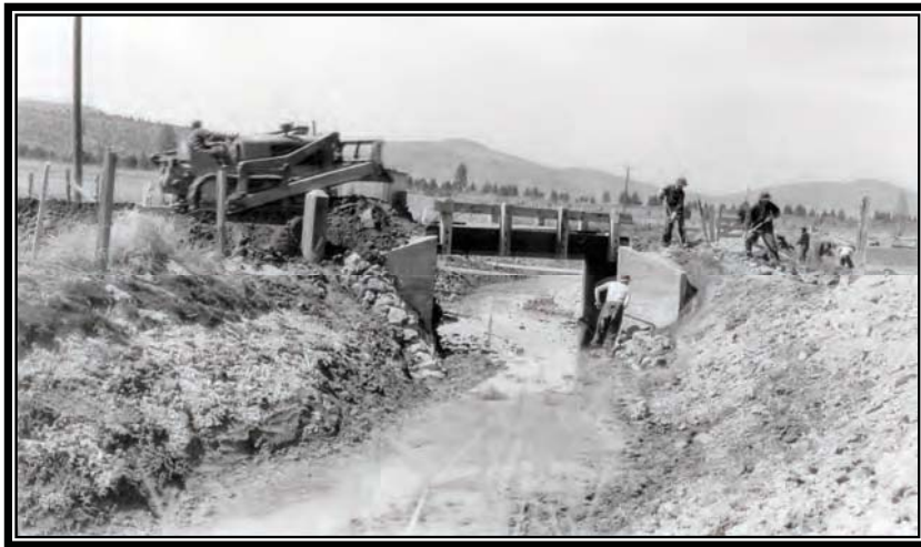
Camp BR-41: Klamath Project, "F" Canal near Olene, Oregon, building approach for bridge and riprapping around bridge abutment, April 11, 1940 (Box 1, Entry 31, RG 115, National Archives, Denver).
