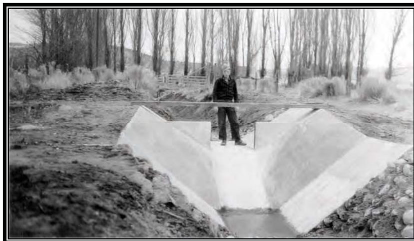
Camp BR-41: Klamath Project, finished concrete water control structure on D-15 Lateral, January 31, 1941 (Box 1, Entry 31, RG 115, National Archives, Denver).
