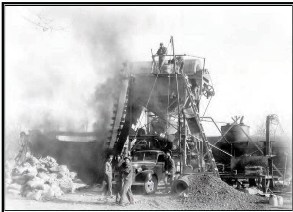
Camp BR-58: Yakima Project, asphalt mixing plant for experimental asphaltic concrete lining project, November 13, 1939 (Box 1, Entry 31, RG 115, National Archives, Denver).
