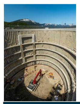
The novel helix fish passage design developed by Reclamation's Hydraulics Lab in Denver, Colorado is being constructed at Cle Elum Dam near Yakima, Washington.
