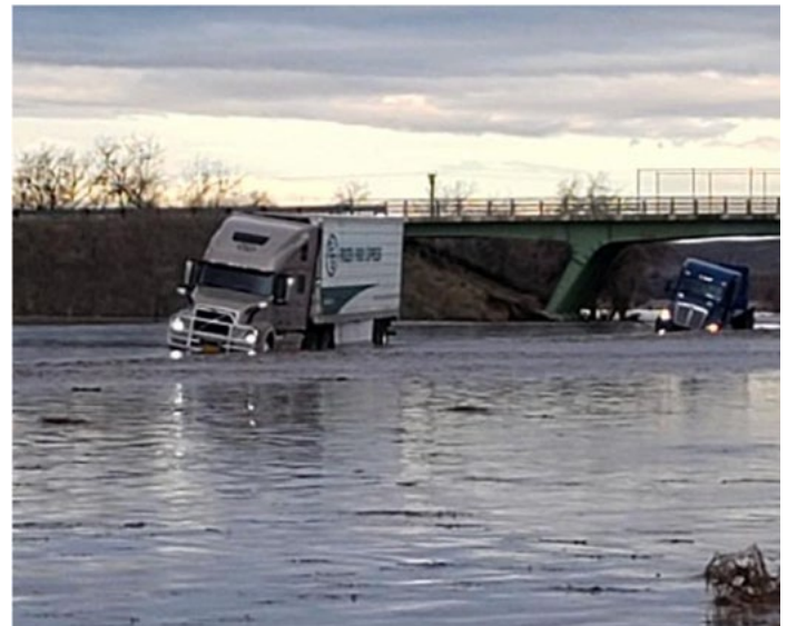
Figure 14. Interstate 84 near Echo, Oregon during the 2020 high flow event from the Umatilla River. (Photograph courtesy of Oregon Office of Emergency Management, all rights reserved)
