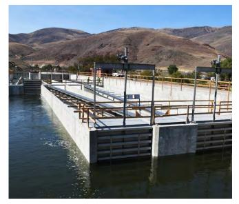
New horizontal fish screens at Derby Dam. The dam is part of Reclamation's Newlands Project and is 115 years old. It was one of the first Reclamation projects approved for construction and is part of a system that provides water to 57,000 acres of cropland in the Lahontan Valley in western Nevada.
