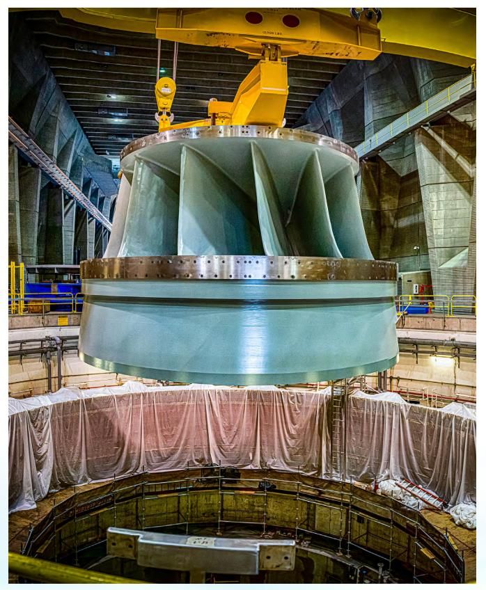
At the Nathaniel Washington Power Plant, a crane lowers a new turbine runner into Generating Unit 22 on June 12, 2020. This powerplant is a feature at Grand Coulee Dam, Columbia Basin Project in Washington State.
