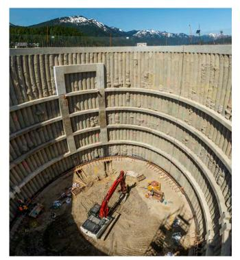
Panoramic view of the secant at Cle Elum Dam, Washington State. The secant is a very large ovalshaped hole that is stabilized by a concrete wall. It was built in preparation to construct the helix fish passage structure.
