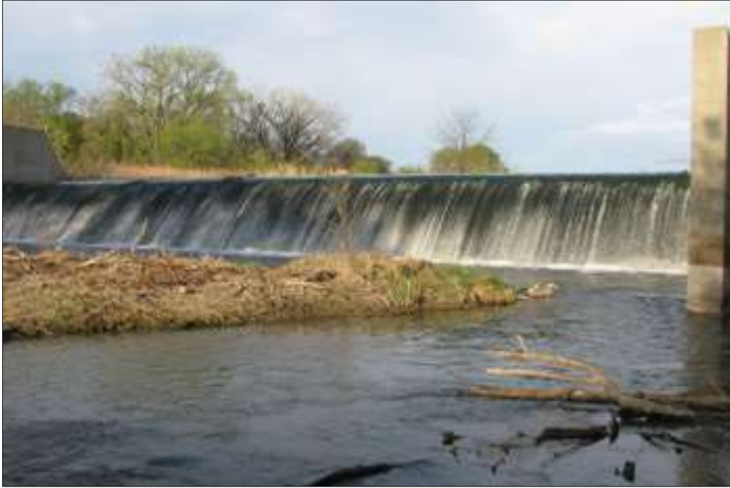
Figure 6–5. St. Mary Diversion Dam, Montana.
