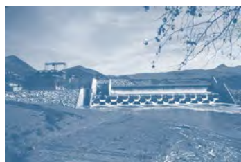
Marble Bluff Dam
