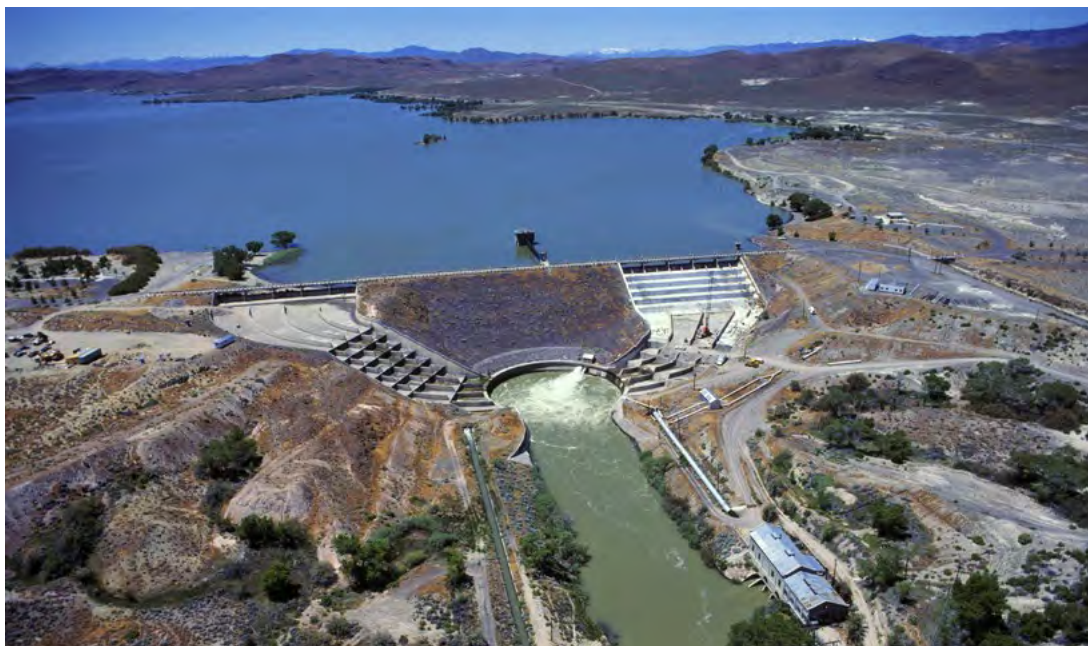
Figure 16. Lahontan Dam in Nevada, completed in 1915, is a zoned earthfill structure. The reservoir has a storage capacity of 289,700 acre-feet. Old Lahontan Powerplant, immediately below Lahontan Dam, has a capacity of 42,000 kilowatts.
