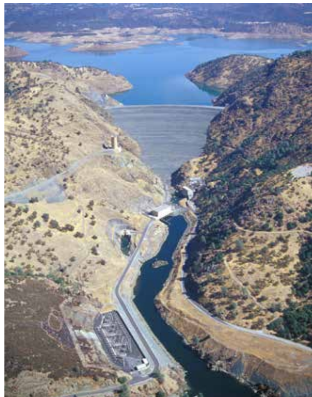
Figure 13. Aerial view of New Melones Dam, a rockfill dam 40 miles east of Stockton, California on the Stanislaus River.
