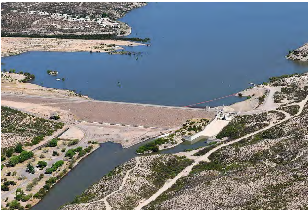
Figure 24. Aerial view of Caballo Dam, New Mexico.
