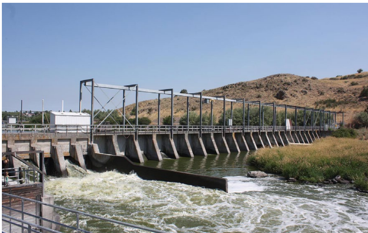
Figure 5. Link River Dam, west of Klamath Falls, Oregon, regulates elevations within Upper Klamath Lake and flow from the reservoir into the Klamath River. This reservoir is the principal source of water for the Klamath Project.
