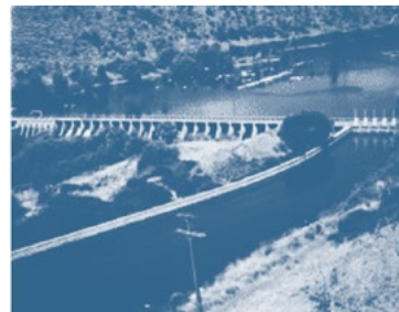
Link River Dam
