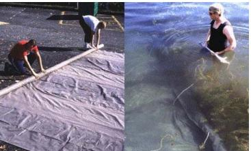
Figure 30. Installing bottom barriers.
