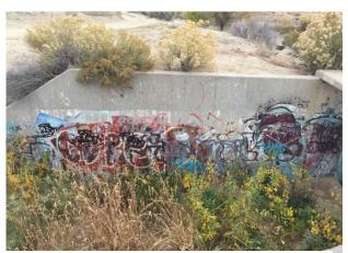
Figure 8. Weeds in a wasteway blocking emergency flows.
