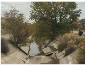
Figure 3. Extensive damage from trees on a concrete-lined canal.
