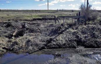
Figure 1. The vegetation in this canal prism is overgrown.
