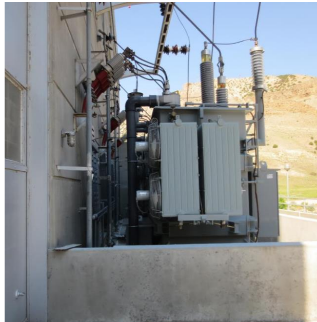
Figure 38. Side view of a transformer, looking at the transformer cooling fans.
