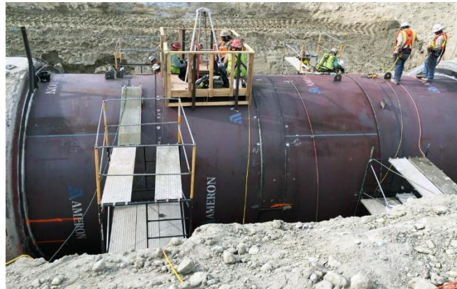
Figure 39. Example of confined space work (inside the pipe). Attendants outside the pipe can hoist people from a confined space but they cannot enter.
