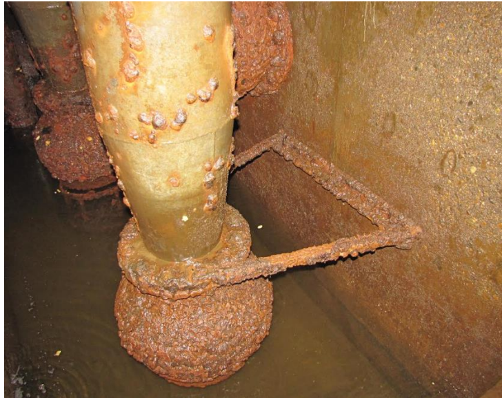
Figure 21. Corrosion can cause water flow issues or other operational problems.
