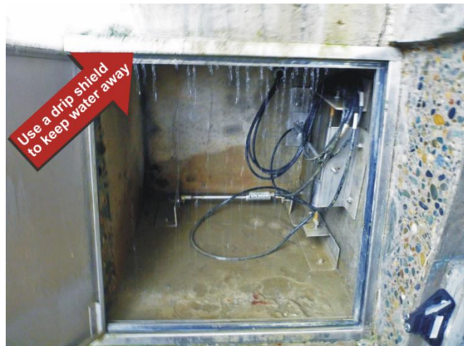
Figure 30. This enclosure has water dripping into it and puddles, making the equipment wet. This enclosure needs a drip shield to divert water running down the wall and door gasketing.
