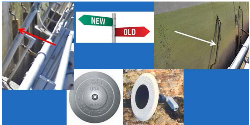
Figure 5. Replace GACP anodes.
