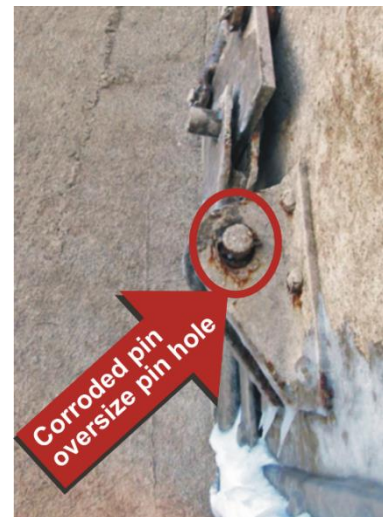
Figure 10. Corroded cotter pins and oversized pin holes from wear.
