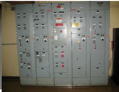
Figure 36. Motor starters in a motor control center.
