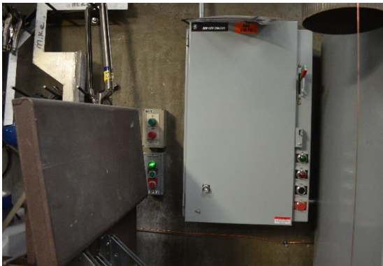
Figure 35. Loose starter.
