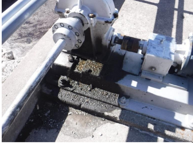
Figure 18. Leaking shaft seal on a gate hoist.
