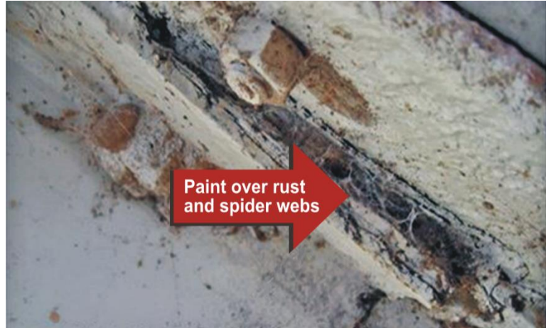
Figure 4. Properly prepare surfaces before coating. This includes cleaning such as abrasive blasting.
