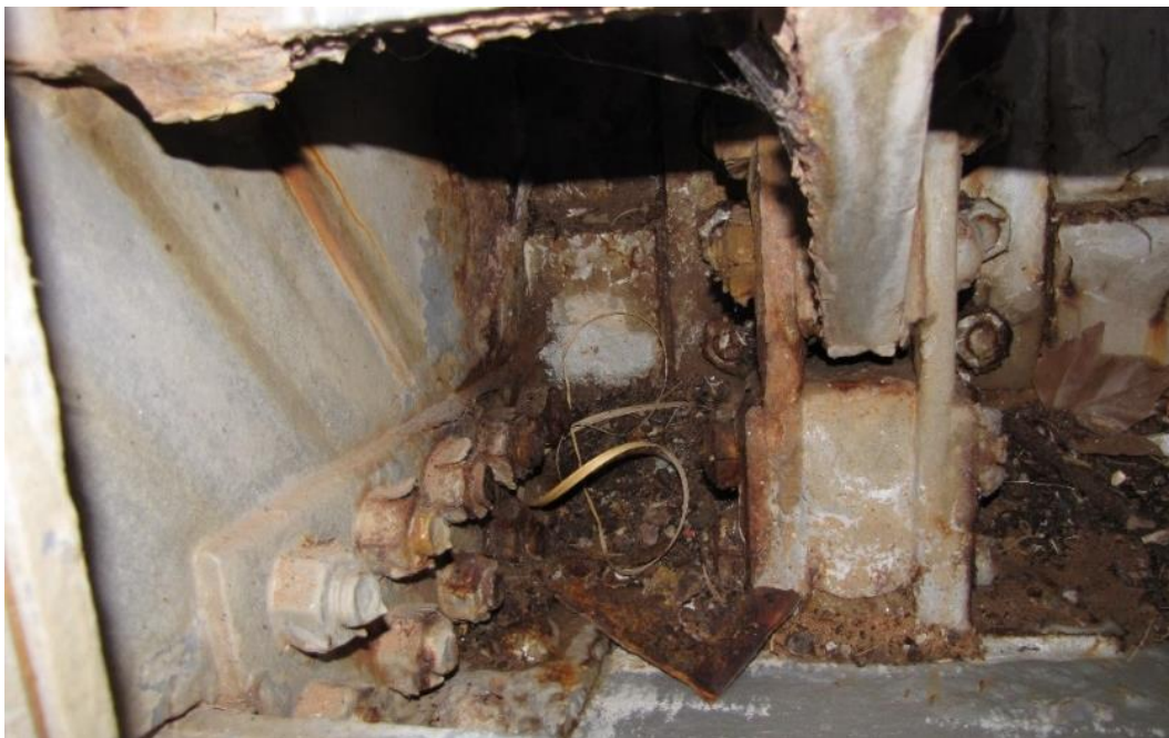
Figure 14. Typical damage on a radial gate (corroded rivets and debris build up due to periodic water intrusion).
