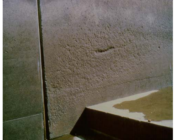
Figure 11. The early stages of concrete erosion and possible cavitation.
