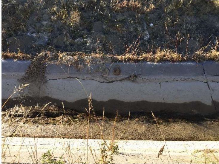
Figure 18. Hydrostatic pressure behind the lining ruptured the canal lining.
