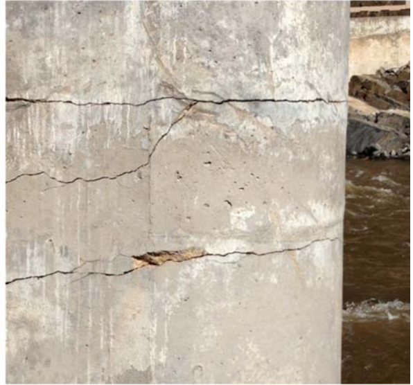
Figure 14. Structural damage from a collapsed roadway that impacted a support pier of a siphon. The road was undercut by flooding and then collapsed against the pier.
