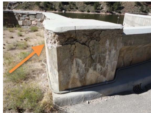
Figure 7. ASR deterioration.
