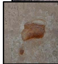
Figure 8. Corrosion of reinforcing steel.
