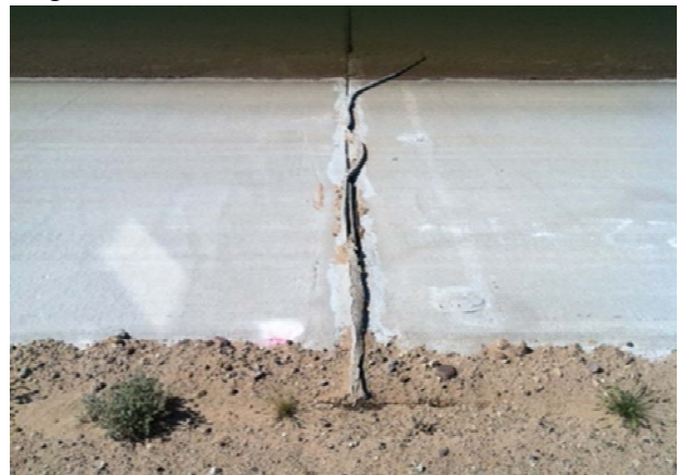
Figure 21. Buckling of canal lining where joint material is being squeezed out.
