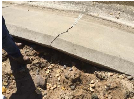
Figure 15. A crack in the canal allowed water to erode the soil beneath the liner.
