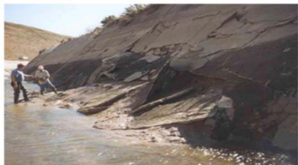
Figure 17. Subsidence of several canal linings.
