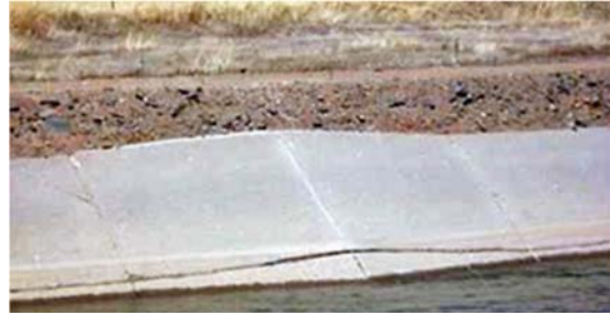
Figure 20. Uplift of the concrete lining.
