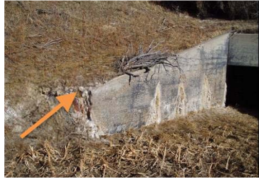
Figure 6. Sulfate attack on a canal structure.
