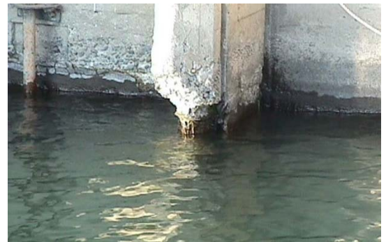
Figure 13. Freeze-thaw damage that could have been reduced by changing the structure's operations.
