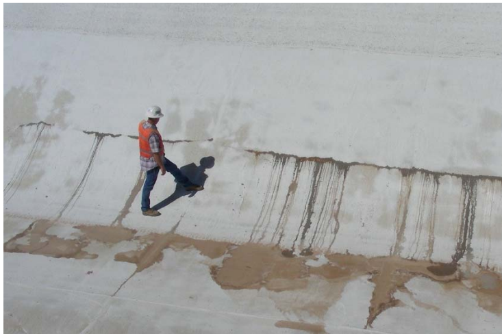
Figure 19. Hydrostatic pressure from ground water cracking a concrete canal lining.
