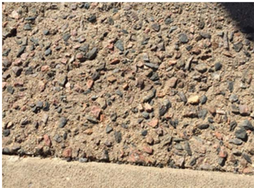
Figure 2. Paste washed from concrete exposed to flowing water before sufficient strength was achieved
