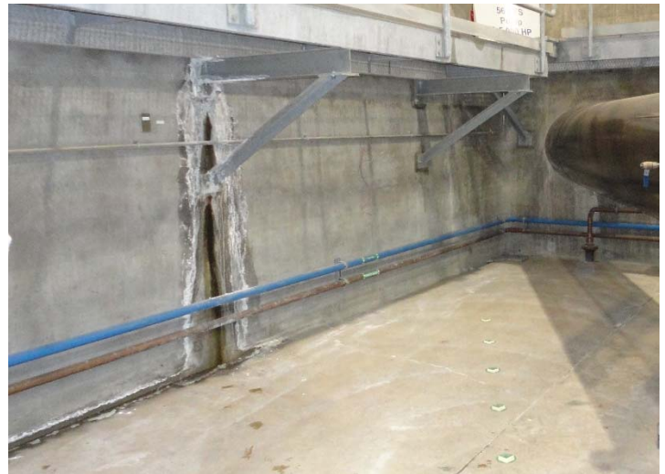
Figure 1. Thermal crack in a thick section of a concrete wall in a pumping plant. Ground water is leaking through the crack.
