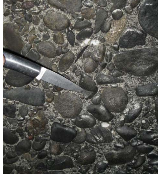
Figure 9. Abrasion-erosion of concrete surface leading to exposed and polished aggregate.
