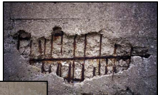
Figure 8. Corrosion of reinforcing steel.
