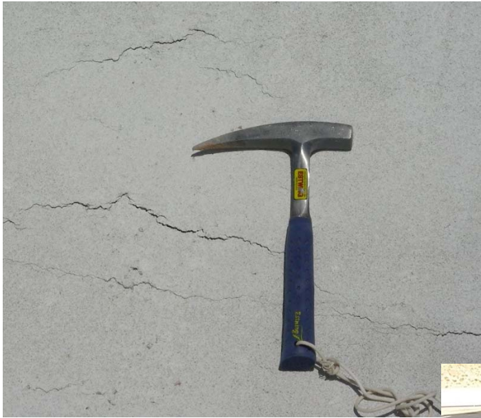
Figure 3. Plastic shrinkage cracking.
