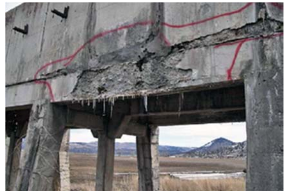
Figure 12. Freeze-thaw damage to concrete flume.
