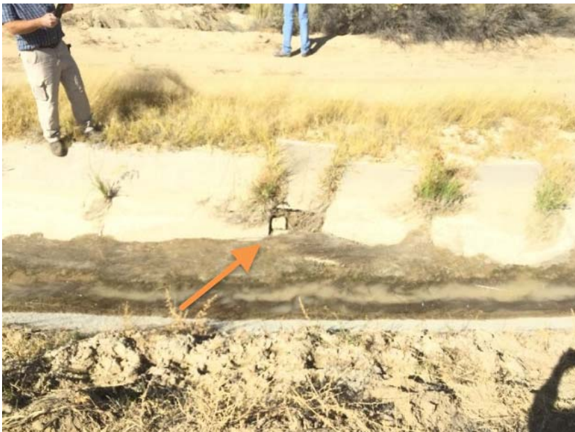
Figure 10. A front end loader damaged this concrete liner.
