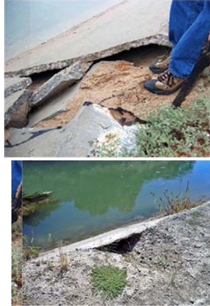
Figure 16. Voids under canal linings.
