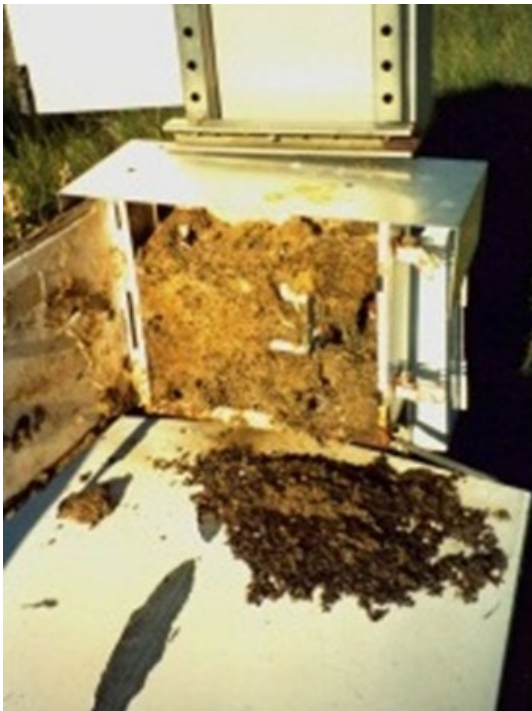
Figure 41. Junction boxes discovered containing a nest of grass and a wasp nest.
