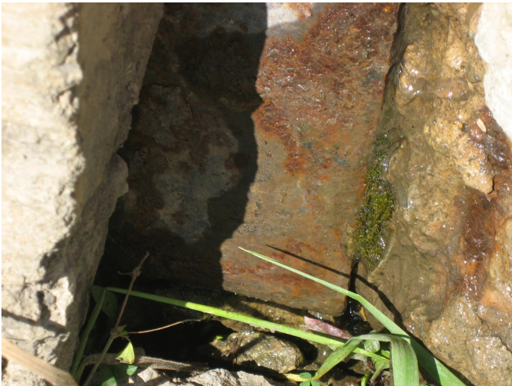
Figure 9. Pitting and surface corrosion of a metal strip between concrete box canal sections. Corrosion has led to increased seepage from the canal.
