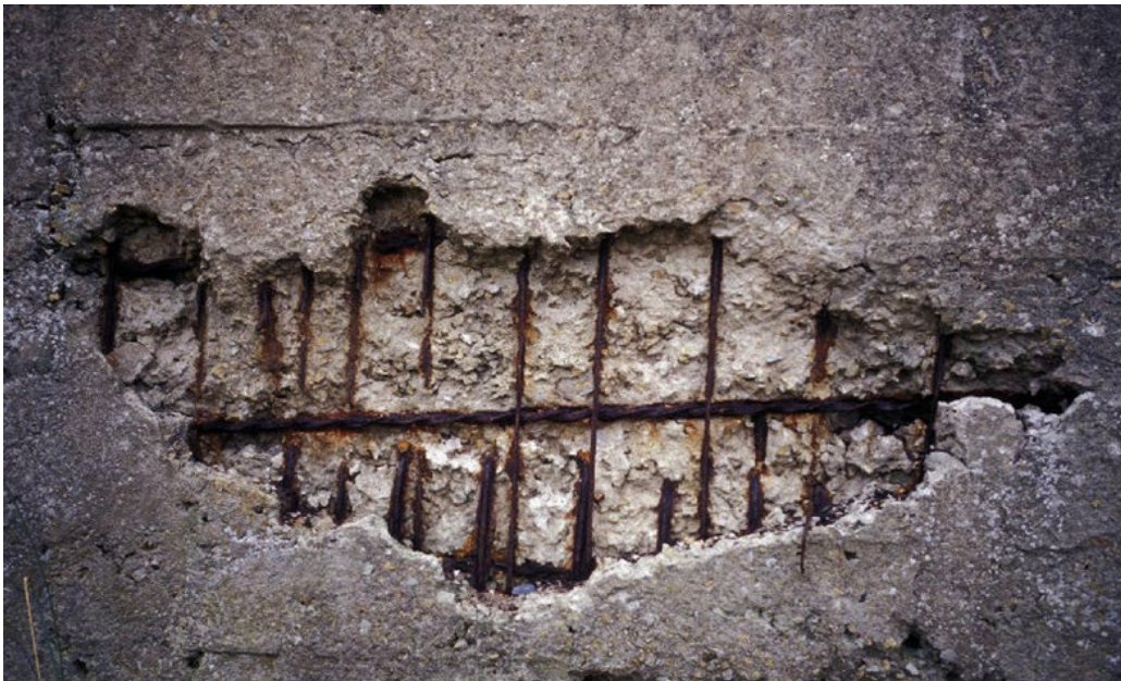
Figure 10. Corrosion of steel reinforcement in concrete, which led to spalling and further corrosion of the reinforcement.
