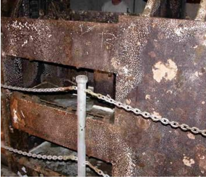
Figure 49. Galvanic anodes were not replaced after they were expended—resulting in extensive corrosion damage.
