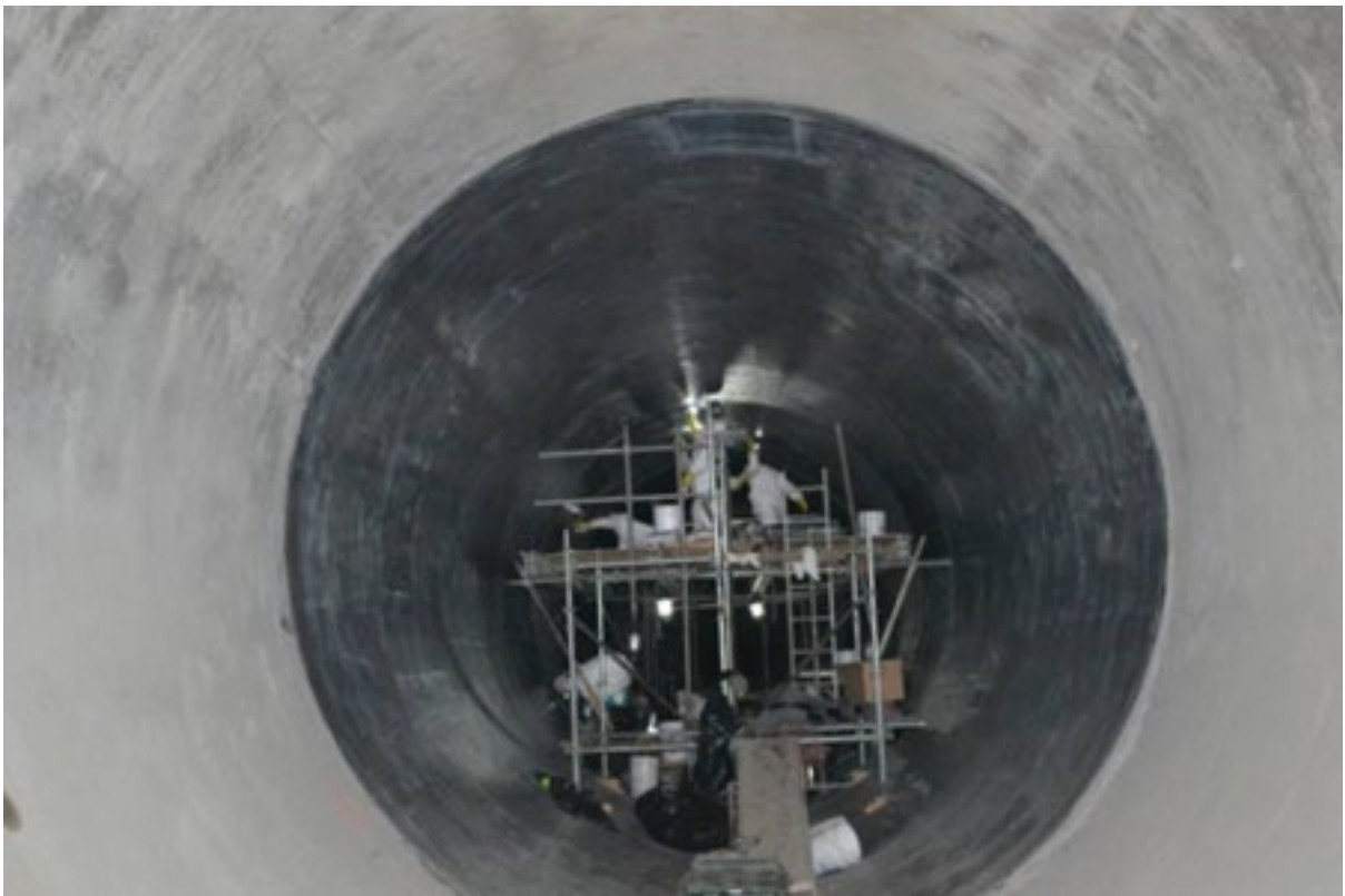
Figure 19. Completed CFRP lined 25-foot section of a 14-foot 8-inch diameter cast-in-place reinforced concrete pipe.
