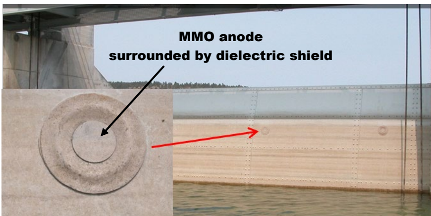
Figure 28. Surface mounted mixed-metal oxide (MMO) disk anode with a dielectric shield for impressed current CP for a radial gate.
