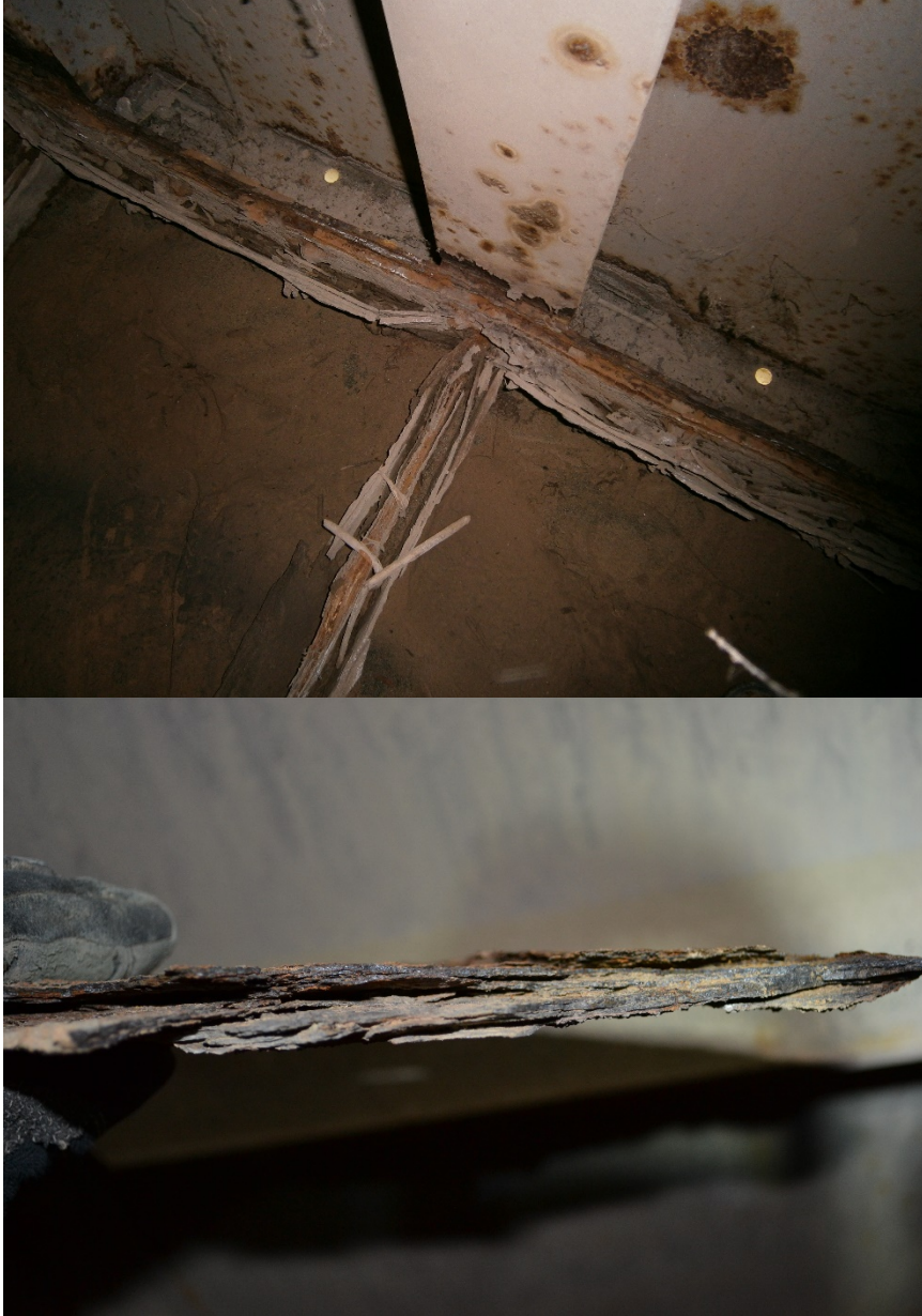
Figure 7. Interior stiffener inside radial gate compartment. Corrosion occurred between the two plates, causing extreme crevice corrosion and eventual exfoliation of the steel stiffeners.
