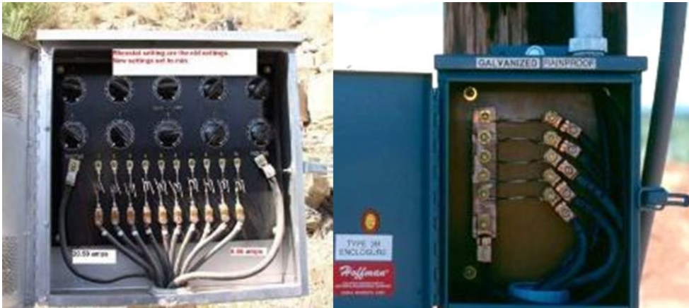
Figure 37. Two anode junction boxes. Both have shunts; however, the one on the left also includes variable resistors.
