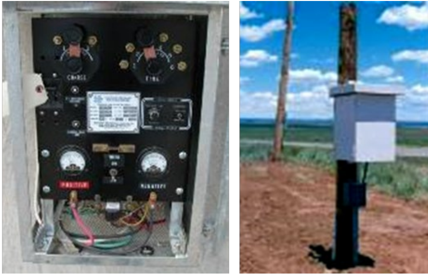
Figure 39. Rectifier for ICCP system on buried pipeline. The photo on the left shows the front panel of a rectifier. The photo on the right is a photo of the rectifier cabinet.
