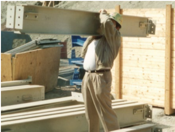
Figure 14. An FRP structural beam is lighter than a steel beam (Strongwell Corporation, all rights reserved).
