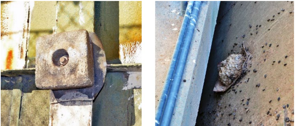
Figure 47. Nearly new hull anode is shown on the left while a depleted anode is on the right. Note the lack of corrosion around the anode on the right.
