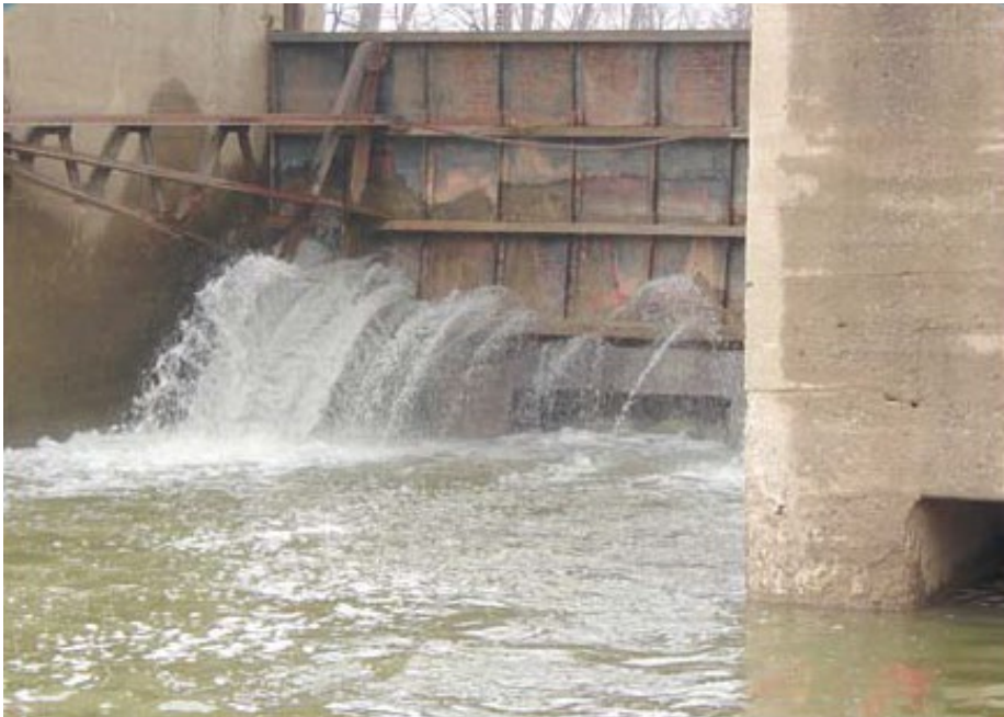
Figure 12. Damage to a radial gate caused by corrosion leading to uncontrolled leakage.
