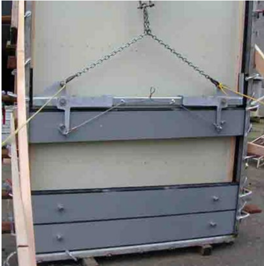
Figure 17. FRP stoplogs. (Plasti-Fab, nd, all rights reserved).
