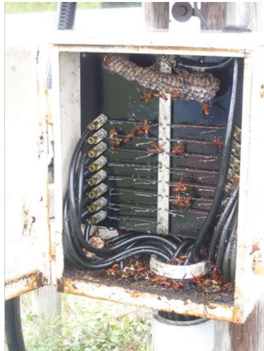
Figure 41. Junction boxes discovered containing a nest of grass and a wasp nest.
