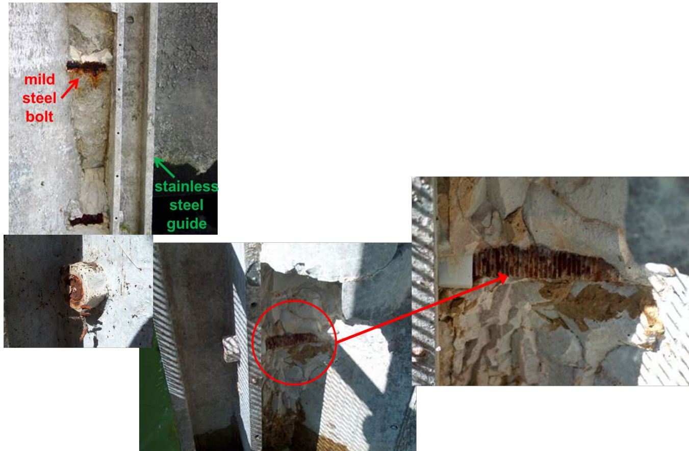
Figure 5. Galvanic corrosion of mild steel anchor bolts in contact with stainless steel guides. Regardless of the grout provided, the effect of the galvanic couple is causing corrosion of the anchor bolts.
