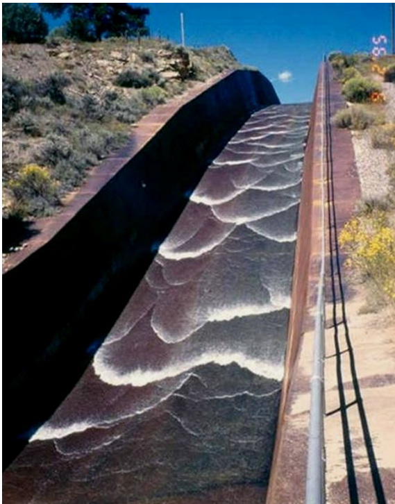
Figure 4. Example of uniform corrosion (rust along the floor and walls) of a steel spillway.
