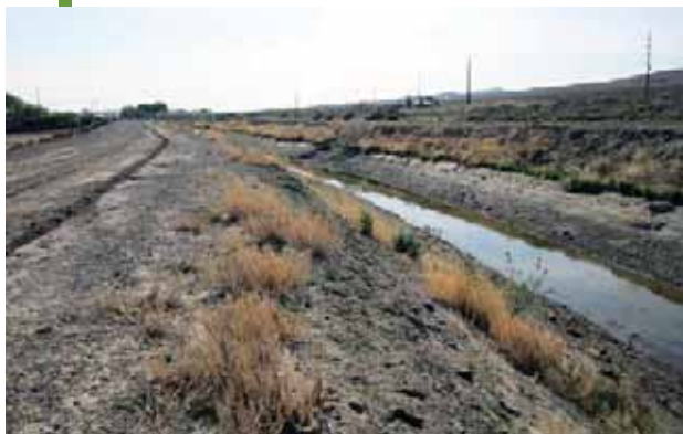
Windrow from the pass of a motor grader.
