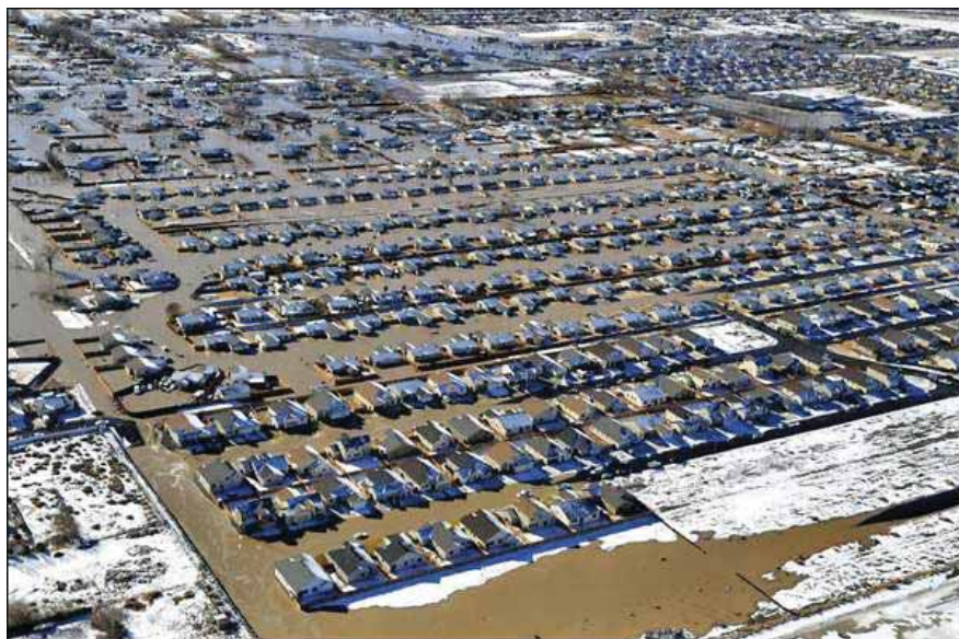
Flooding from a breach in a Reclamation canal embankment.
