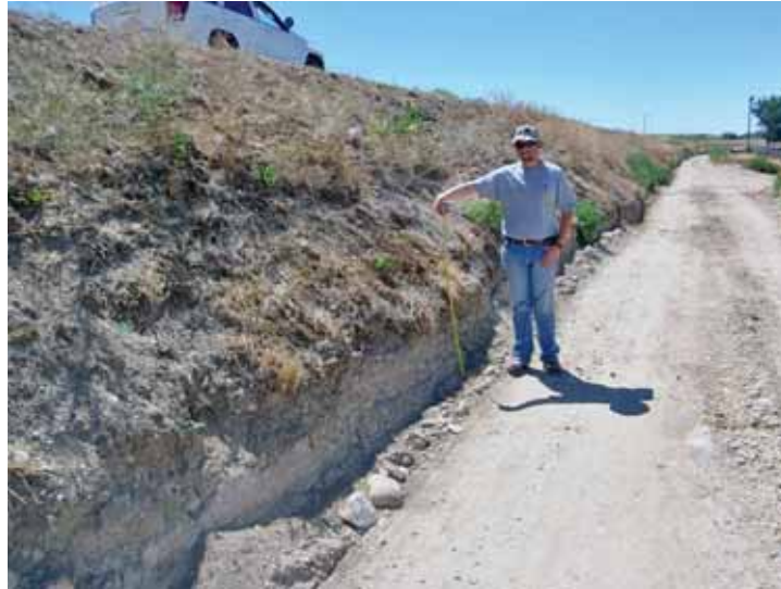
This road was built so close to the embankment that they cut off the toe of the canal embankment.
