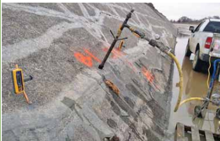
Pressure grouting to fill seepage paths behind the concrete lining.
