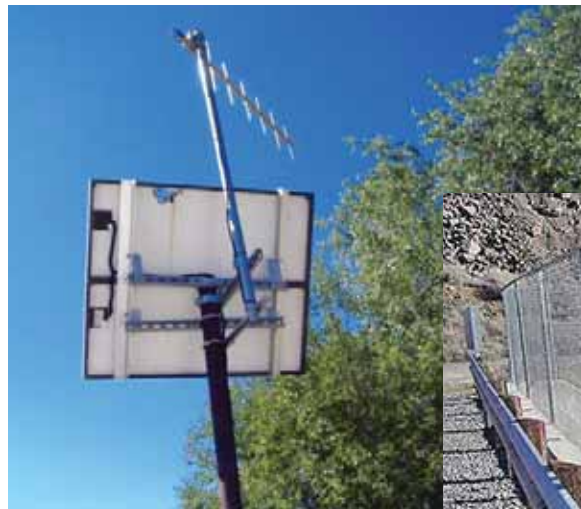
Vandalized solar panel.
