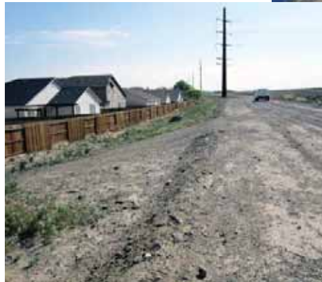
Power pole in the embankment slope and fence at the embankment toe.
