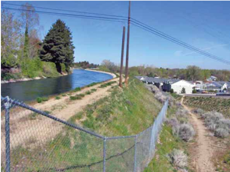
Typical Reclamation canal in an urbanized area.
