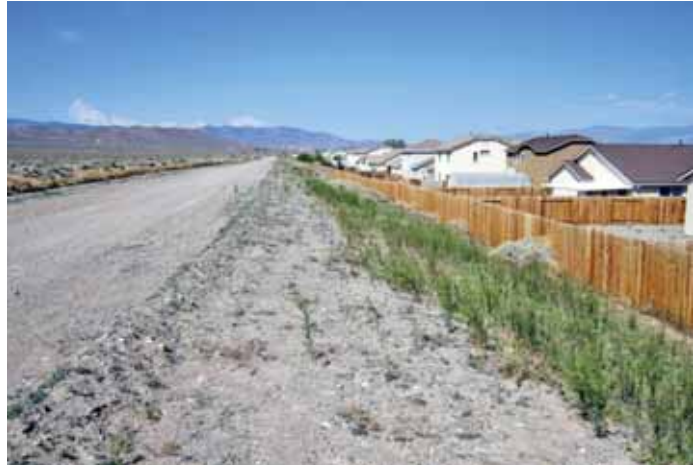
Fences close to the embankment toe do not allow enough room for you to perform O&M.
