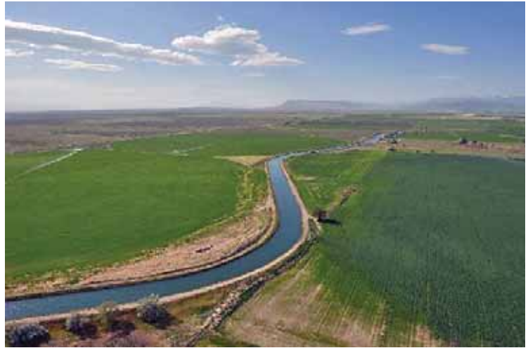
Typical Reclamation canal in a rural area.
