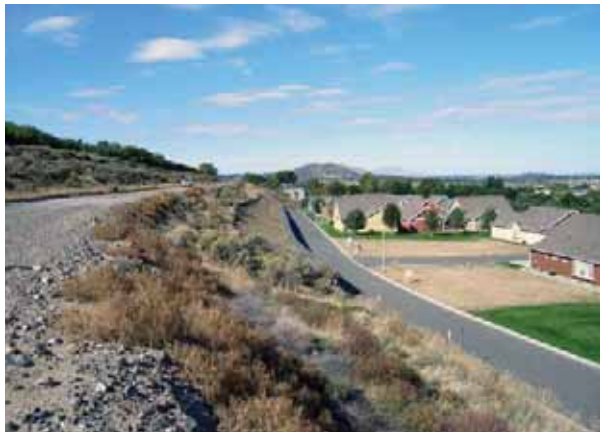
Development with retaining wall at embankment toe next to road.
