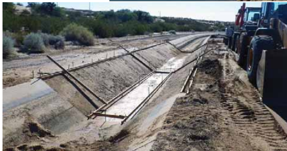
Replacing canal concrete lining.
