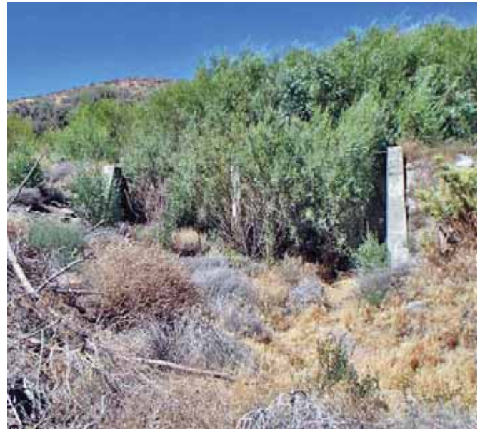
Canal undershot with plugged outlet.
