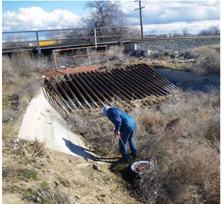
Clearing a trashrack.
