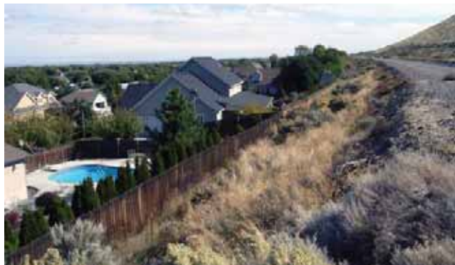
Swimming pool at the toe of a canal.
