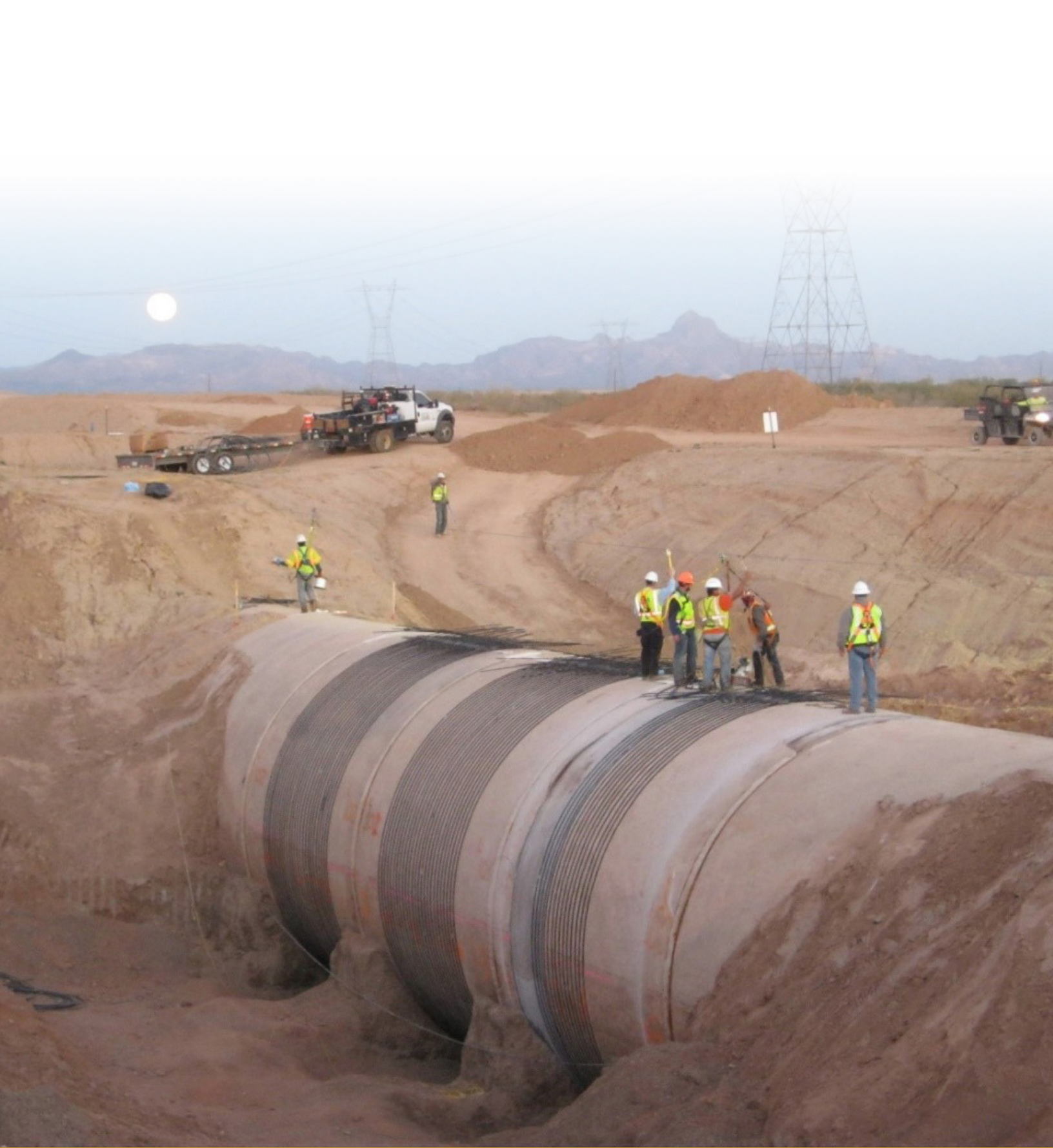
PCCP wrapping operations at Centennial Wash Siphon, Maricopa County, Arizona.
