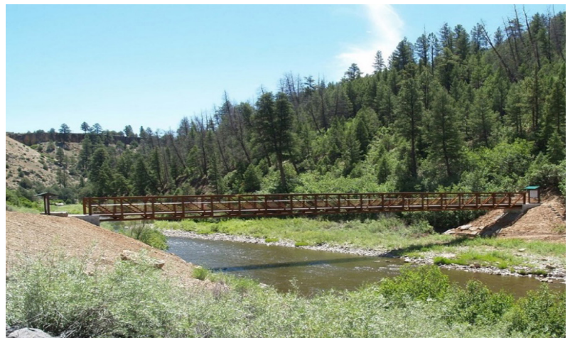
Completed Rio Chama Trail Bridge, Chama, New Mexico, a Federal Lands Transportation Program-funded project completed in summer 2022.
