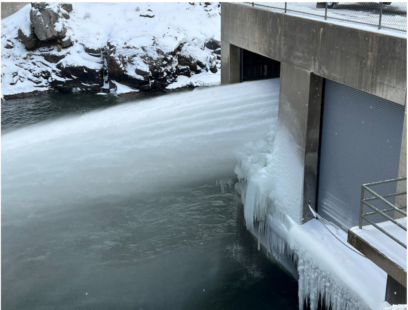
Bypassing water during Blue Mesa Powerplant (Colorado) outage in 2022.
