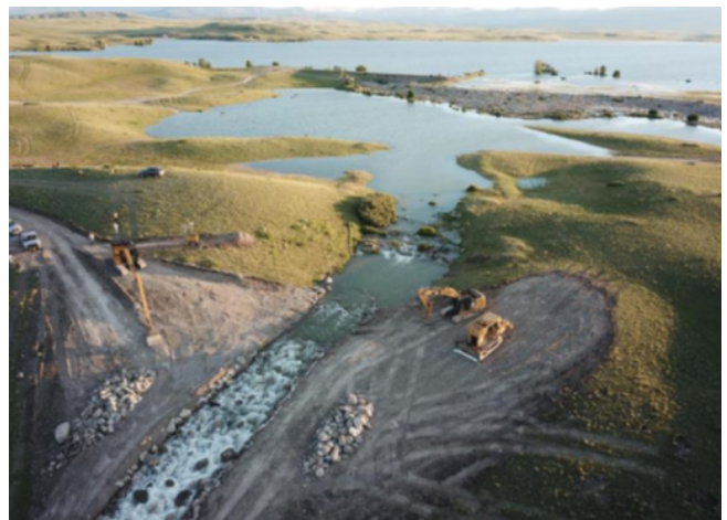
Aerial view of spillway flows at Willow Creek Dam in Montana. Flows over the earthen, uncontrolled spillway resulted in erosion and activation of the EAP.
