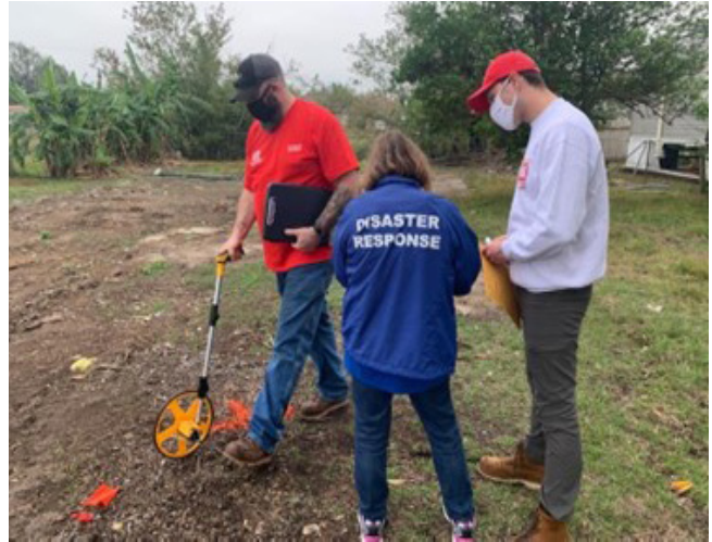
USACE and Reclamation deployers assess a hurricane-impacted property and measure the area for installation of temporary housing (Louisiana, 2021).
