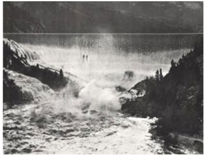
Gibson Dam overtopping during the June 1964 flood.
