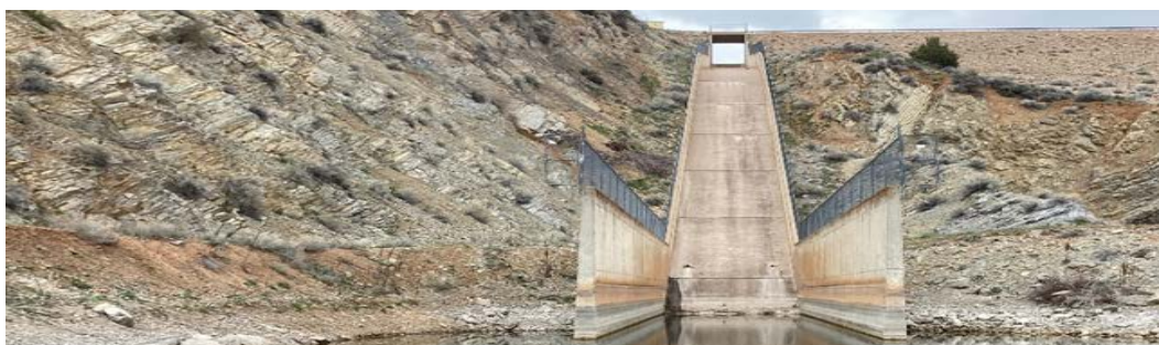
Spillway chute at Lost Creek Dam in Utah – 2022 Comprehensive Review Exam.
