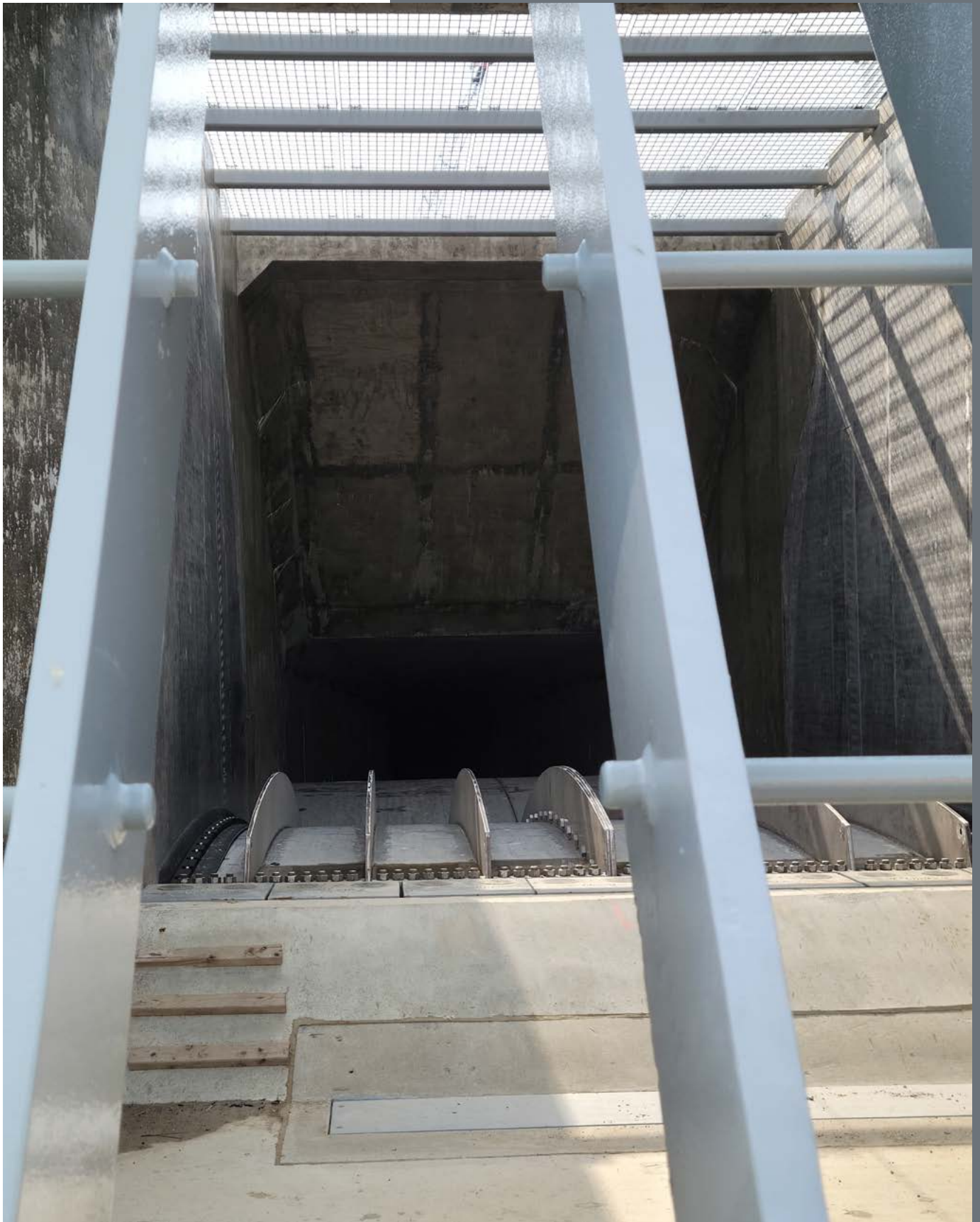
Fish Passage Facility, Cle Elum Dam, Yakima Project, Washington, as seen at the April 2023 Review of Operation and Maintenance Workshop.
