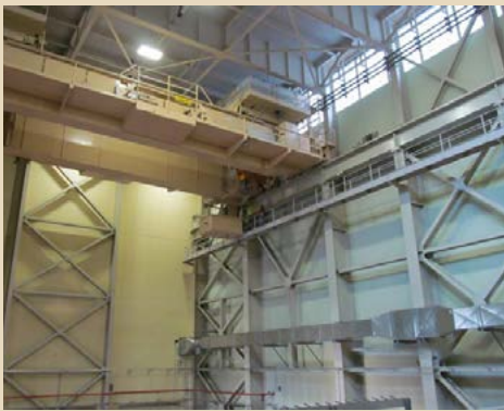
Palisades Dam Powerplant, Bonneville County, Idaho.
