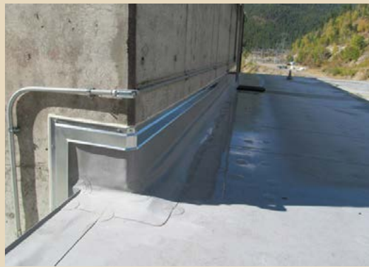
Hungry Horse Dam Powerplant Roof, Flathead County, Montana.
