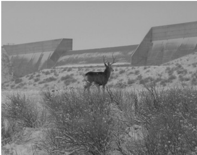
Pueblo Dam, part of the Fryingpan-Arkansas Project, is in the background, while a buck poses in the snow in the foreground.
