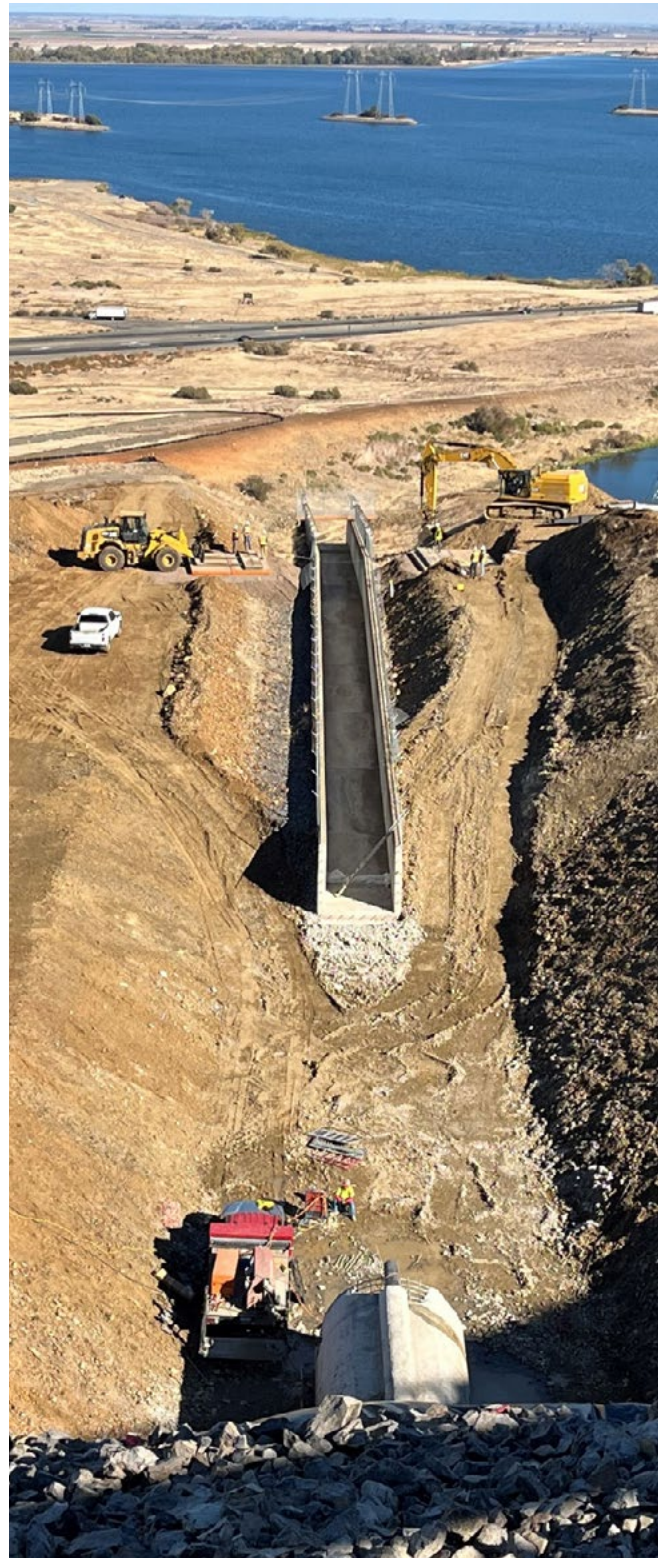
Spillway demolition and foundation preparation.
