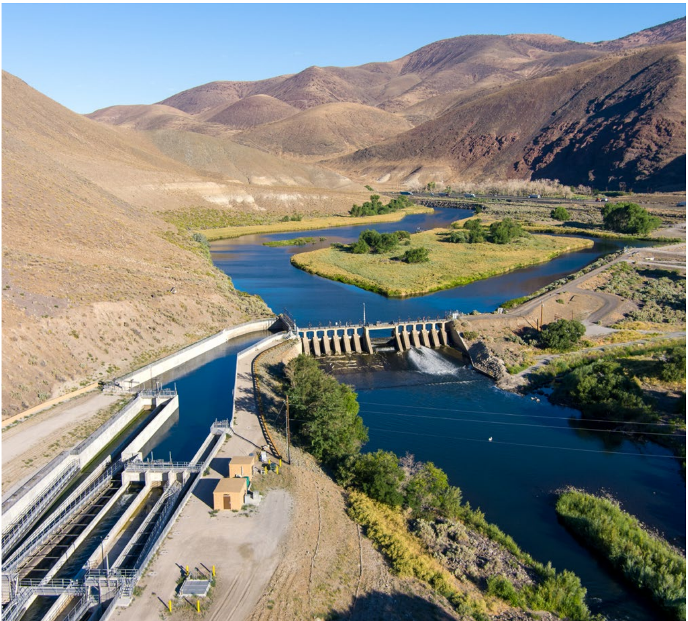
Truckee Canal at the Derby Diversion Dam, Newlands Project, Nevada.
