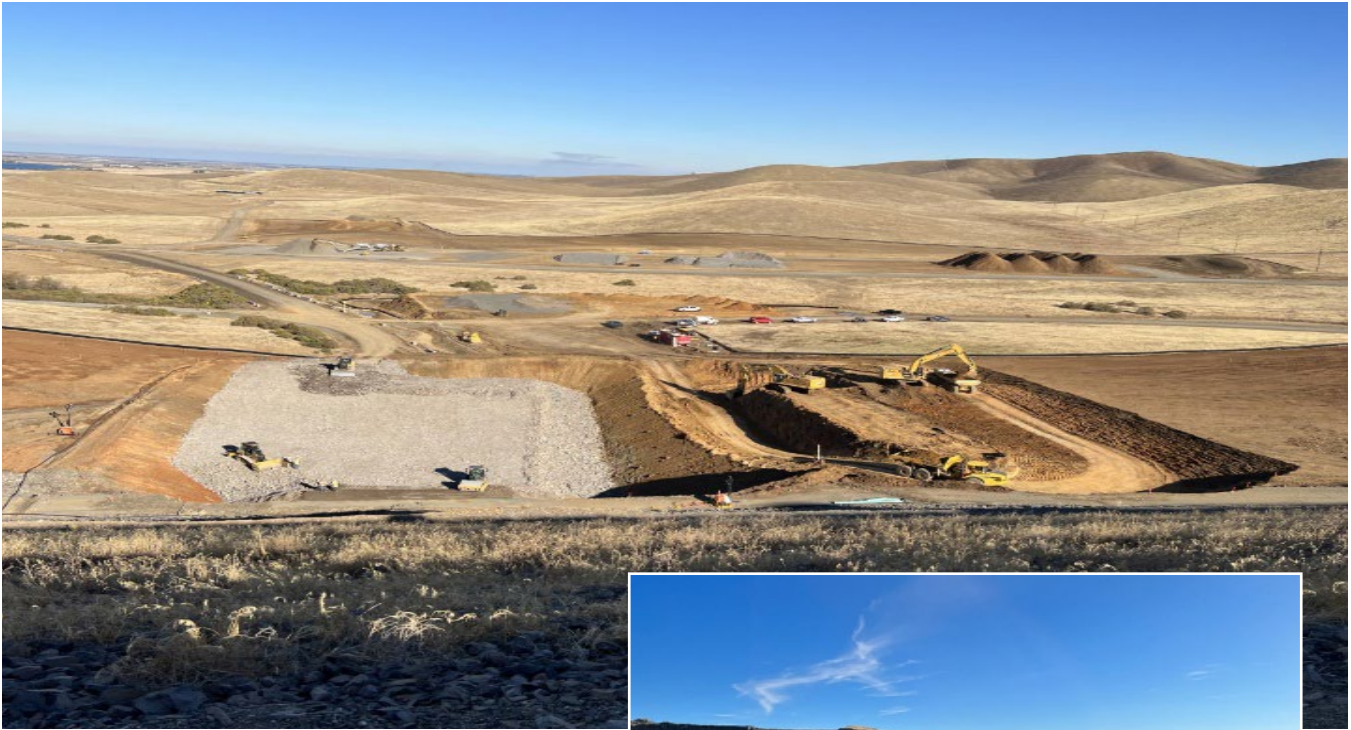
Construction of shear keys, part of the first contract scope.
