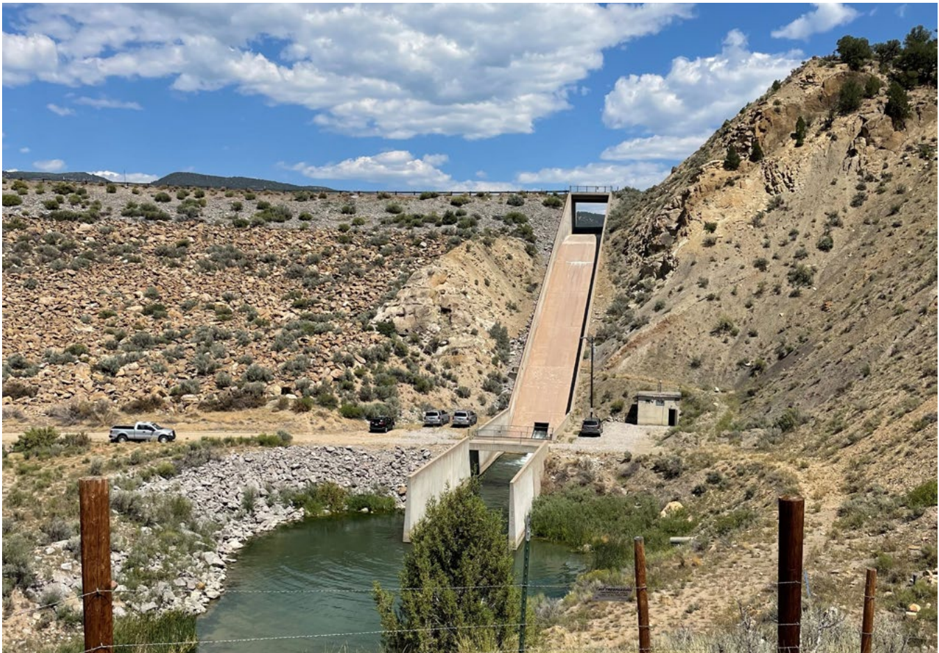
Rifle Gap Dam, part of the Silt Project, in Rifle, Colorado.
