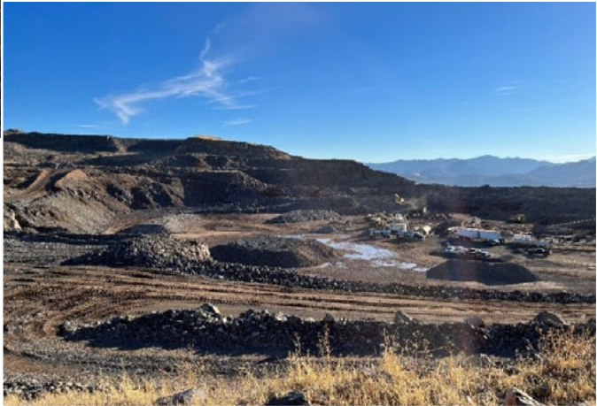
Basalt Hill Quarry – material processing.
