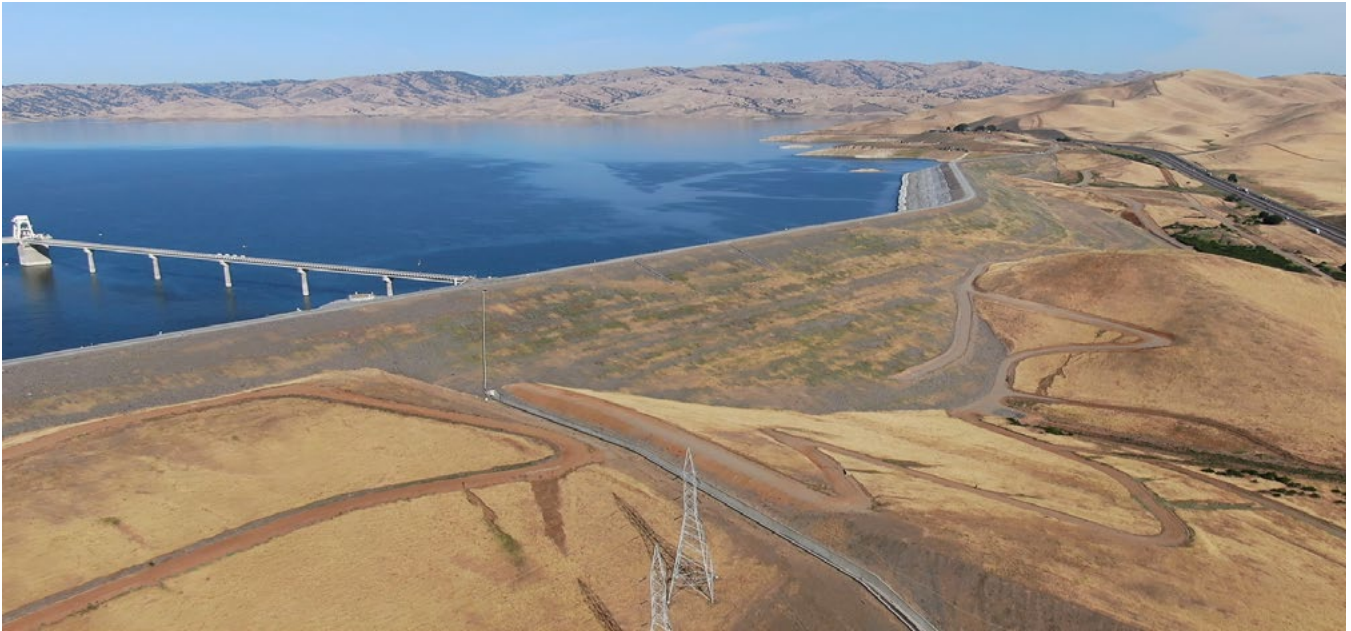
B.F. Sisk Dam, spillway (center), and bridge to outlet works intake structures. Screen capture from aerial footage captured by Dudek in Summer 2020.
