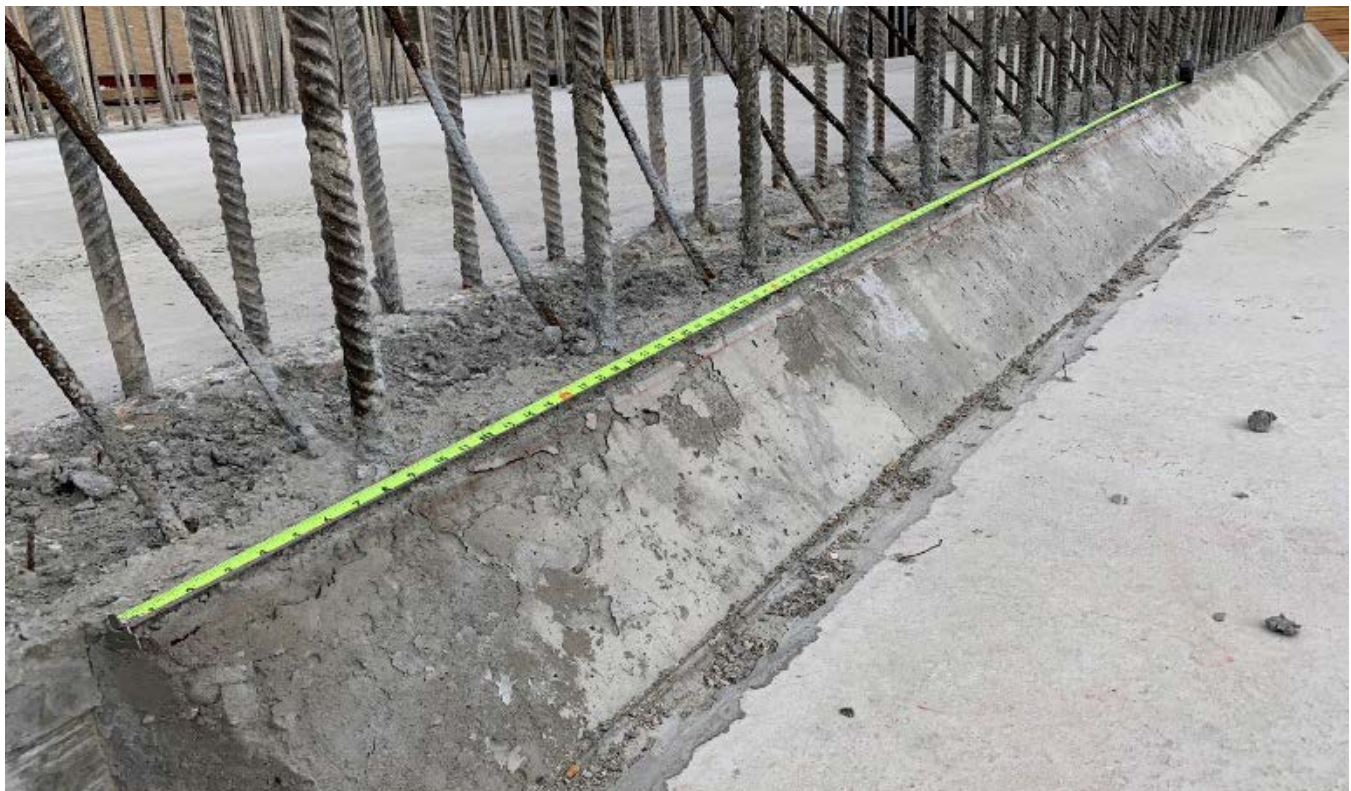
Slaking and scaling on formed concrete surface due to hot air blowing directly on the forms, which dried out the concrete underneath.
