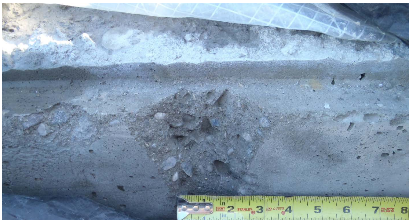
Damage due to early age freezing. Top surface was tented and heated. Freezing is localized to form panel seams and exterior upper edges of block.
