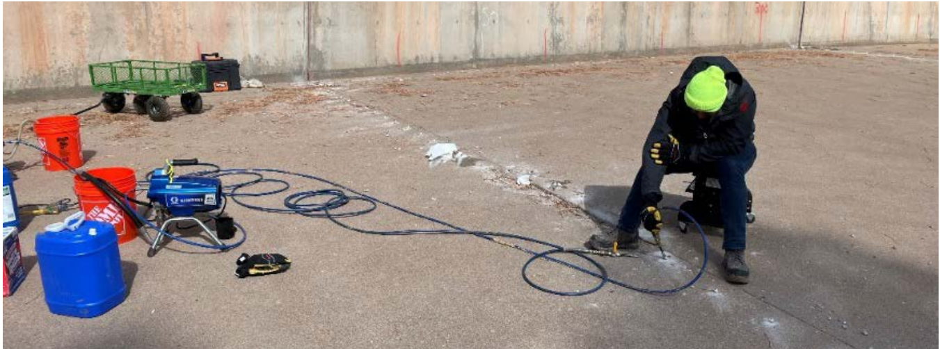
Chemical grout injection in a spillway contraction joint at Vallecito Dam to prevent water inflow leading to uplift pressure.
