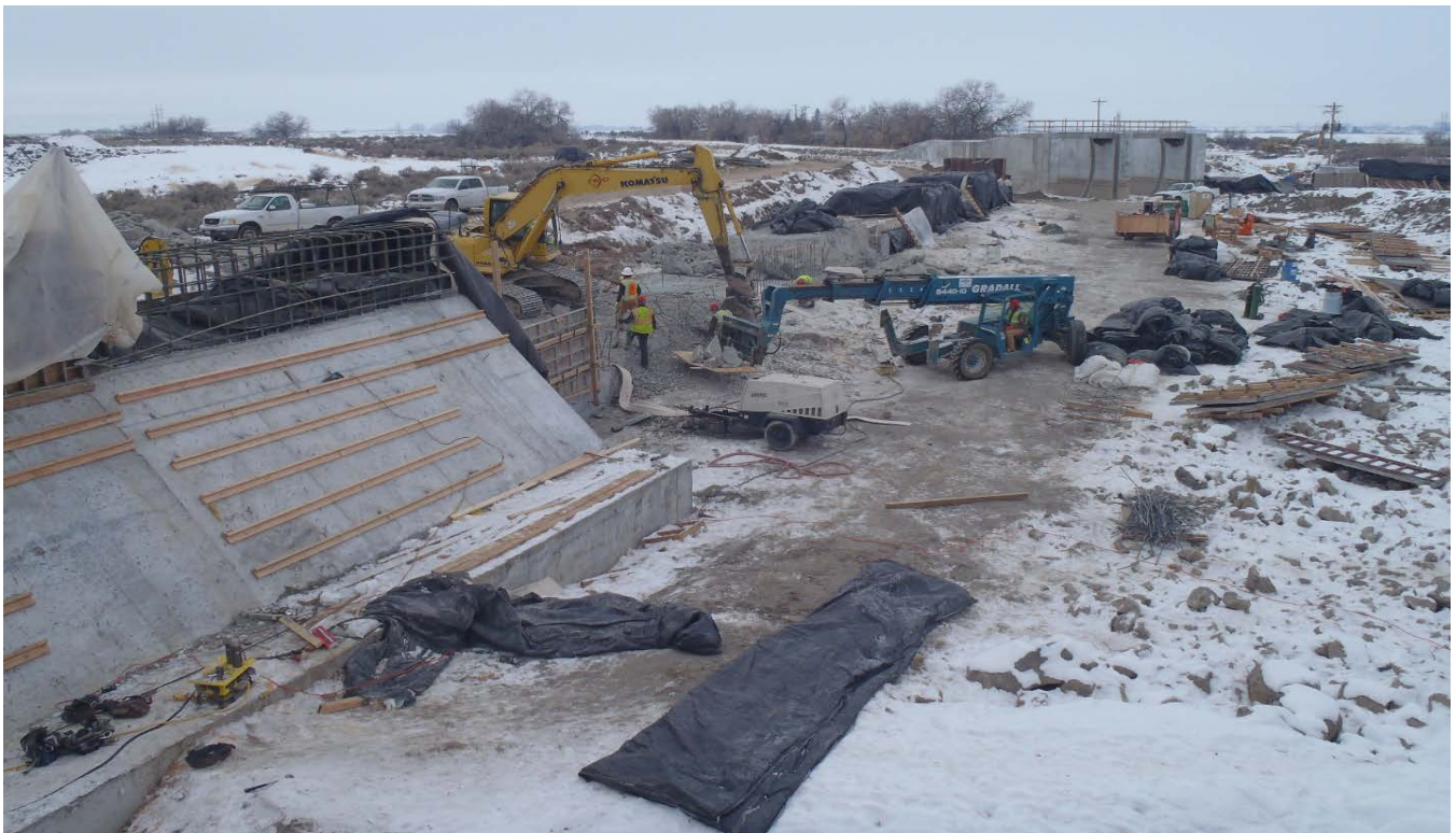
Frozen concrete being removed by excavator after improper early age protection.
