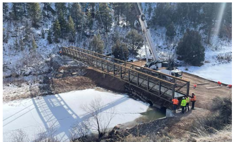
New bridge being lifted into place and set on the abutments.
