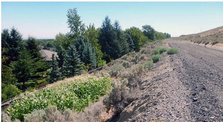
Building or growing crops on a canal right-of-way is a common type of encroachment.
