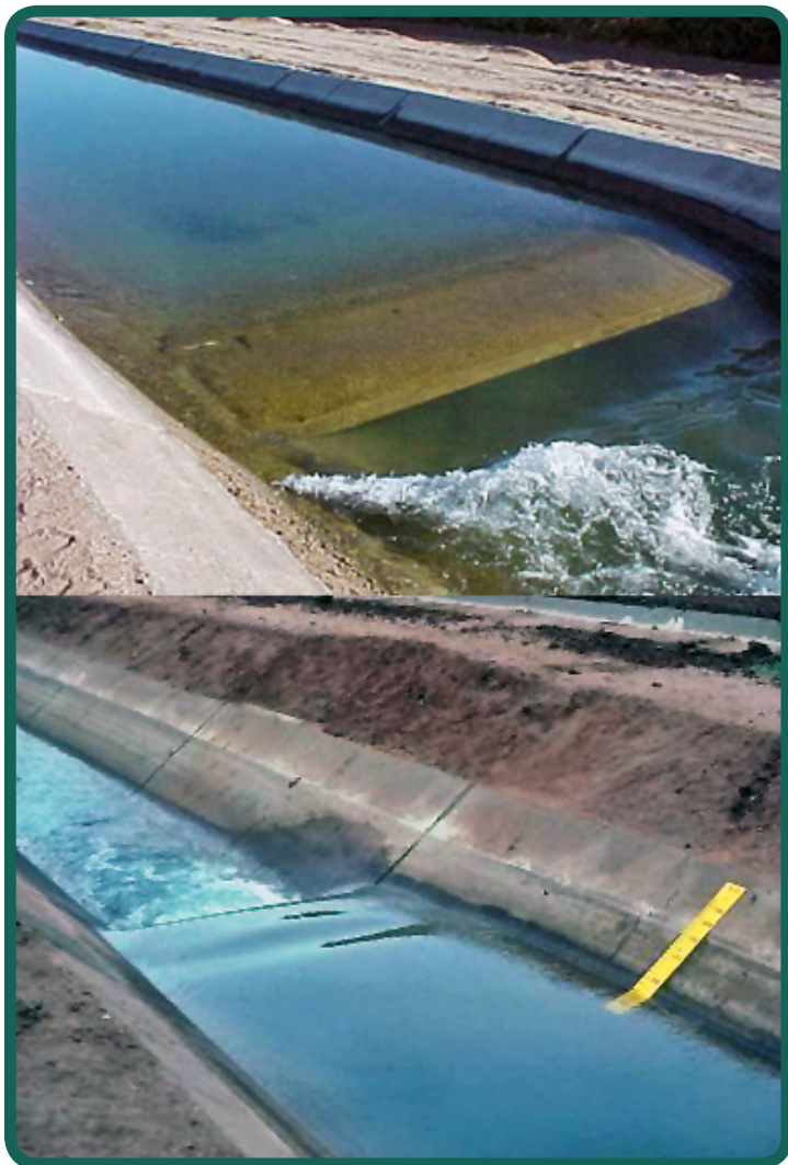
Less head is needed for broad-crested weirs and long-throated flumes.
