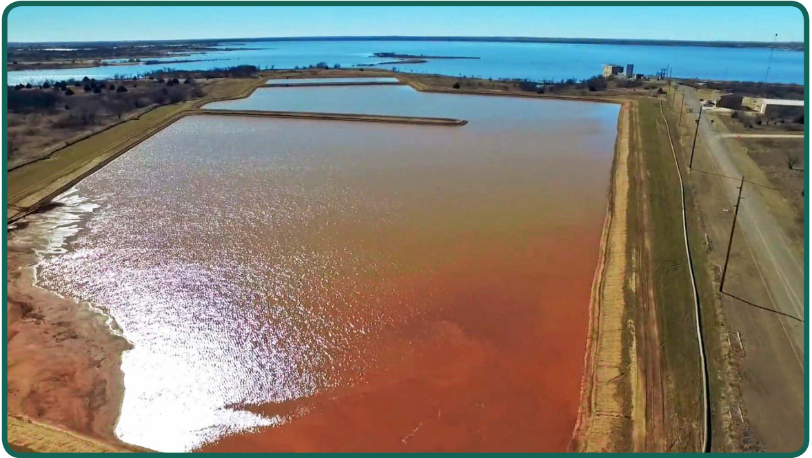
Drying out the dredged sediment in the confined material dredge storage area.
