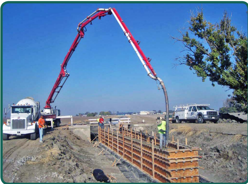
Constructing a long crested weir.
