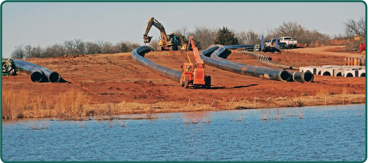
Assembling the five 800-foot-long section of 42-inch HDPE pipe that were combined in the lake intake channel.
