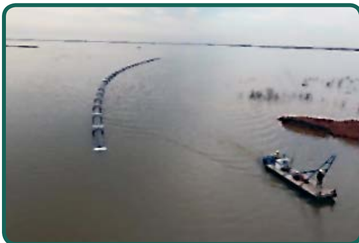
Lowering the pipe onto the bottom of the Waurika Lake underwater intake channel.
