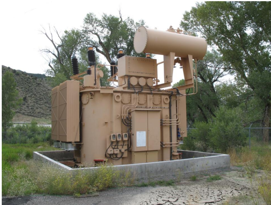
Figure 6.—Spare transformer located at the Curecanti Field Division, Colorado. Secondary containment is provided by a concrete wall around the transformer. Imbiber Beads® allow drainage of storm water, but swell upon contact with oil and prevent flow of oil out of the containment area.
