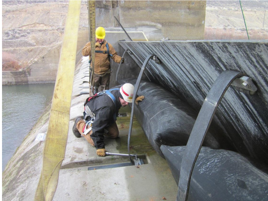
Figure 9.—Back side of gates, showing the gate bladders and restraining straps. In this photo, Government crews are checking bolt torques during the first maintenance season.
