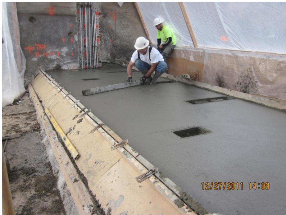
Figure 5.—Placement of concrete crest, imbedding the air lines.
