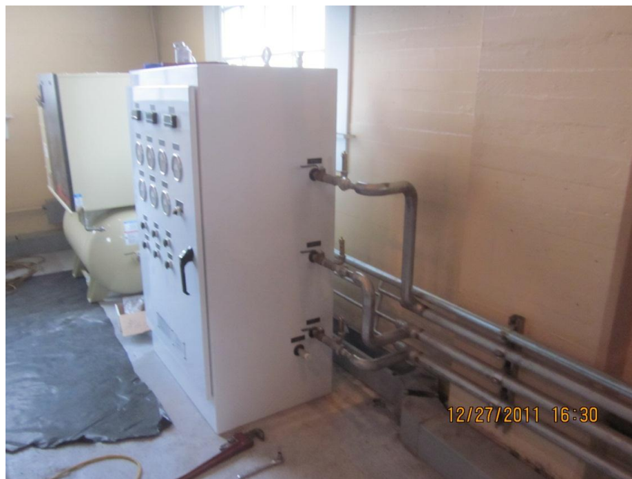
Figure 8.—Pneumatic control system for the Obermeyer gates, including the compressor and air receiver in rear, control cabinet, and stainless steel air piping, which is connected to the air bladders under the gates.
