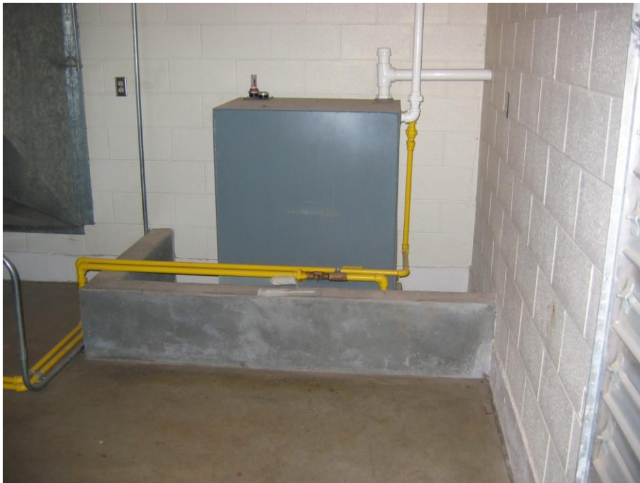
Figure 1.—Secondary containment around oil-containing equipment at Deer Creek Powerplant, Utah.
