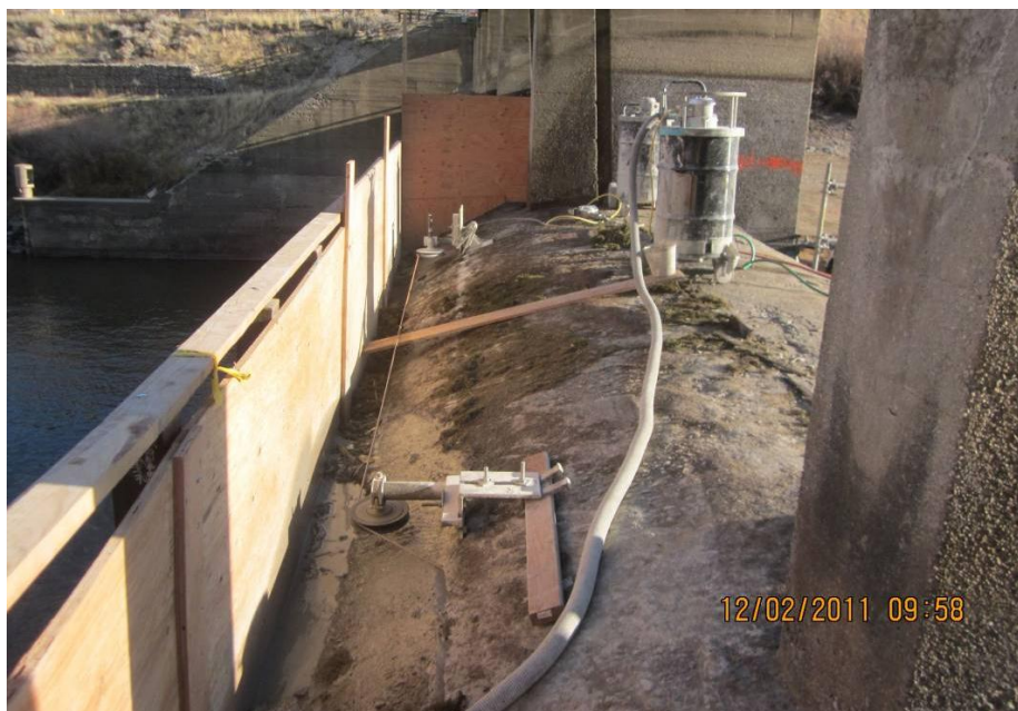
Figure 3.—Horizontal cable saw used to cut off the top of the original ogee spillway crest at Boise River Diversion Dam.
