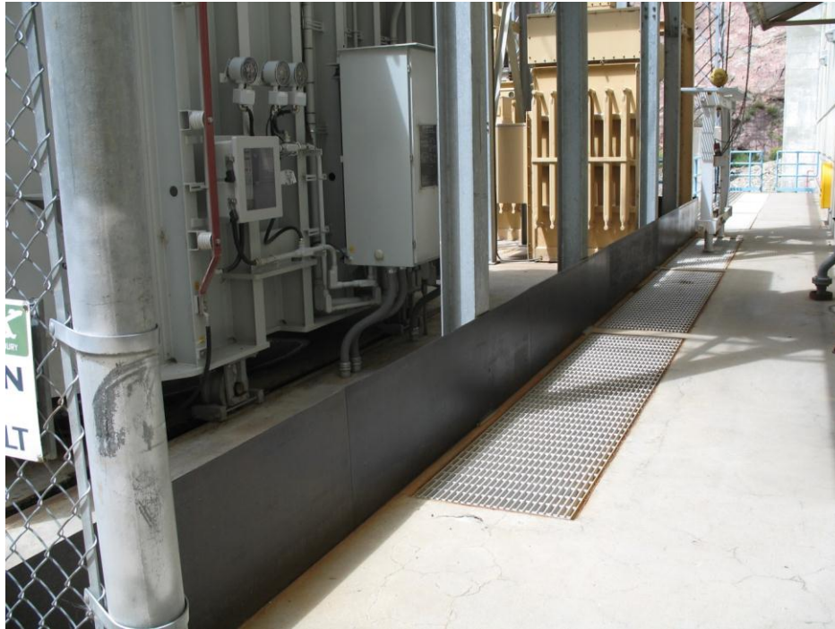
Figure 3.—Containment area around transformers at Blue Mesa Powerplant, Colorado.
