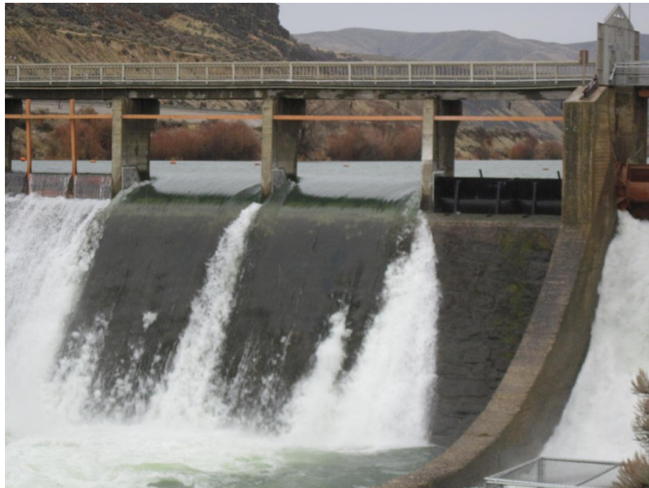
Figure 10.—Boise River discharge over Obermeyer gates 2 and 3, with the gate at the far right in the fully raised position. When the gates are fully raised, the leakage past the seals is drop-tight. The installed flashboards can be seen on the far left in bay 4.
