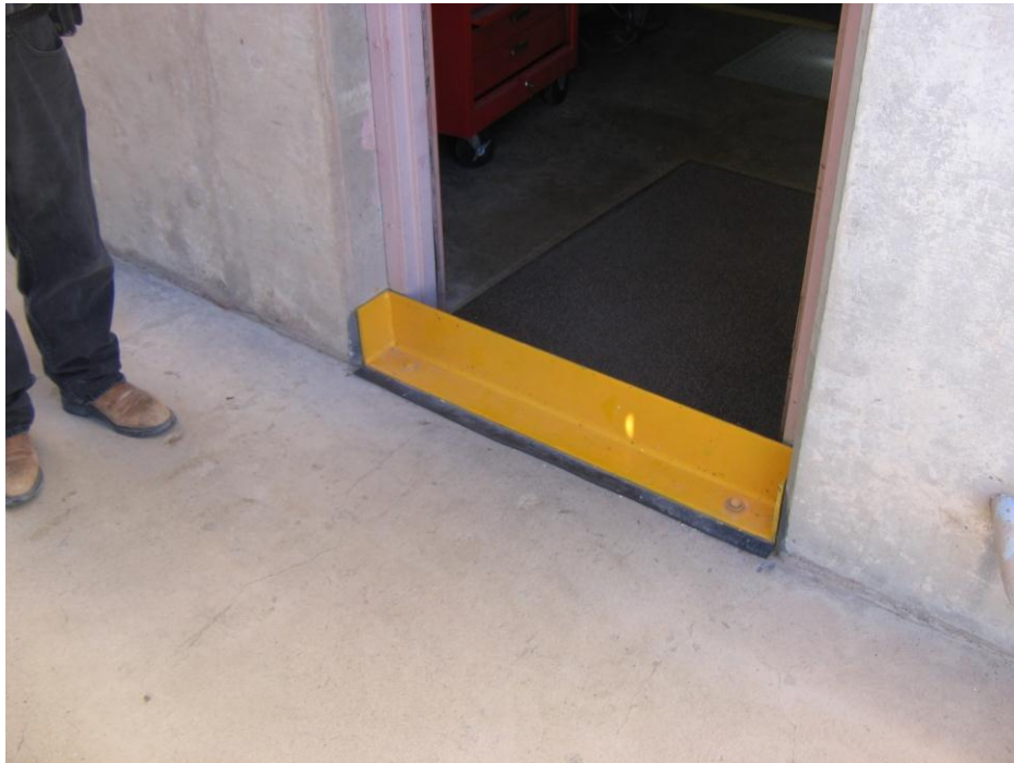
Figure 7.—A containment berm at Fontenelle Powerplant, Wyoming. The berm provides containment of oil, which in the event of a spill would otherwise flow under the door.
