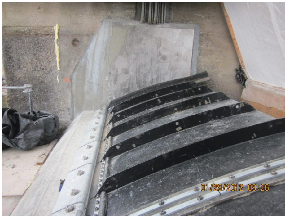
Figure 7.—Gate panels in place. Note, from left to right, the anchor clamp castings, with two anchor bolts each, the rubber hinge, and two steel gate panels, connected by a reinforced polyester inter-panel seal, and the stainless steel abutment plate and polyester seal in the rear. Note also the vertical air lines behind abutment plate, which supply air to the gate bladders.
