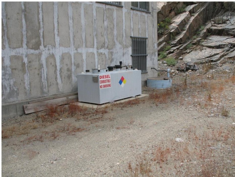
Figure 4.—Fuel storage tank for backup generator at Blue Mesa Powerplant, Colorado. The tank is located in a low area, which serves as secondary containment, away from any direct path to open water.
