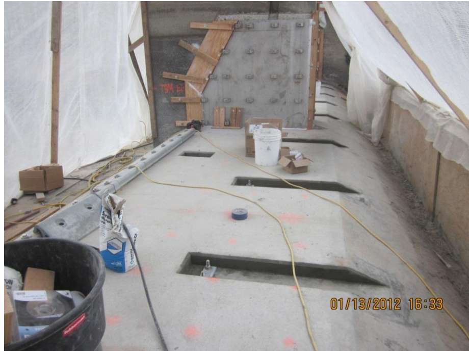
Figure 6.—New crest in place and stainless steel abutment plate being grouted in at rear of photo.
