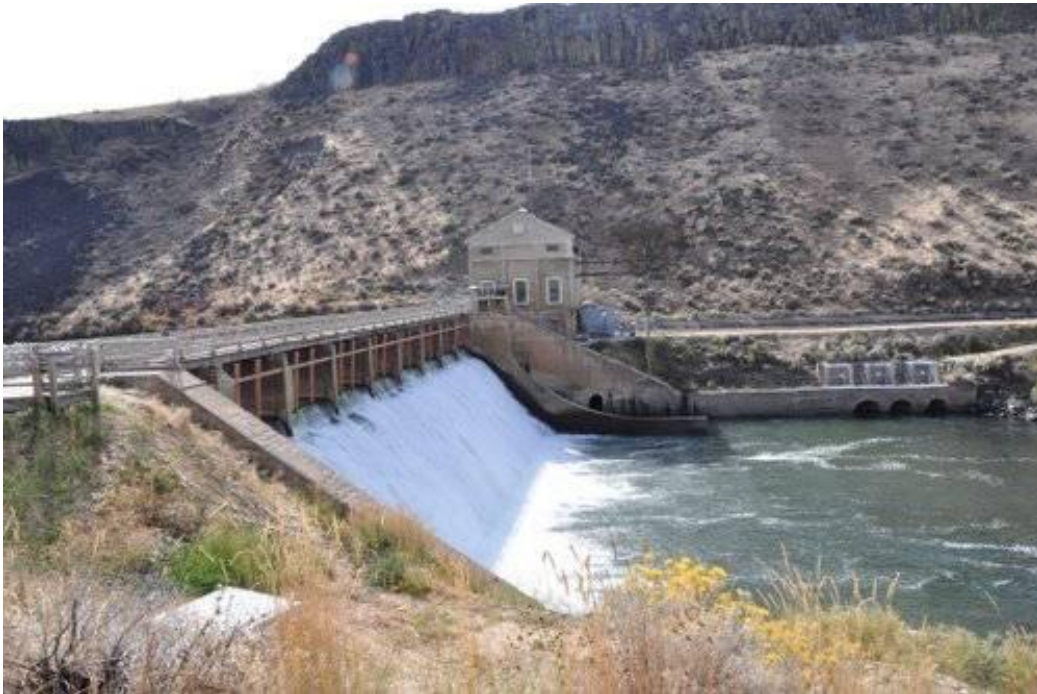
Figure 1.—Boise River Diversion Dam prior to installation of the pneumatic gates, showing the spillway and power house. New York Canal can be seen in the background.
