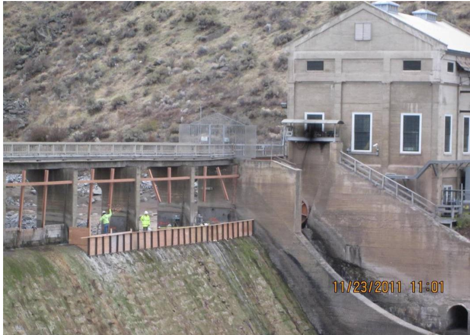
Figure 2.—Boise River Diversion Dam during the Obermeyer gate installation. Wooden safety rail has been placed at the worksite. Workers are removing original steel flashboard guides where the gates will be placed. Installed flashboards can be seen at far left.
