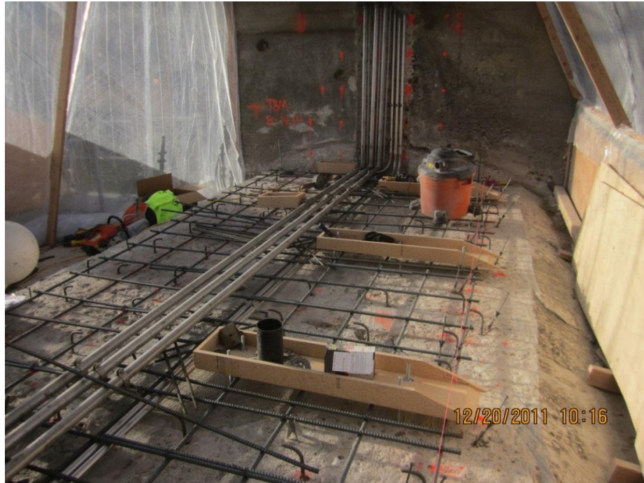
Figure 4.—Pre-placement of concrete crest, showing re-bar, stainless steel air lines, and forming slots for bladder restraining straps.
