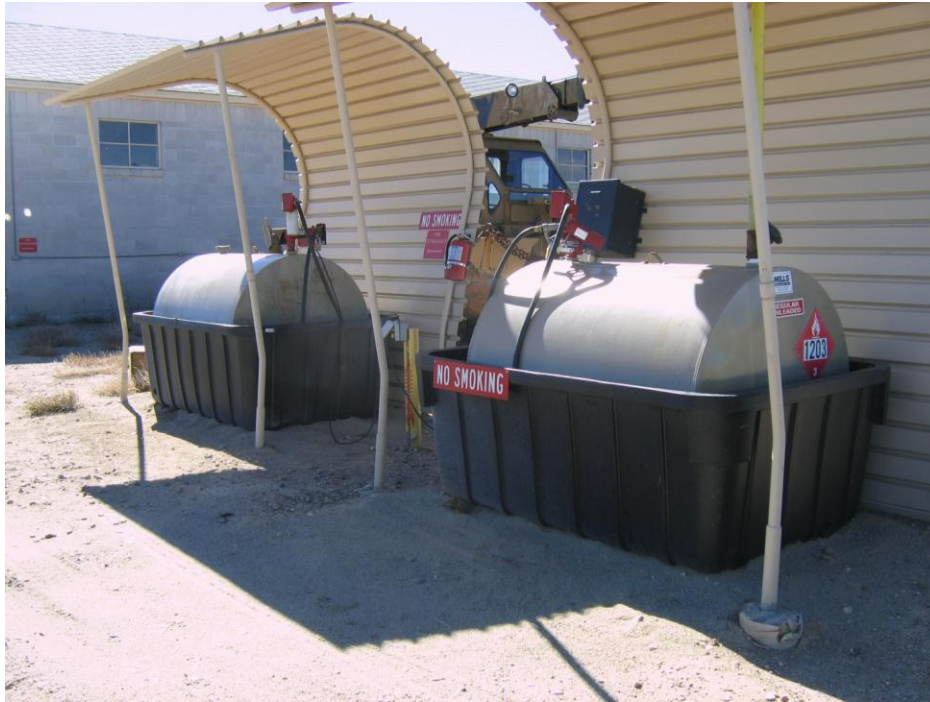
Figure 5.—Fuel storage tanks at Fontenelle Powerplant, Wyoming. The tanks are located away from any channels leading to water, and secondary containment is provided by the containment bins in which the tanks are placed.
