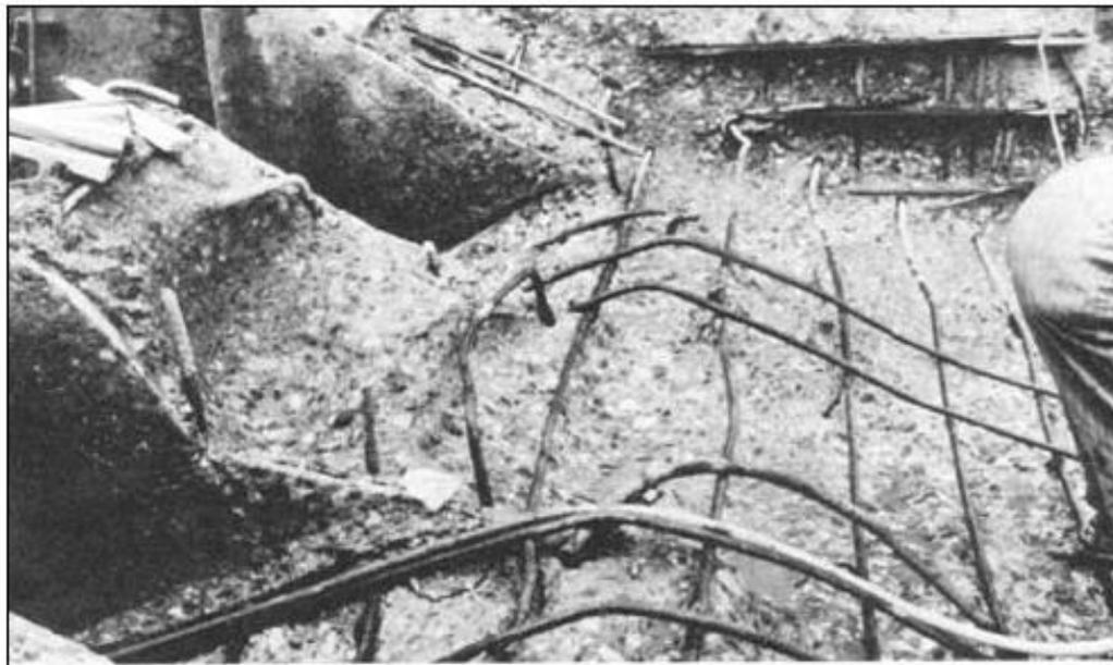
**Figure 3.—Two types of concrete damage caused by waterflow: cavitation damage in upper photograph and abrasion damage from action of cobbles, etc., in water in lower photograph. Yellowtail Afterbay Dam, Montana. Photos C-8272-3NA and C-8272-23.**
