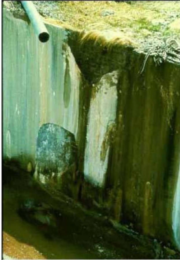
**Figure 2.—Freezing and thawing damage resulting from continuous moisture exposure.**
