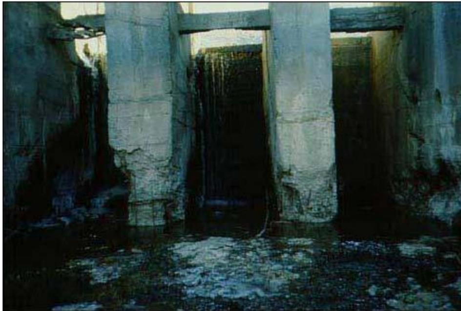
**Figure 1.—Lack of proper maintenance resulting in near loss of structure.**
