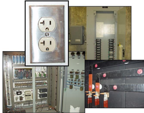
Some of the equipment where there is a potential arc flash hazard.
