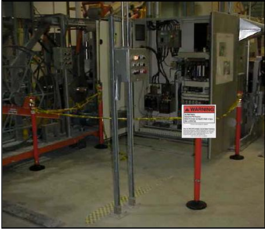
There are many different techniques used to alert workers of an arc flash boundary. The simplest technique is with caution tape as shown here.
