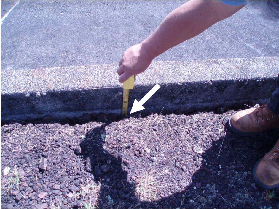
Photo 3.—Waikoloa Reservoir II Dam – Closeup view of the new typical earthquake-induced 1-inch wide, 20-foot-long separation between the reservoir concrete lining and the crest embankment material (arrow), shown in the previous photograph, evident at numerous locations and of various lengths on the crest.
