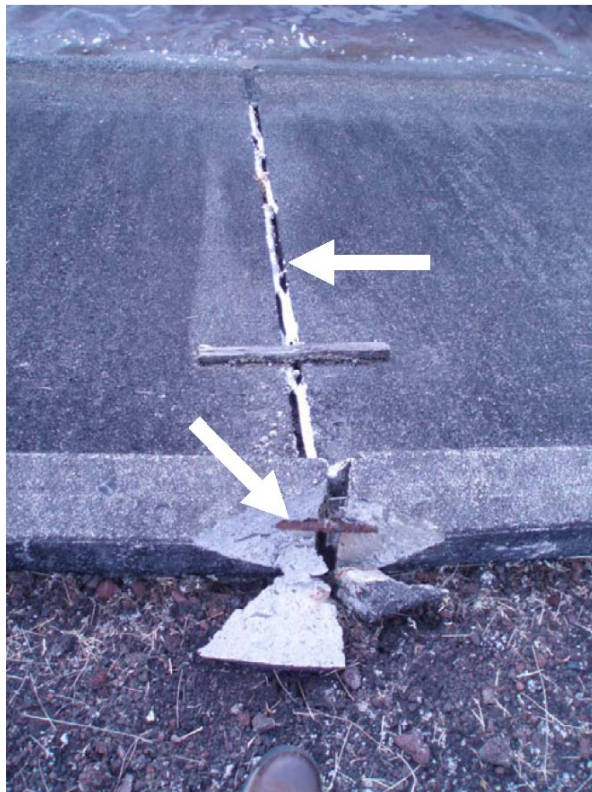
Photo 3.—Waikoloa Reservoir II Dam – Closeup view of the new typical earthquake-induced 1-inch wide, 20-foot-long separation between the reservoir concrete lining and the crest embankment material (arrow), shown in the previous photograph, evident at numerous locations and of various lengths on the crest.
