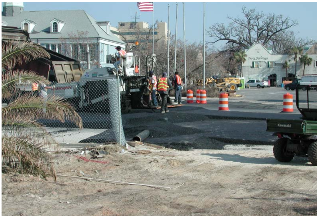
Figure 5.—Mississippi Department of Transportation building a ramp over the distribution line.
