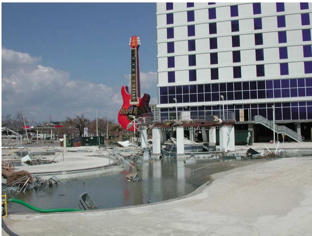
Figure 2.—Hard Rock Casino pool area – operations site.
