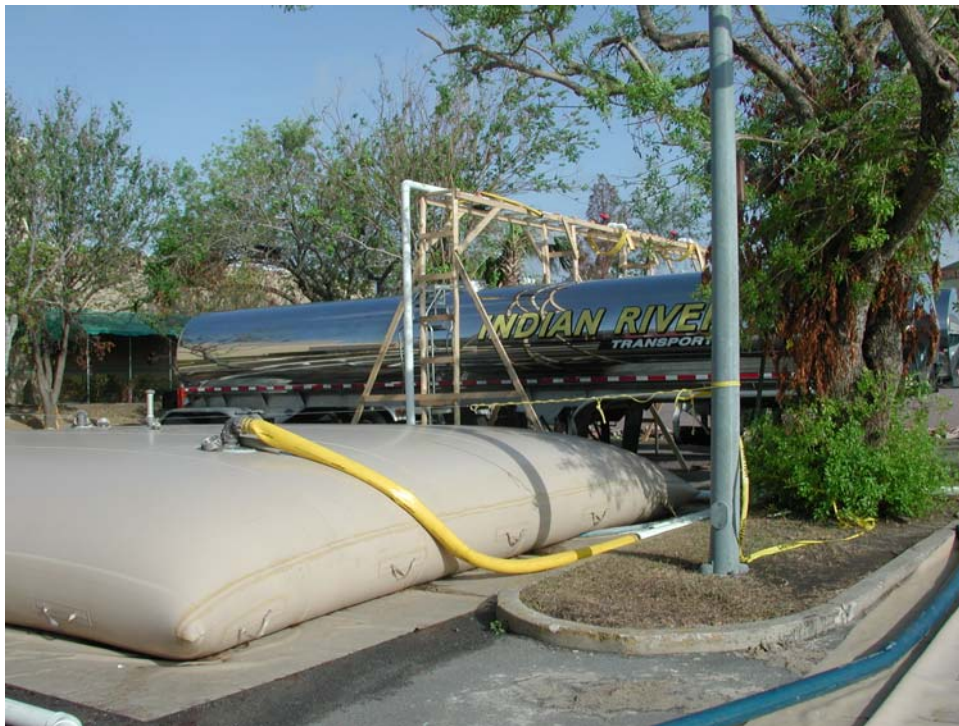
Figure 7.—Additional storage at the hospital – 3 6-kgal trucks and another 20-kgal bladder.
