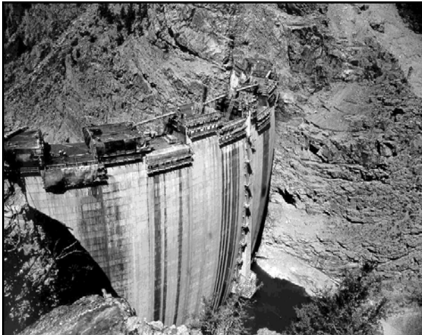
Figure 6.—Upstream face of Morrow Point Dam during construction.
