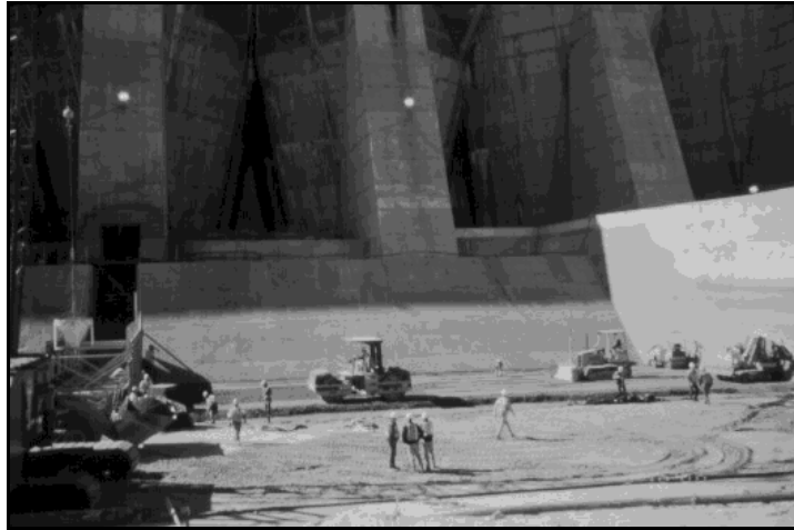
Figure 7.—RCC placement at Pueblo Dam.
