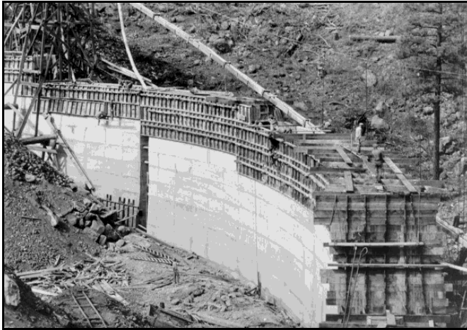
Figure 3.—Gerber Dam under construction.
