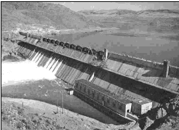
Figure 5.—Grand Coulee Dam under construction.
