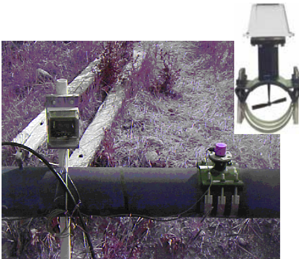
Figure 8.—GF+Signet propeller meter and display installed on a 10-inch pipeline. These meters may be used on pipes from 6 to 30 inches.
