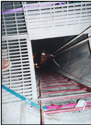
One victim, in a vertical shaft in a confined space, is placed in a SKED litter device and hoisted out of the shaft.
