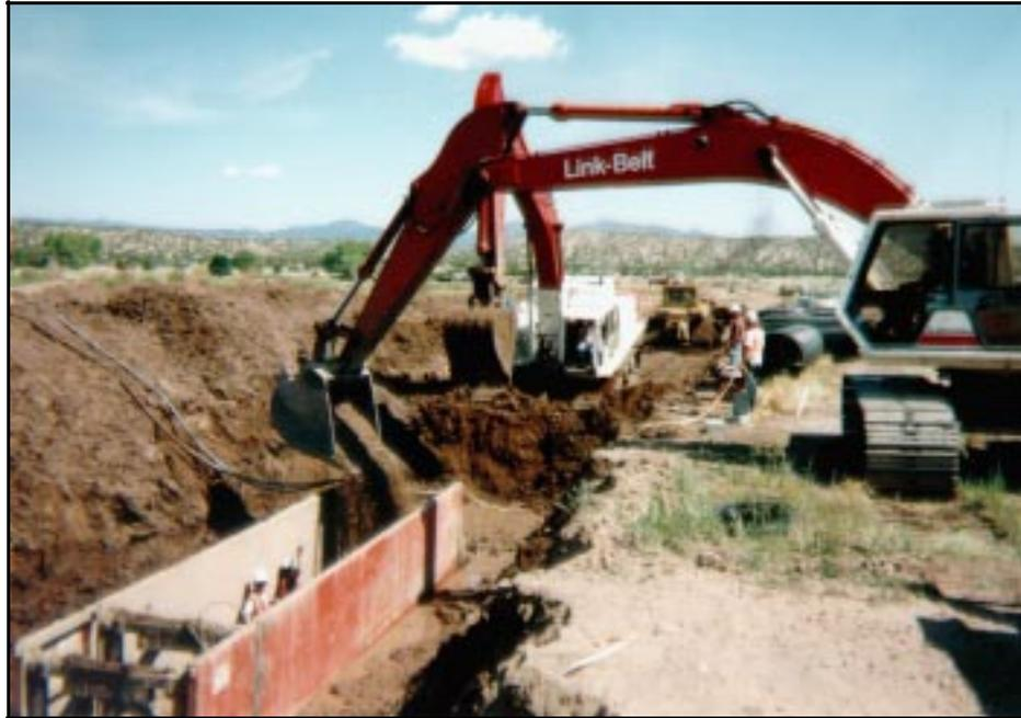
*Figure 6.—Open trench with box, envelope material controlled.*
