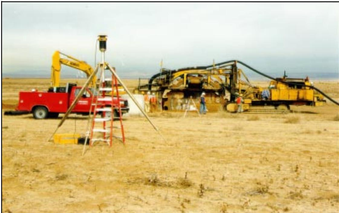
*Figure 12.—Laser plane system.*
