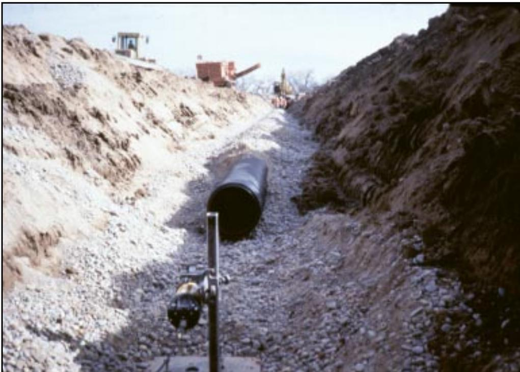
*Figure 2.—Pipe being covered with granular envelope material.*
