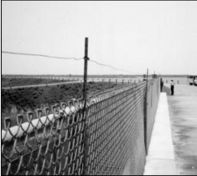
*Figure 1.—Wire barrier above fencing at Choke Canyon Dam.*
