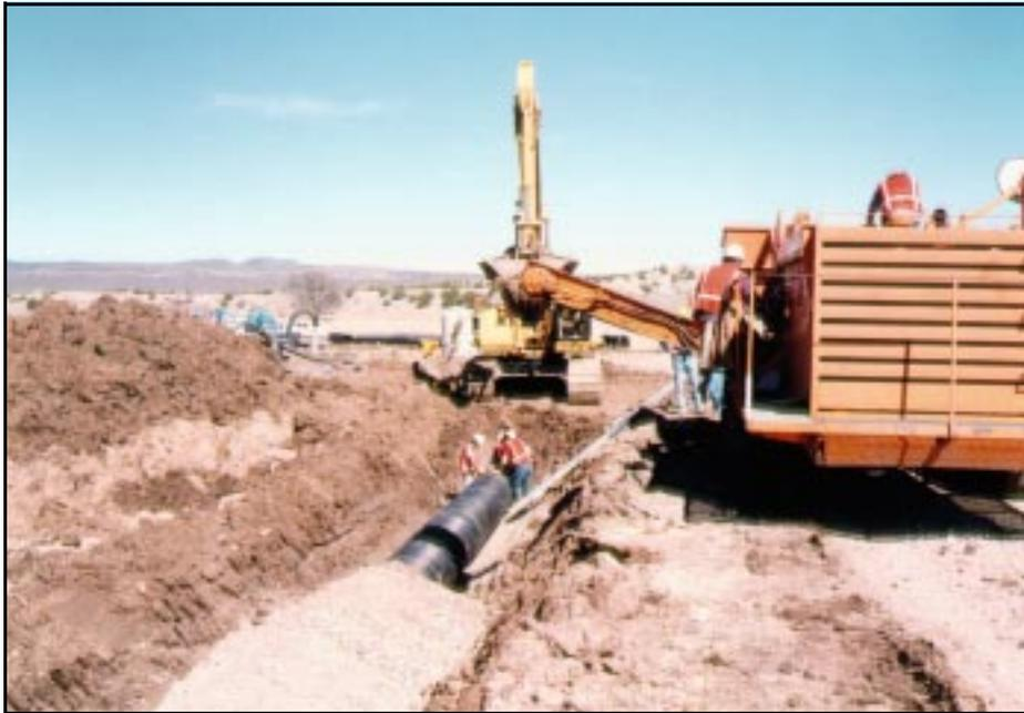
*Figure 5.—Open trench without box, gravel uncontrolled.*
