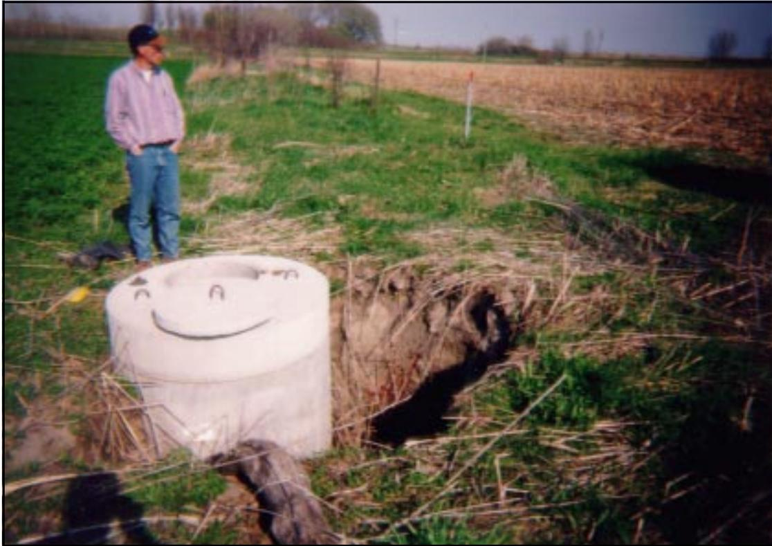
*Figure 13.—Sink hole at manhole caused by improper pipe connection.*
