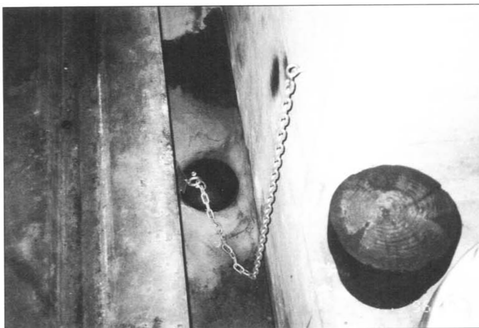
An innovative way to prevent oil spills.
