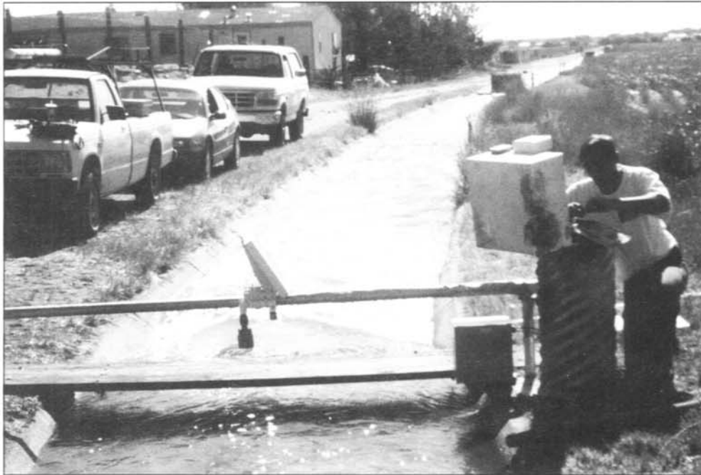
Figure 4.—Flume instrumentation including the transducer and temperature sensor, solar cell and battery, and the electronic flow meter mounted at site NT22.
