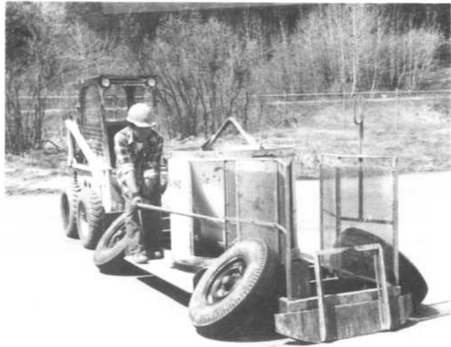
CN465-528-1114NA Blanco Tunnel, Chama Field Division, New Mexico. View of concrete bucket on the concrete cart used to repair the invert of Blanco Tunnel. Notice the man standing on the running board while operating the dump handle. The scree at the end of the cart helps spread the concrete when bolted in place.
