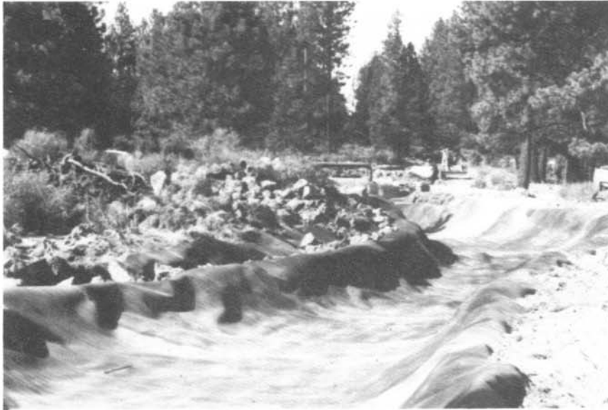
Figure 3.—Arnold Canal test sections 3 through 6. Installation of exposed geomembrane liner.
