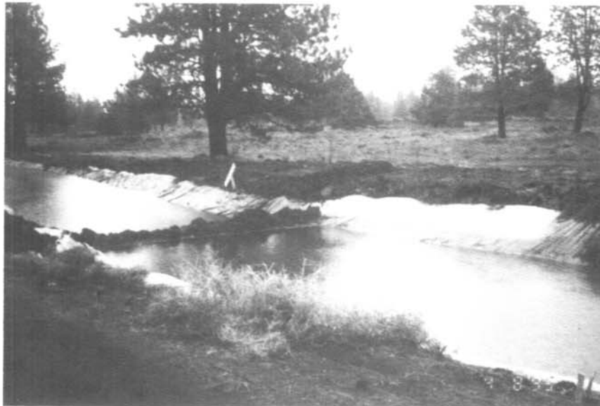
Figure 9.—Post-construction ponding tests.
