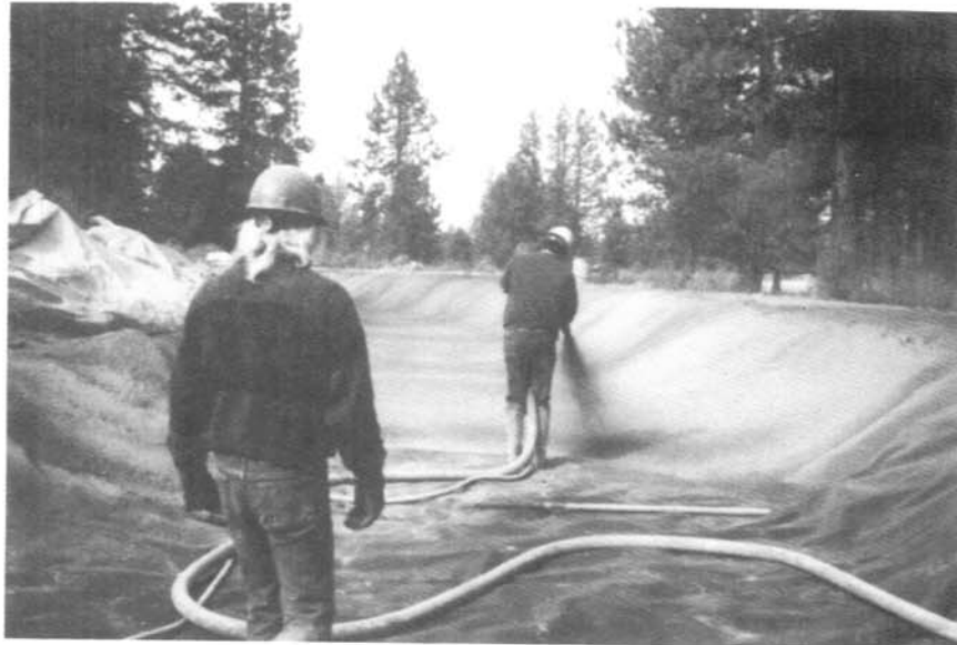
Figure 2.—Arnold Canal test sections 1 and 2. Application of shotcrete cover over geomembrane.
