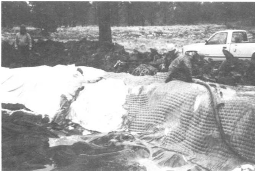
Figure 4.—Arnold Canal test sections 7 through 10. Installation of grout-filled mattress.
