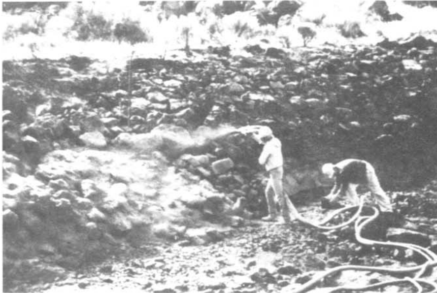
Figure 7.—North Unit Canal test sections 6 through 9. Application of 3-inch shotcrete lining.
