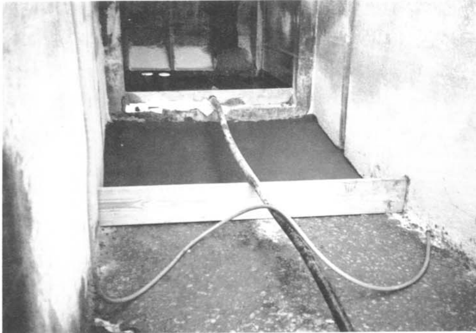
Concrete placement in downstream canal invert.
