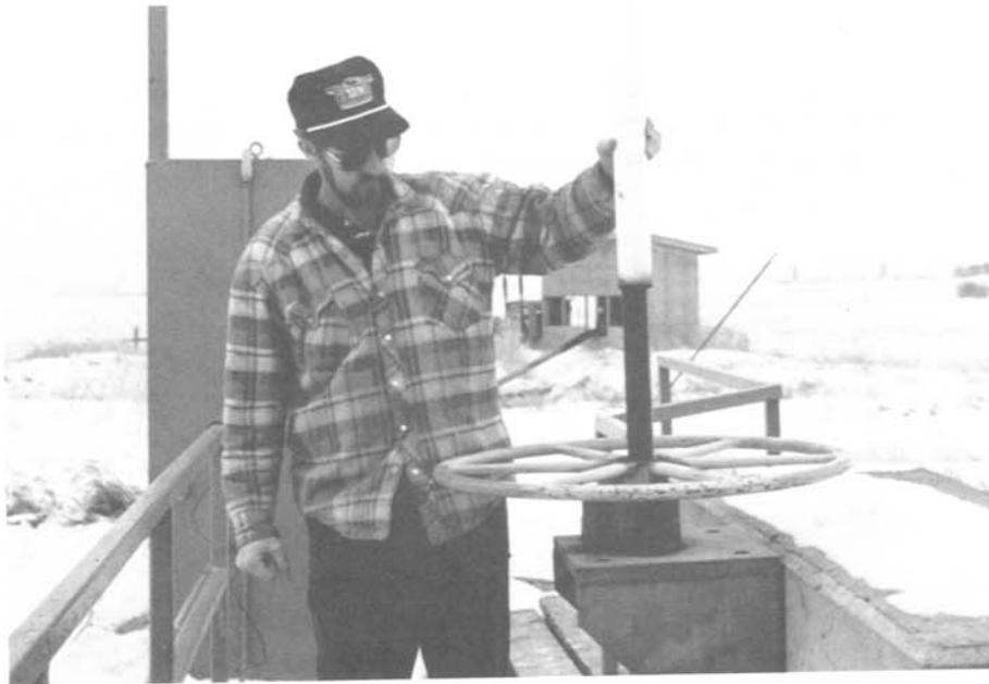
Ralph Oldenburger lifts gate stem cover from hand wheel gate.
