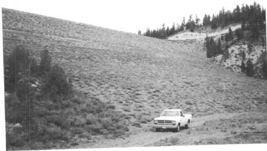
Figure 4. - Stampede Dam - Downstream face of dam showing minor vegetative growth. 5/10/90
