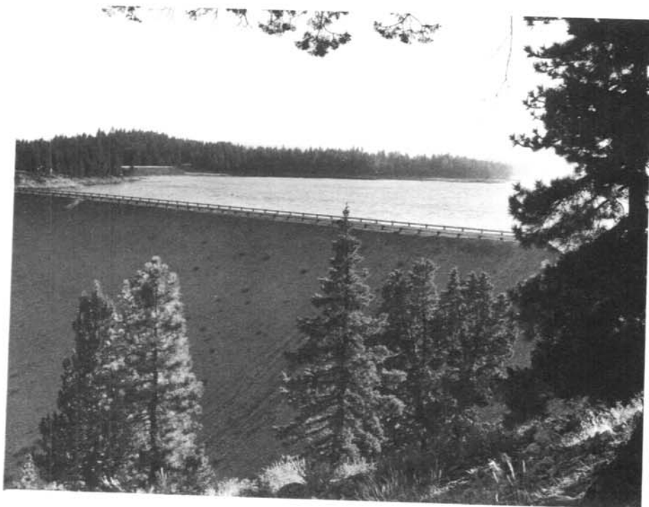
Figure 2. - Stampede Dam and Reservoir looking upstream from left abutment. 7/1/73
