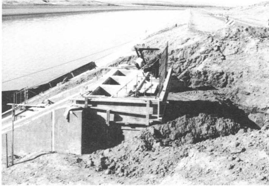
Figure 14. – Earth being graded in around turnout.
