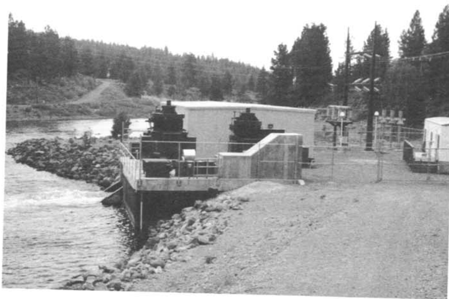
Figure 5. - Stampede Dam - Powerplant service yard. 5/10/90
