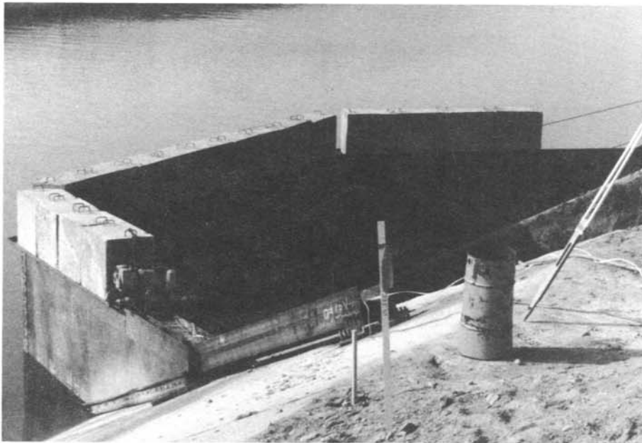
Figure 7. – Cofferdam in place (note concrete weights).
