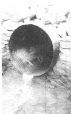
Figure 3. - Corrugated metal culvert after cleaning, showing patchy tar coating.
