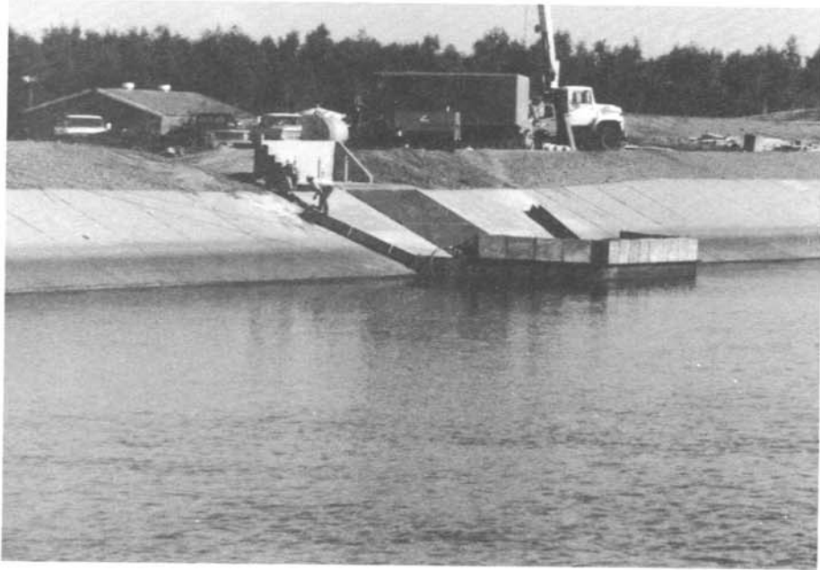
Figure 18. – Preparing to remove the cofferdam.
