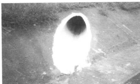
Figure 5. - Finished culvert outlet on bottom of downstream face of Enid Dam.
