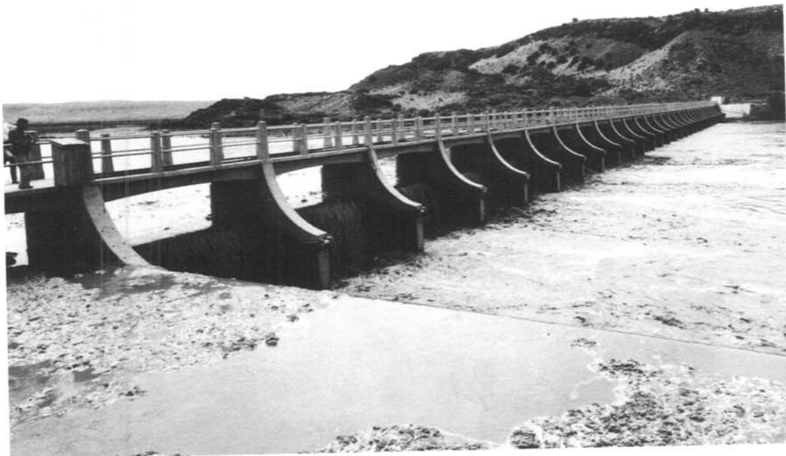
Figure 1. - Downstream view of San Acacia Diversion Dam from canal headworks. 6/30/66
