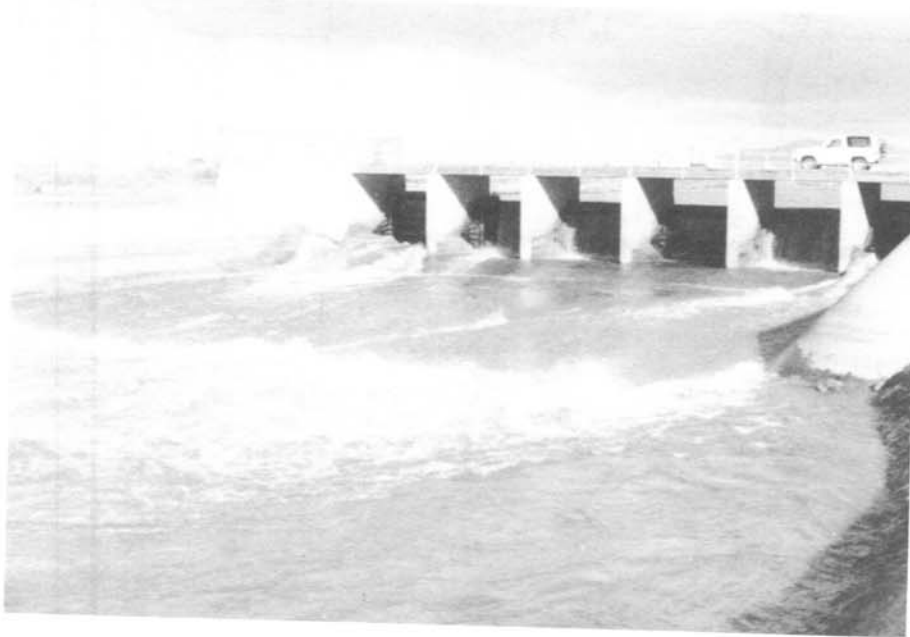
Photograph 1. - Riverside Diversion Dam. Sluiceway stilling basin. 3/17/87
