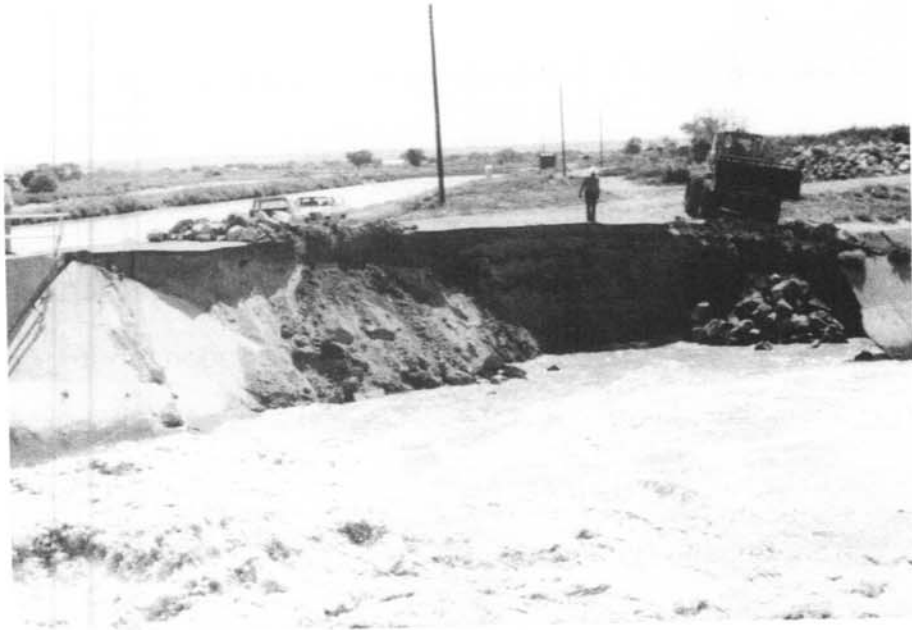
Photograph 2. - Riverside Diversion Dam. Left abutment of sluiceway stilling basin. 6/9/87
