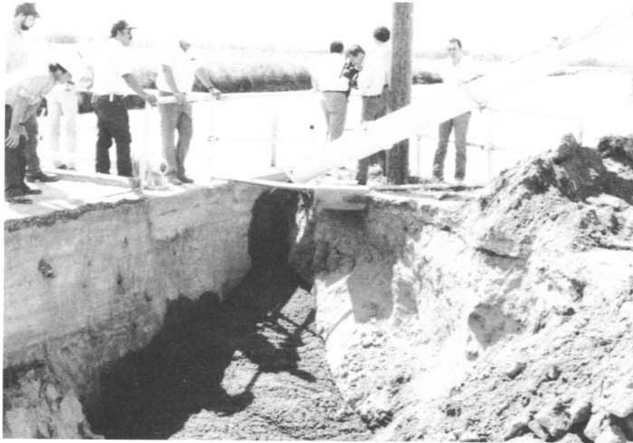
Photograph 5. - Riverside Diversion Dam. Filling sinkhole at left side of sluiceway. 6/9/87
