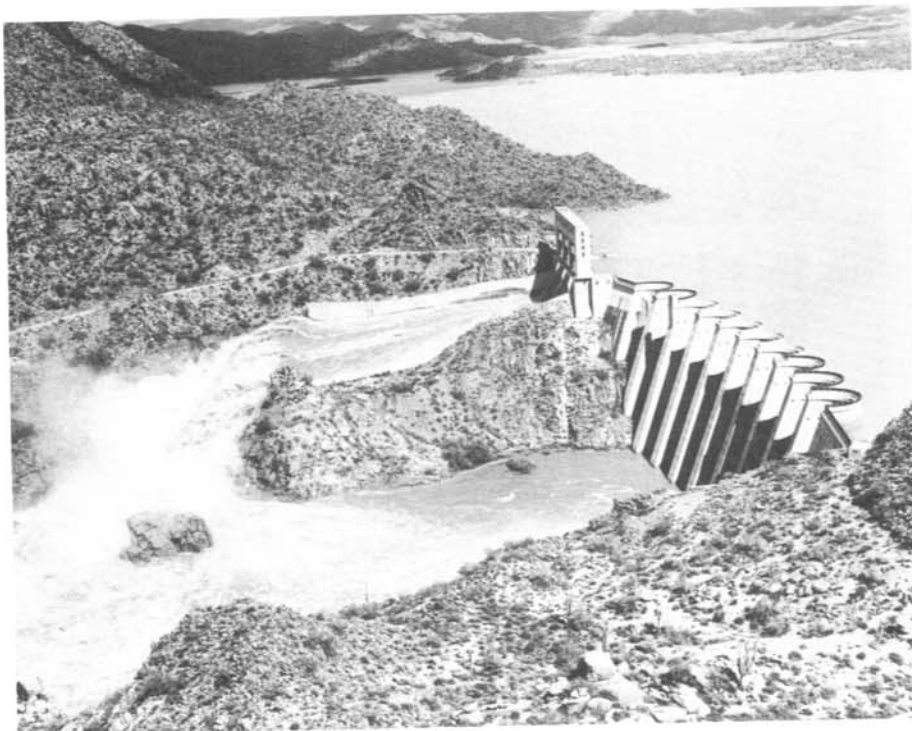
Figure 4. - Aerial view of Bartlett Dam showing approximately 70,000 ft 3 /s being released from the reservoir which was filled with recent heavy rains. 3/3/78
