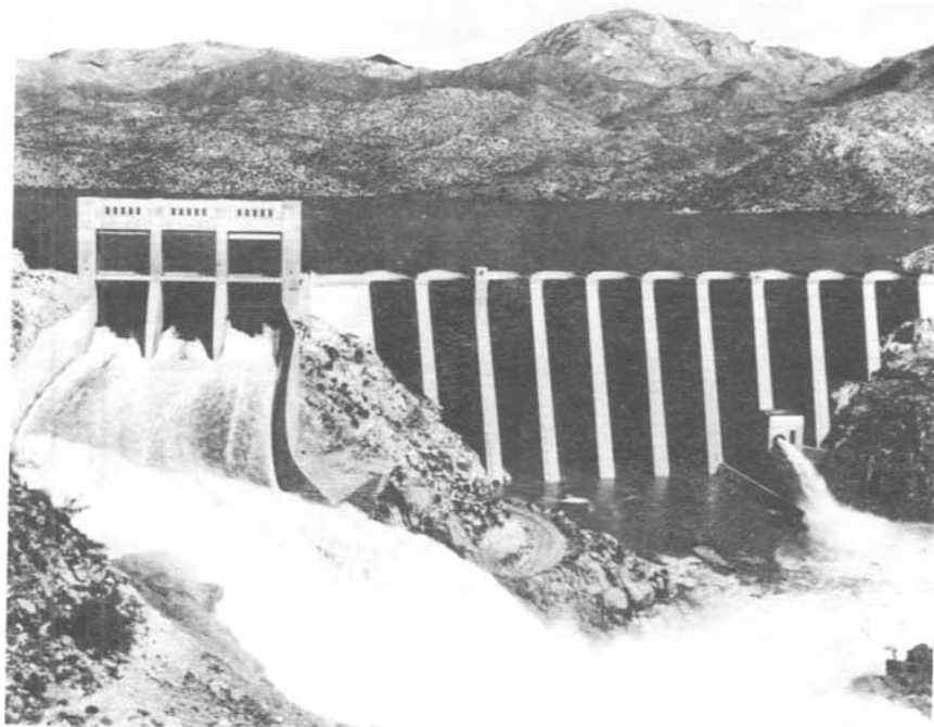
Figure 2. - Bartlett Dam showing reservoir full with a flow through the spillway of approximately 14,000 ft 3 /s. 4/15/41
