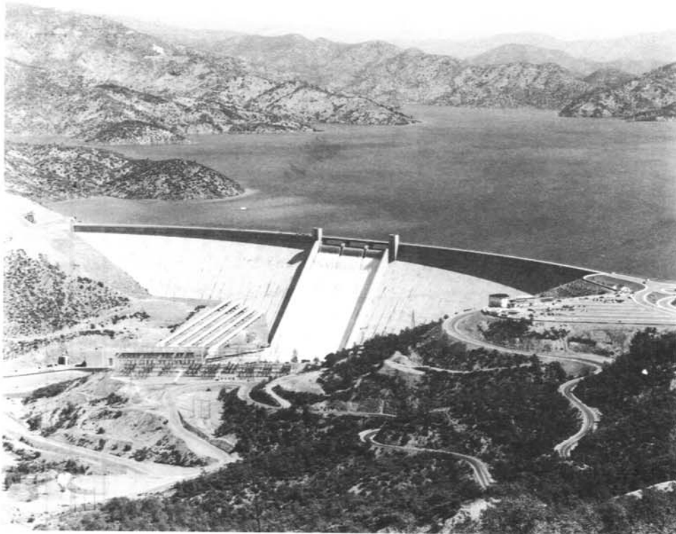
Photo 2. - Aerial view of Shasta Dam showing spillway gates operating — 7/18/51
