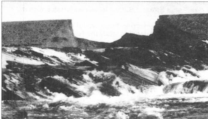
Earthfill dike that burst had history of leakage ever since its reservoir was first filled in 1985.
