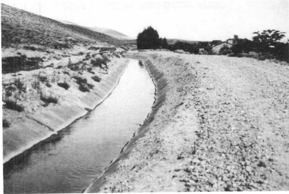
Completed Project, Badger East Lateral
