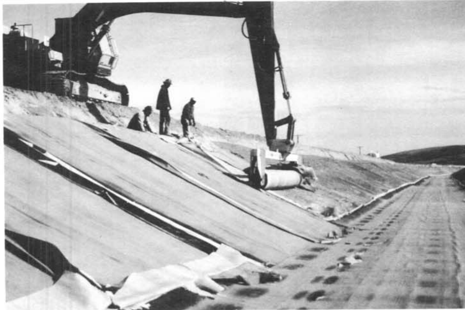
Placement of liner
