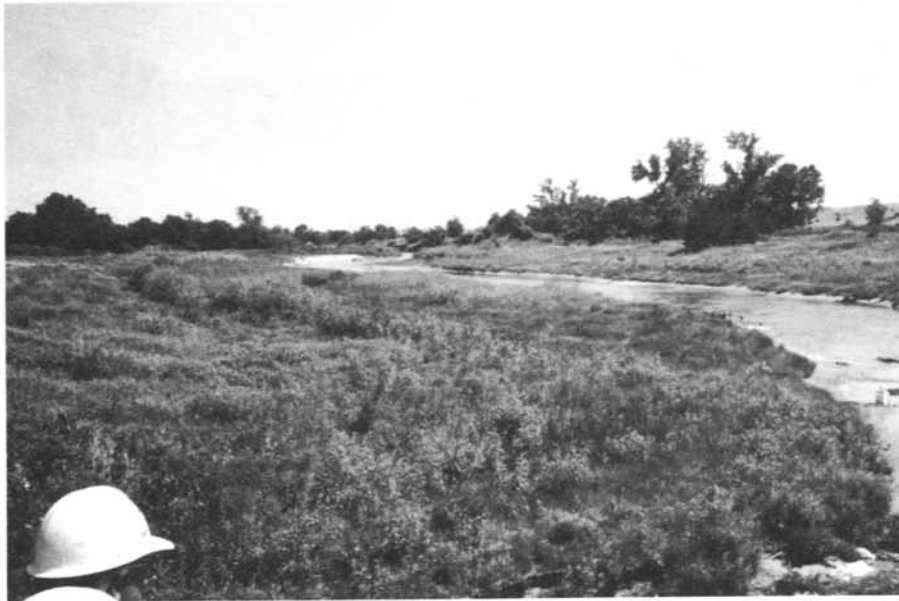
Calamus Dam – Calamus River downstream of river drop structure. 6/7/88
