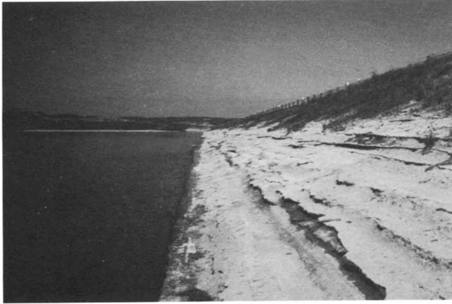
Calamus Dam – Soil-cement protection on upstream face of dam. 6/7/88
