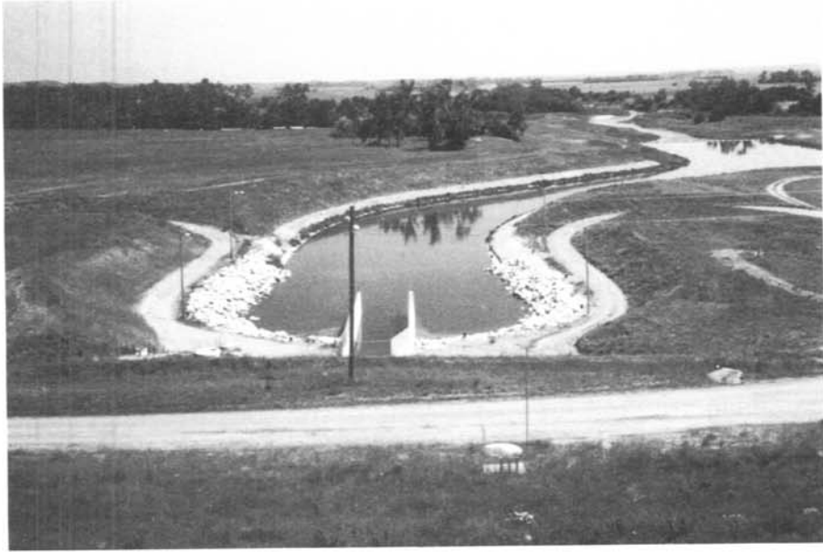
Calamus Dam - Spillway discharge channel. 6/7/88
