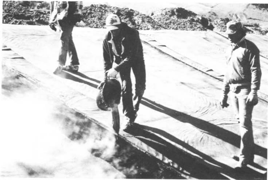
Joint sealing
