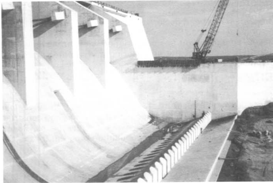
Figure 1. - Brantley Dam - Spillway chute and stilling basin. 10/4/87
