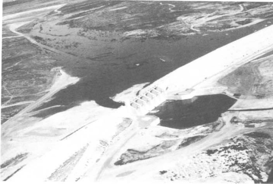
Figure 5. - Brantley Dam - Aerial view of concrete structure, stilling basin, left and right abutments, and Reservoir. 9/7/88
