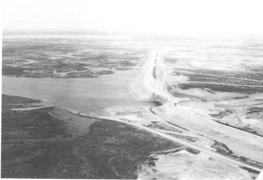
Figure 6. - Brantley Dam - Aerial view showing Dam and Reservoir. Lake McMillan can be seen in the background. Note curve of the earthen abutments. 9/29/88
