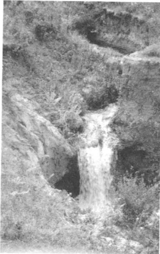
Figure 1. - Erosion occurring prior to installation of the rock drops.
