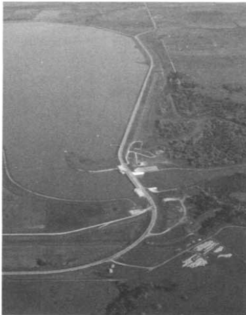
Cover photograph: Palmetto Bend Dam, Texas
