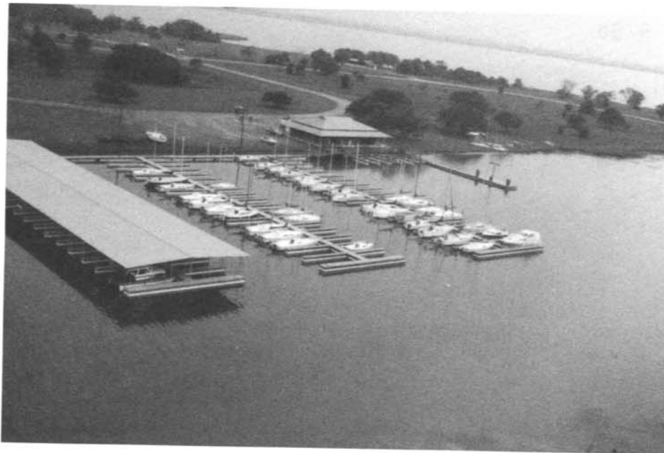
Photo 6. - Palmetto Bend Dam, Texas. Aerial view of the marina. 9/7/84
