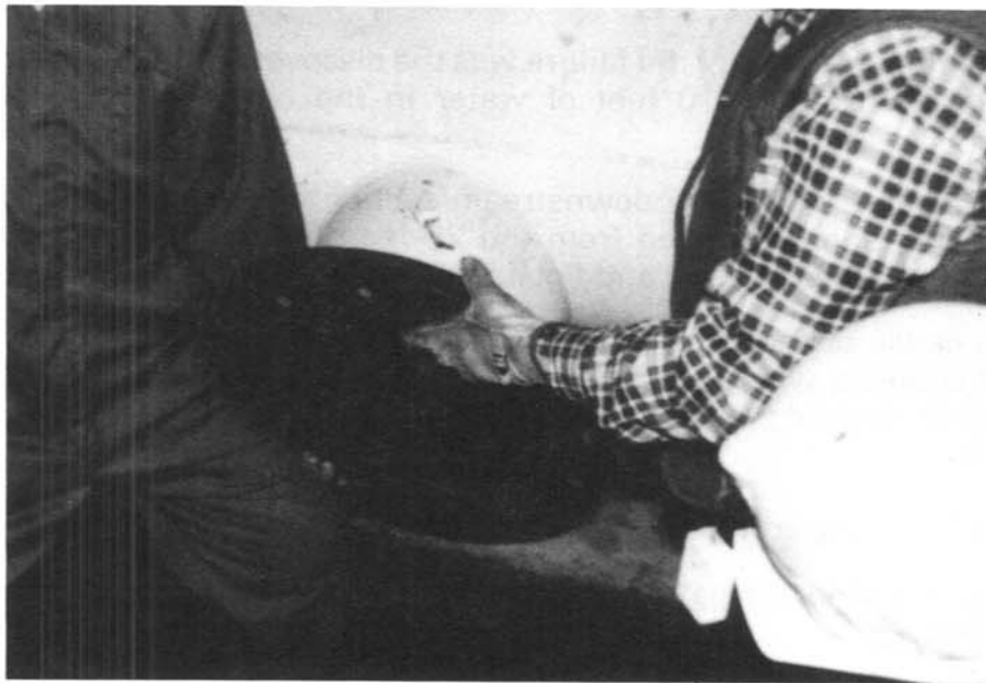
Currant Creek Dam. - Class E-type flange which replaced sleeve-type couplings. 4/9/85
