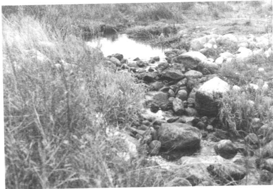
Figure 2. - Rock drop in Drain No. 64 Hays has stopped erosion - excellent regrowth of vegetation occurring.
