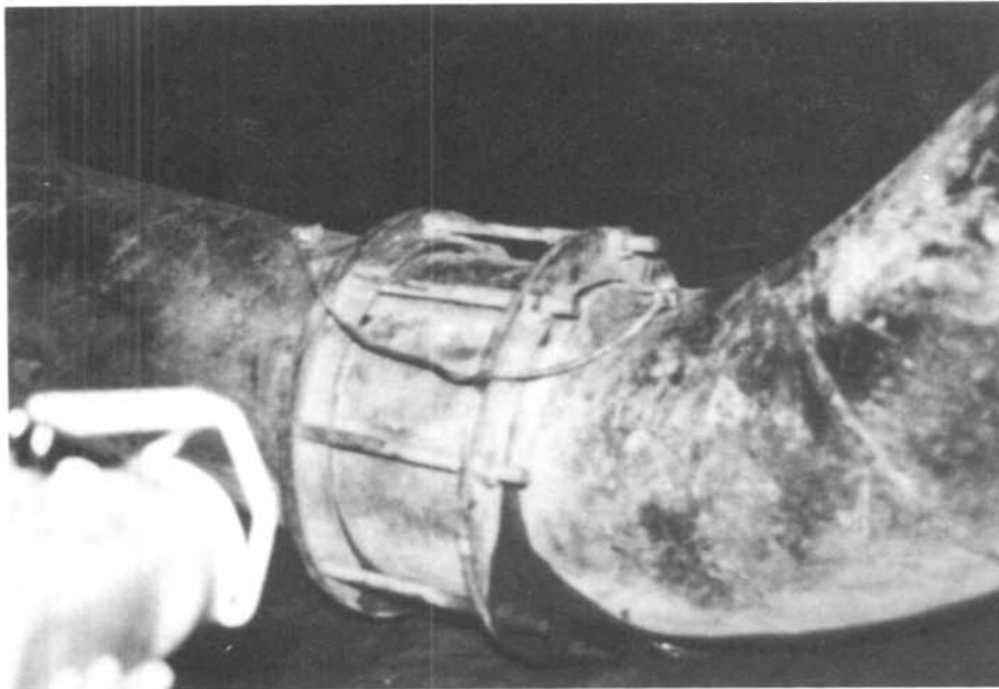
Currant Creek Dam. - Example of dresser-style coupling unsupported for thrust load. 4/9/85
