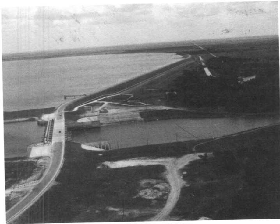
Photo 3. - Palmetto Bend Dam, Texas. Aerial view of spillway, river outlet works, pipeline, and east and west parking lots. 9/86
