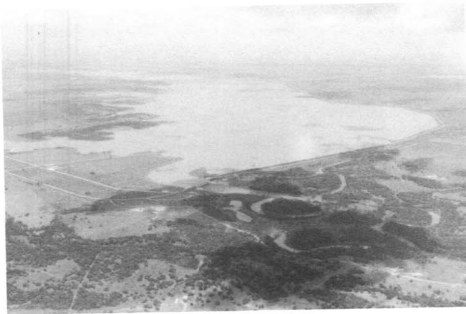
Photo 4. - Palmetto Bend Dam, Texas. Aerial view of Dam and Lake Texana. 5/12/84
