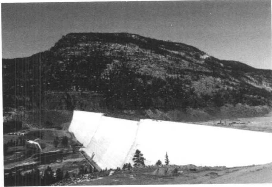
Aerial view of Upper Stillwater Dam. 11/23/87
