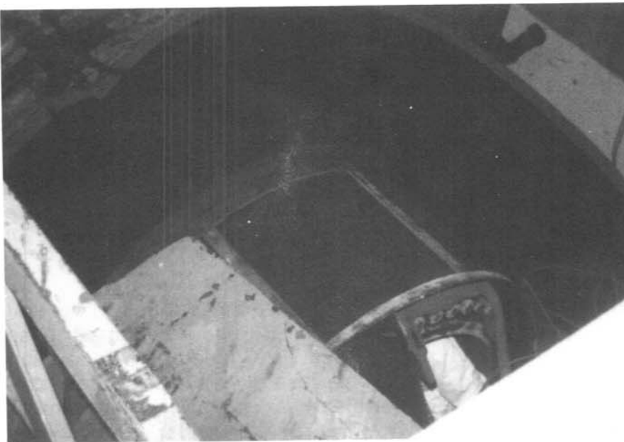
Photo 2. - Bartlett Dam, Arizona
