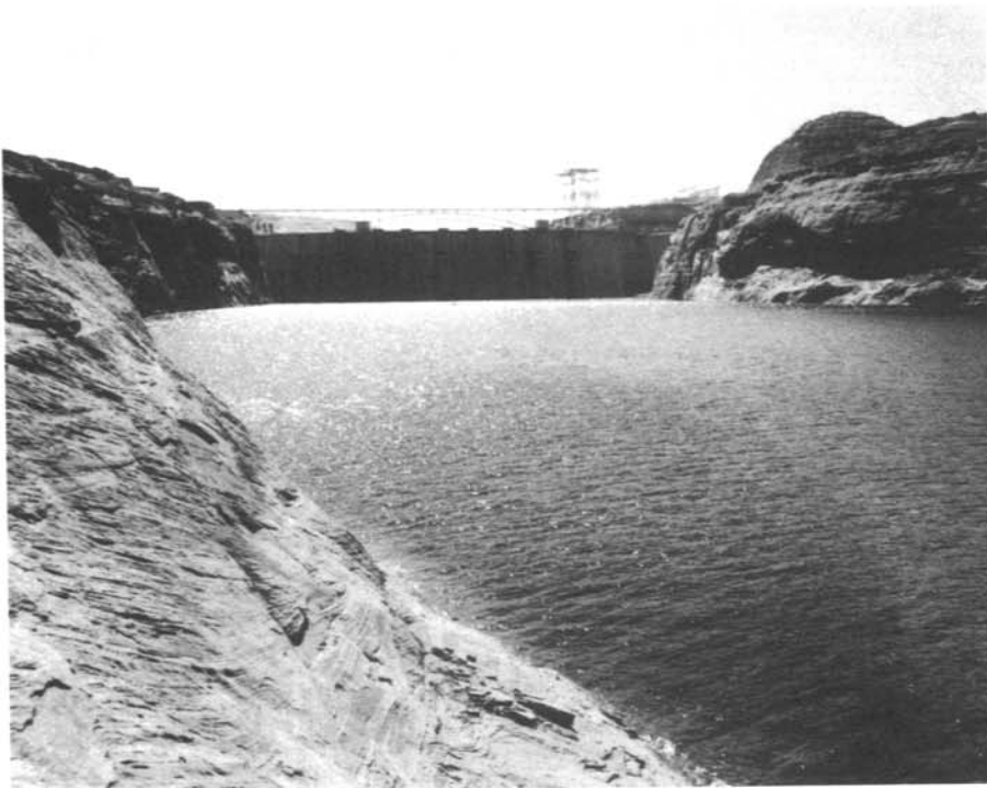
Photo 6. Glen Canyon Dam.
