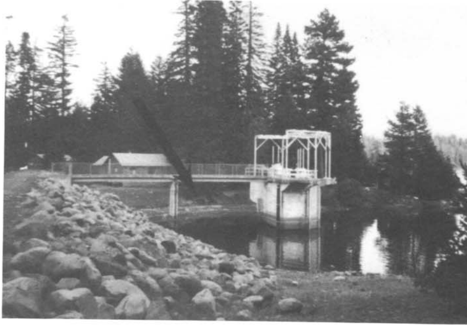
Photo 7. - The soil around the root system of the mature conifer (arrow) has been eroded by fluctuating reservoir levels and wave action. This conifer needs to be removed because it can fall and destroy the access bridge or equipment on the intake tower.
