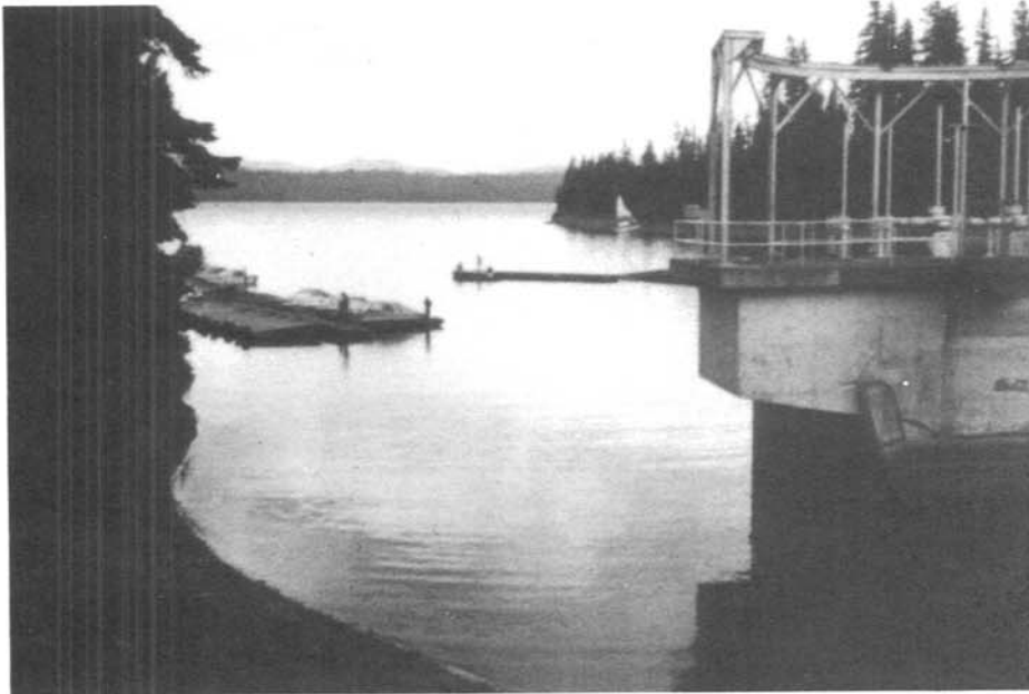
Photo 2. Potentially hazardous intake tower. A safety buoy line should be installed to prevent swimmers and boaters from drifting into intake tower. A sign should also be posted warning recreationists of high-velocity flows.
