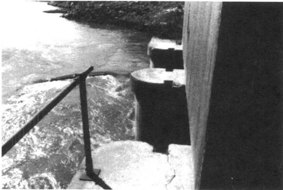
Photo 4. - Closeup view of above photo showing opening.
