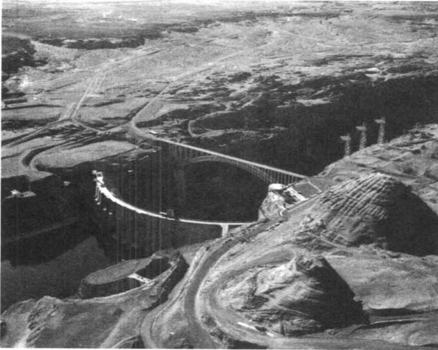
Photo 3. Glen Canyon Dam.
