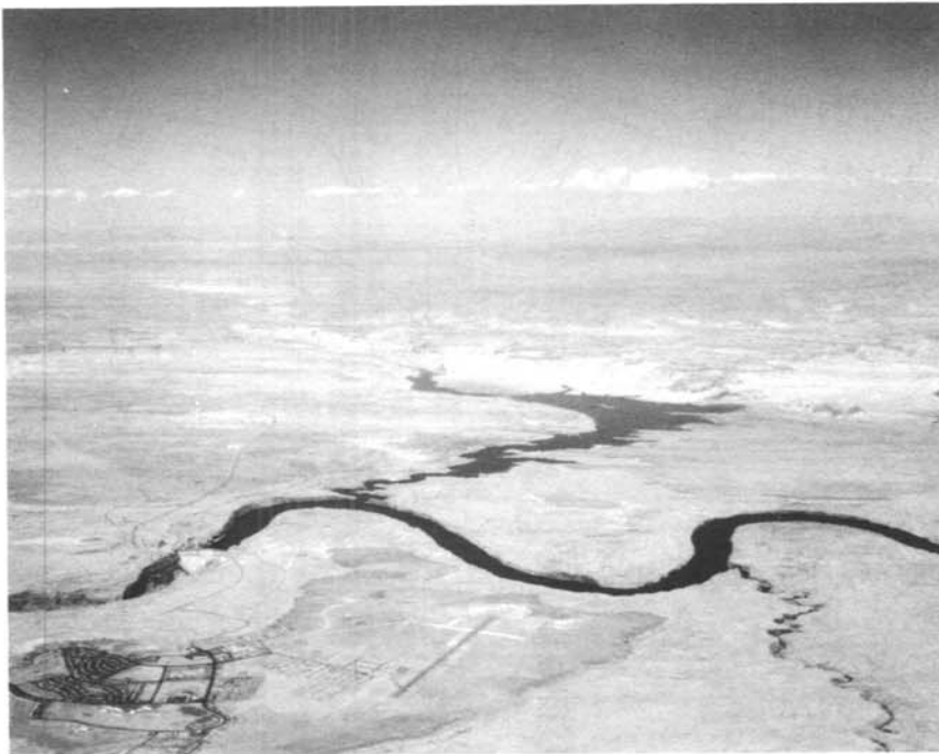
Photo 2. Glen Canyon Dam.
