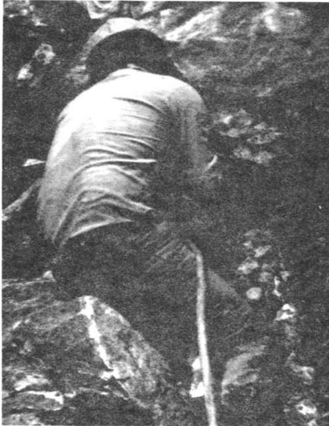
Figure 6. – Shear zones were removed with a hand-held air spade.
