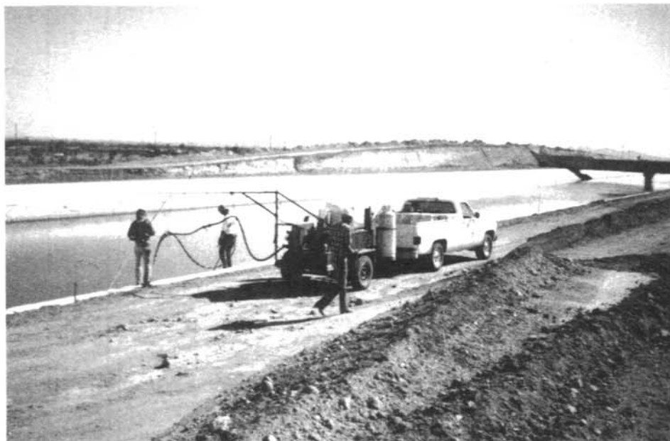
Figure 7. – Contractor seals contraction joints with hot-applied sealant on California Aqueduct.
