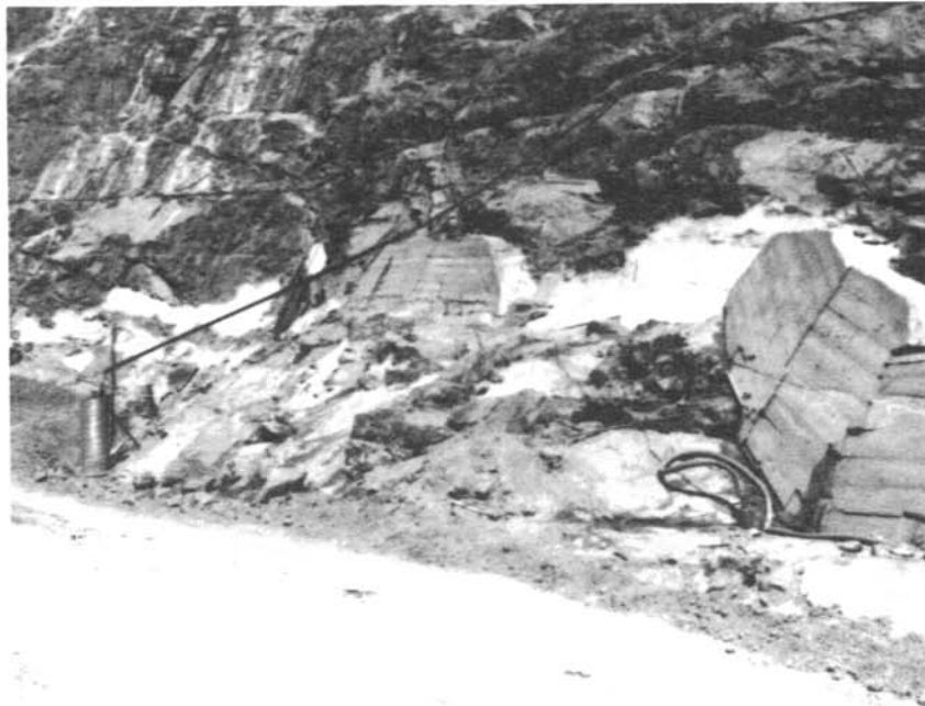
Figure 5. - Overhangs were backfilled by installing bulkheads and filling with conventional concrete.
