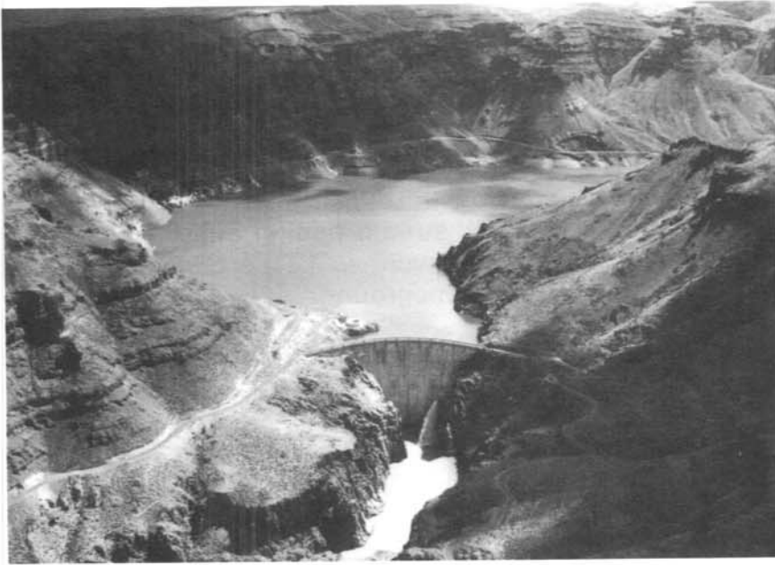
Photo 1. Aerial view of Owyhee Dam and reservoir looking upstream. "Glory hole" spillway stands dry above the waterline.
