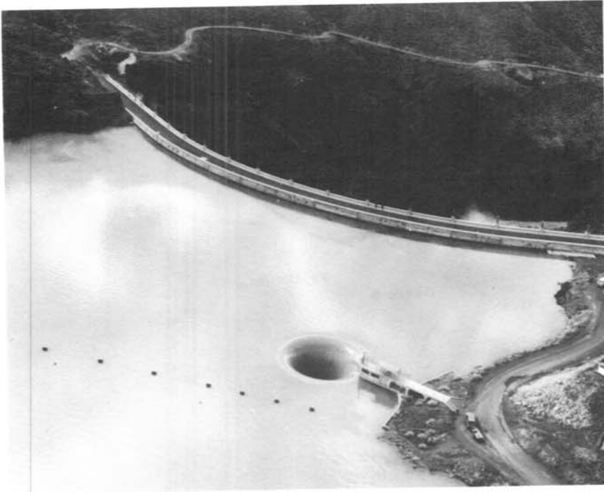
Photo 3. Aerial view of Owyhee Dam and reservoir showing the high water level following heavy spring rains. Note "glory hole" spillway in foreground.
