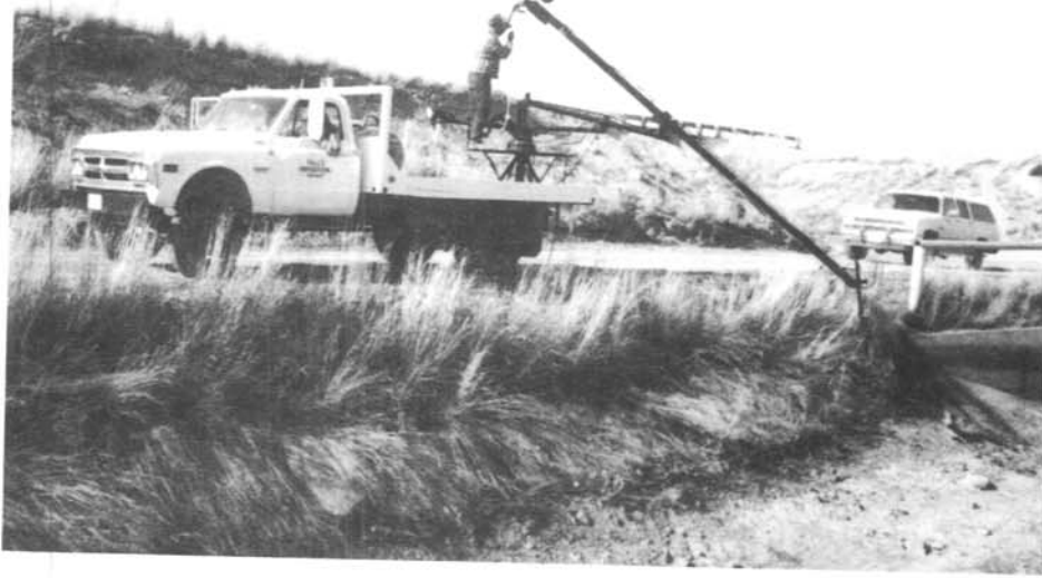
Photo 1. Weedburner mounted on truck and being used in ditch alongside of road.
