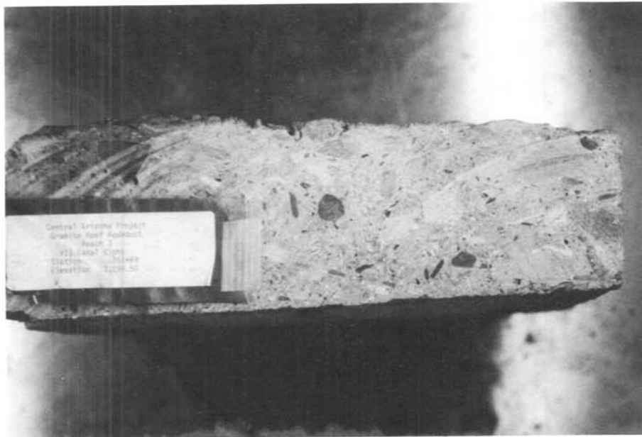
Figure 2. Side view of Sample No. 11. This edge shows generally satisfactory consolidation.
