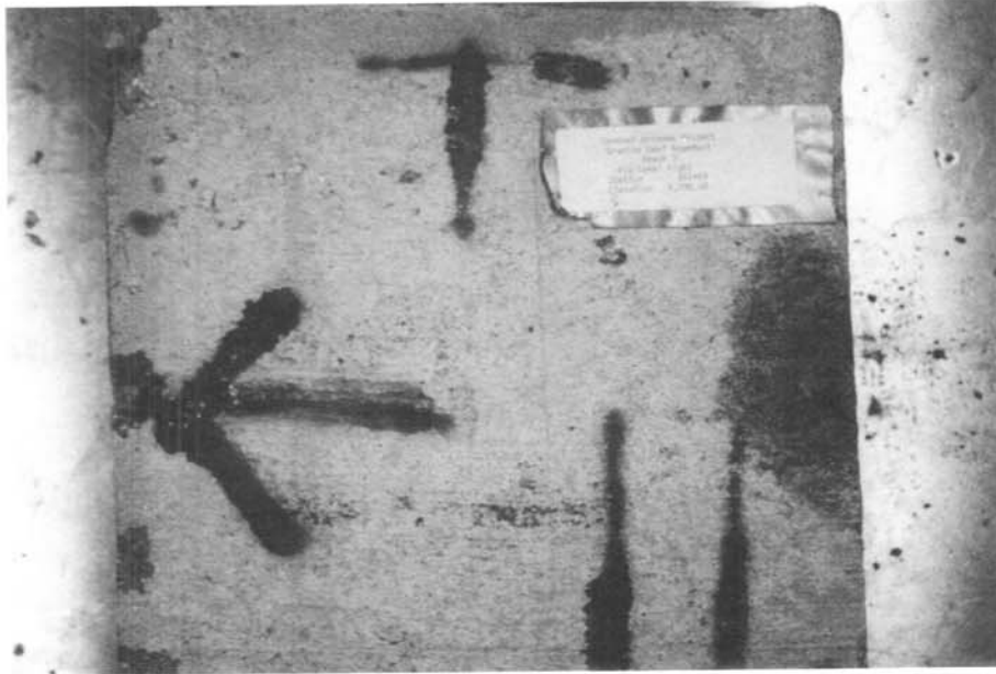
Figure 1. Upper surface of Sample No. 11. Consolidation of the concrete on the exposed surfaces was generally satisfactory.
